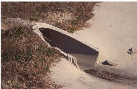
Use **Beveling of Pipe End** (719-610-00) when specified in the plans or special provisions. Beveled ends may only be used on flexible pipe up to 24" diameter and on rigid pipe up to 60" diameter. When beveling of pipe ends is specified on flexible pipe larger than 24" diameter, install pipe straight headwall, pipe end structure, flared end section, or wingwall section. Use factory fabricated beveled ends for all pipe types unless approved by the Engineer.
