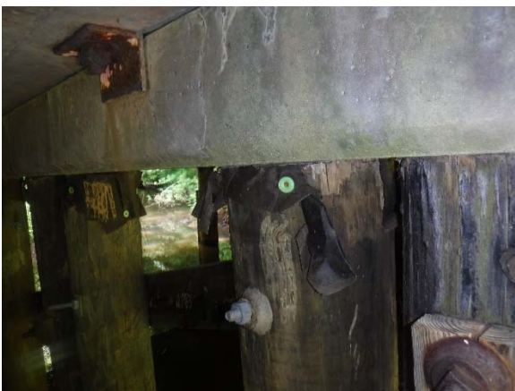
Photo 5. Timber Pile Cap Felt
