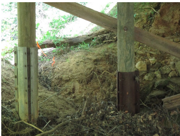
Photo 5. Metal Sleeve's on Timber Piles.
