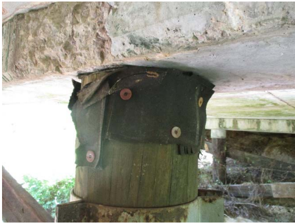
Photo 3. Timber Pile Felt Material
