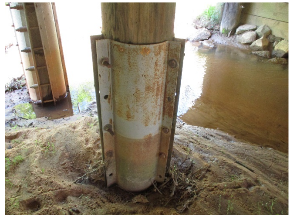
Photo 4. Metal Sleeve on Timber Pile.
