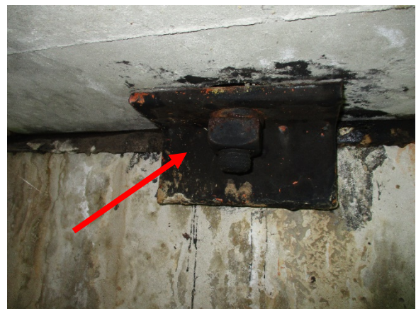
Photo 6. L-Bracket is Positive for Lead.
