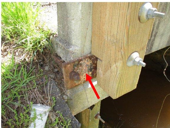
Photo 5. Tie-rod Washer Is Positive for Lead.
