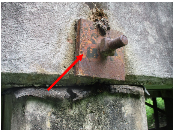
Photo 5. Tie-rod Washer is Positive for Lead.
