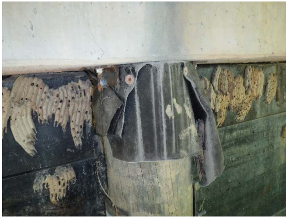
Photo 3. Timber Pile Felt Material
