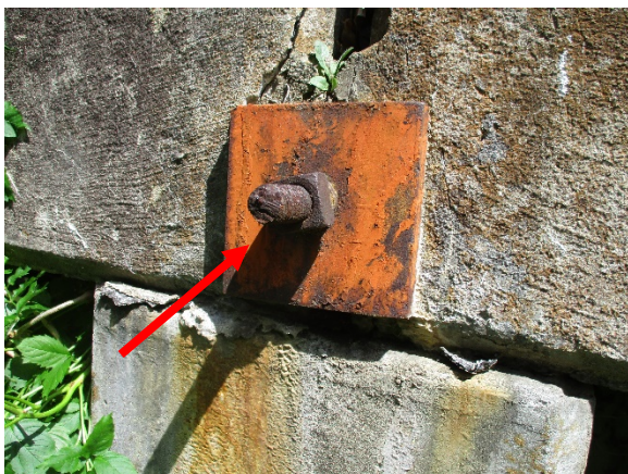
Photo 5. Orange Tie-rod Washer is Positive for Lead.
