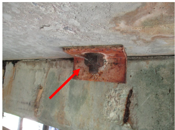
Photo 6. L-Bracket is Positive for Lead.
