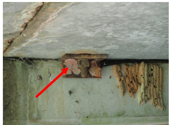
Photo 6. Orange L-Bracket is Positive for Lead.
