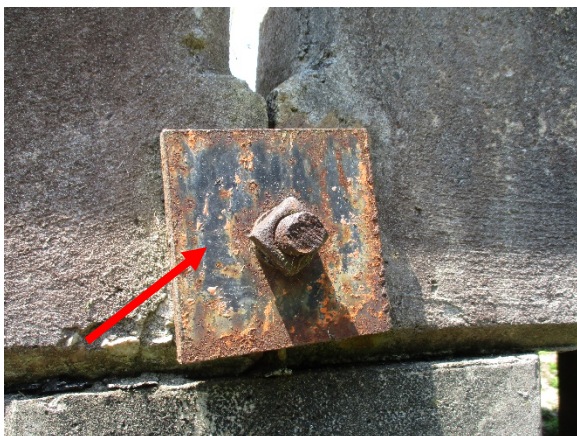
Photo 5. Tie-rod Washer is positive for Lead.
