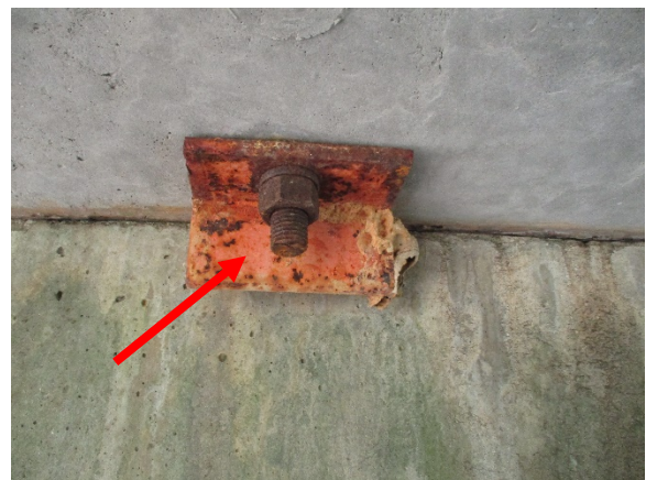
Photo 6. L-Bracket is Positive for Lead.
