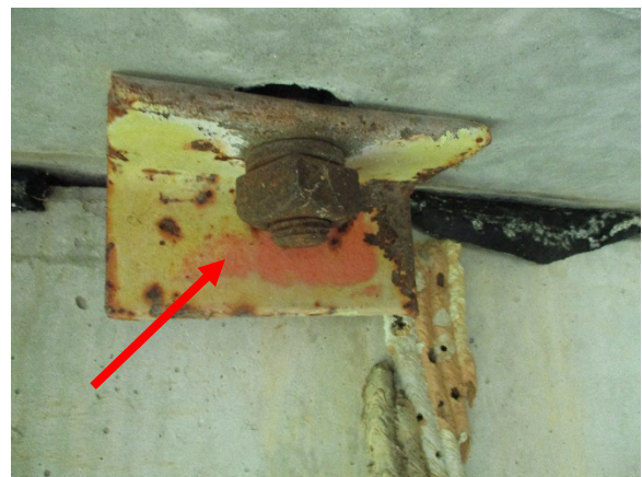
Photo 6. Orange L-Bracket is Positive for Lead.
