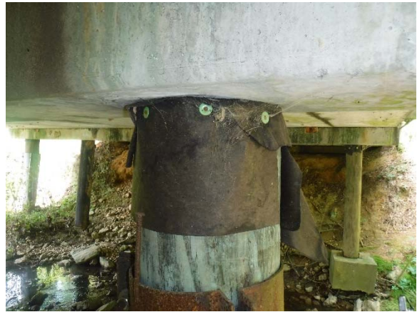
Photo 4. Timber Pile Cap felt.
