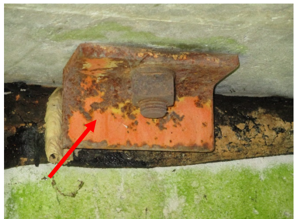
Photo 6. L-Bracket is Positive for Lead.
