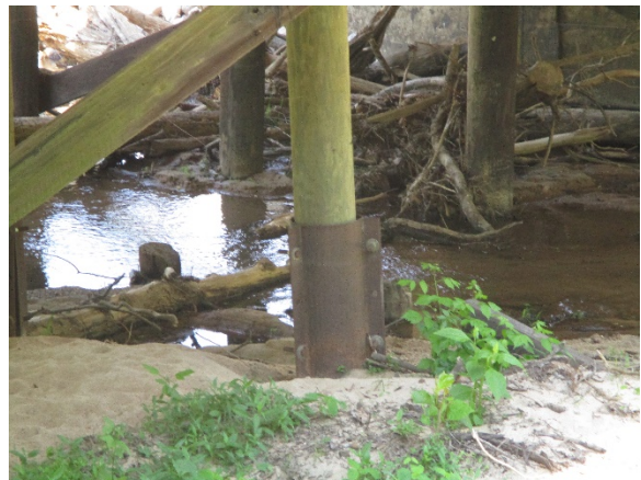
Photo 4. Metal Sleeve on Timber Pile.
