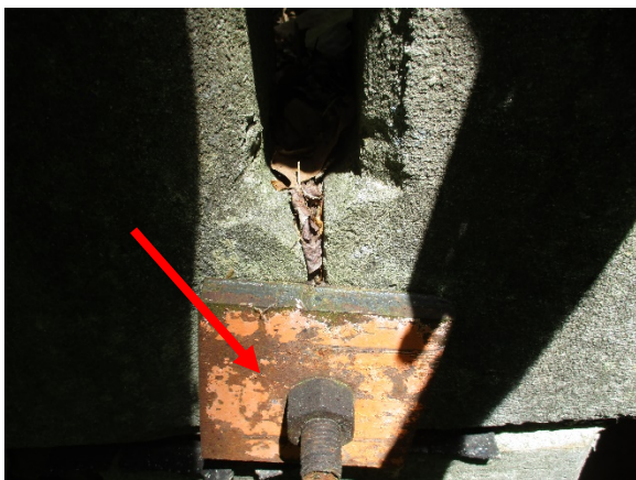
Photo 5. Orange Tie-rod Washer is Positive for Lead.
