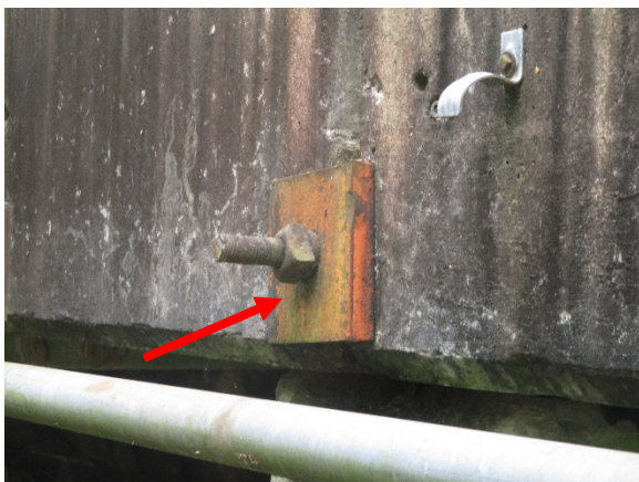
Photo 5. Tie-rod Washer is Positive for Lead.
