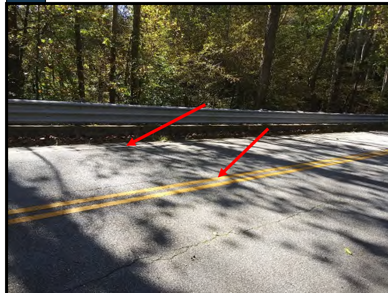
4 Yellow and white stripes tested negative for lead-based paint.
