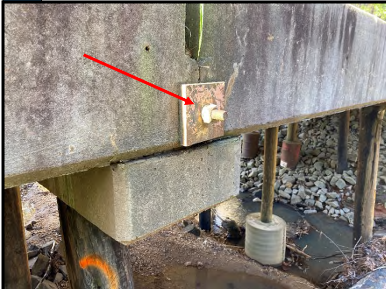
3 Orange metal square washer tested positive for lead-based paint (39.1 mg/cm 2 ).
