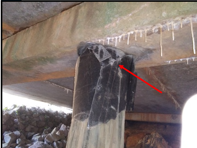
3 Felt paper tested negative for asbestos.
