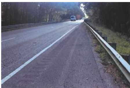
Example 1 – Longitudinal “Kink” in the Guardrail
