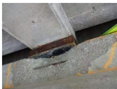
(2240 – Loss of Bearing Area) Condition State 3
