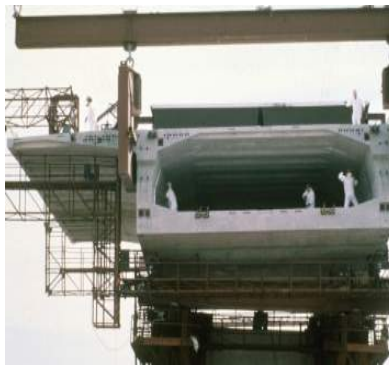
104 Prestressed Closed Web/Box Girder (Segmental)
