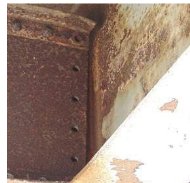
(1020 – Connections) Condition State 4
