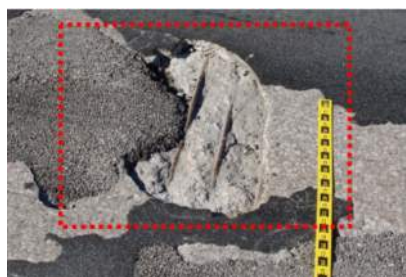
(1090 – Exposed Rebar) Condition State 2
