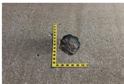
(1080 – Delamination/Spall/Patched Area) Condition State 3
