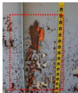
(3420 – Peeling/Bubbling/Cracking) Condition State 3
