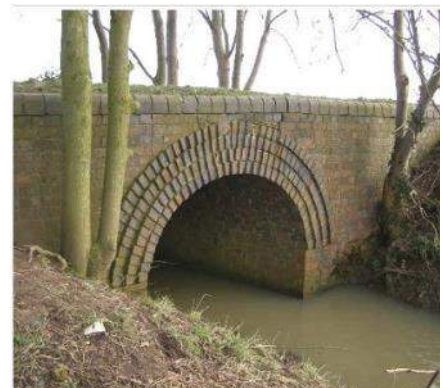
Masonry Culvert
