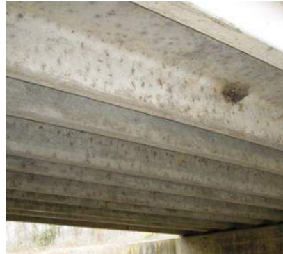
109 Prestressed Concrete Open Girder (Precast Double T)
