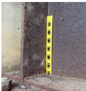
(3430 – Oxide Film Degradation) Condition State 3
