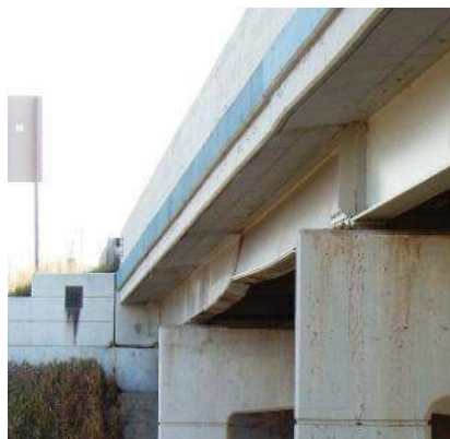
Condition State 3 (Damage)
