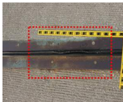
(2330 – Seal Damage) Condition State 3
