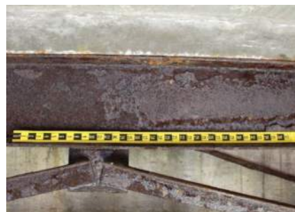
(3430 – Oxide Film Degradation) Condition State 4
