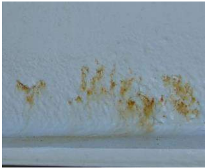
(1000 – Corrosion) Condition State 2
