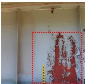
(3420 – Peeling/Bubbling/Cracking) Condition State 2
