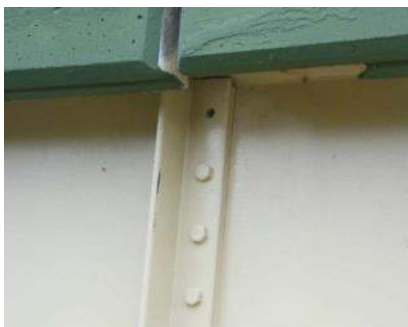
(1020 – Connections) Condition State 2
