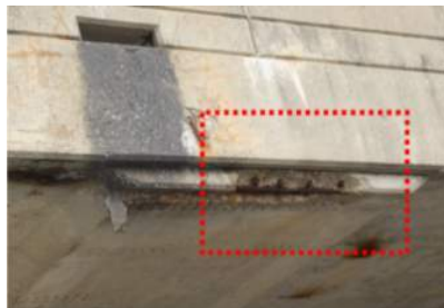
(1090 – Exposed Rebar) Condition State 3
