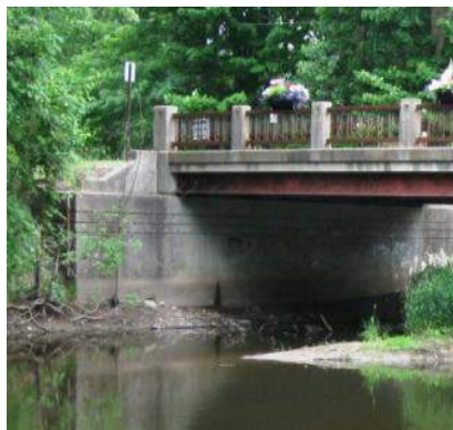
215 Reinforced Concrete Abutment
