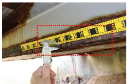
(1000 – Corrosion) Condition State 3
