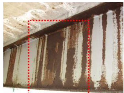
(3420 – Peeling/Bubbling/Cracking) Condition State 4
