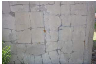
(1130 – Cracking/RC and Other) Condition State 3
