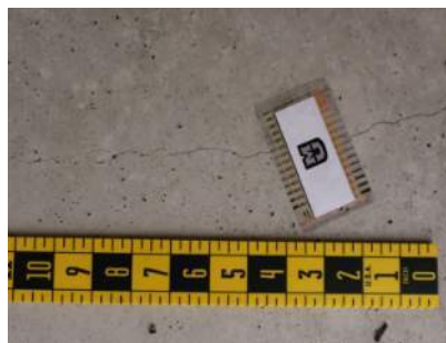
(1110 – Cracking/PSC) Condition State 3
