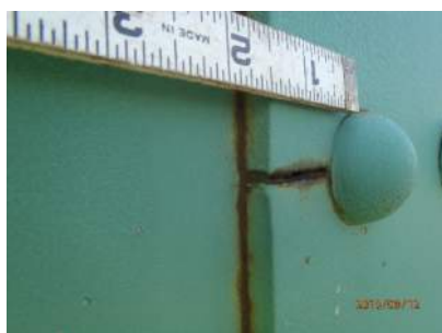
(1010 – Cracking) Condition State 2
