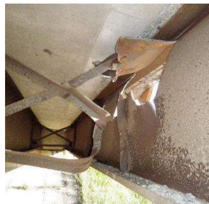
Condition State 4 (Damage)
