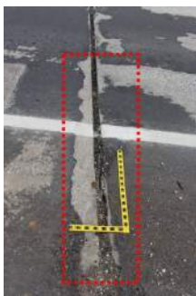
(2350 – Debris Impaction) Condition State 3
