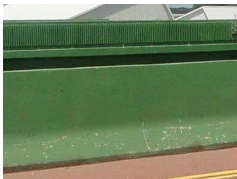
521 Concrete Protective Coating
