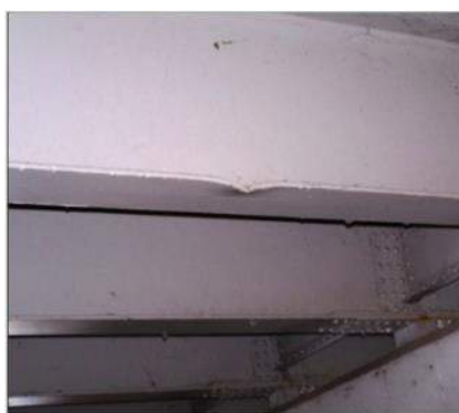
Condition State 2 (Damage)
