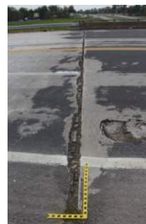
(2350 – Debris Impaction) Condition State 4
