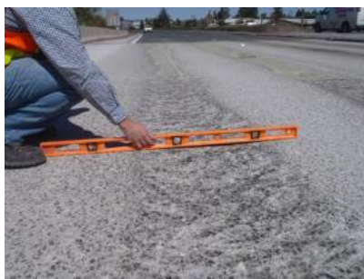
(1190 – Abrasion/Wear) Condition State 3
