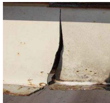
(1010 – Cracking) Condition State 4
