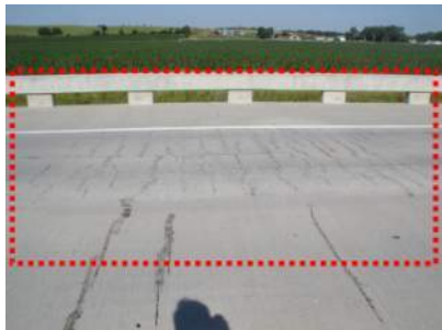
(1130 – Cracking/RC and Other) Condition State 2
