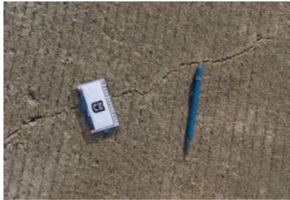
(1130 – Cracking/RC and Other) Condition State 2
