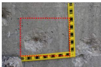
(1080 – Delamination/Spall/Patched Area) Condition State 2
