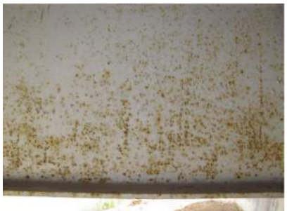
(1000 – Corrosion) Condition State 2
