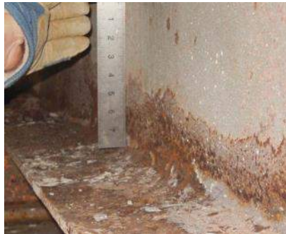
(1000 – Corrosion) Condition State 3
