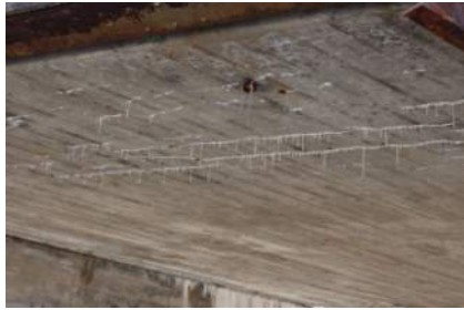
(1120 – Efflorescence/Rust Staining) Condition State 2
