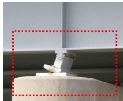
(2220 – Alignment) Condition State 3
