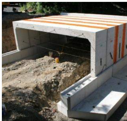
3-Sided Concrete Box Culvert
