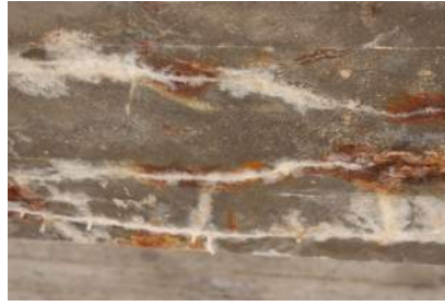
(1120 – Efflorescence/Rust Staining) Condition State 3
