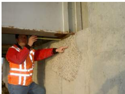
(2240 – Loss of Bearing Area) Condition State 2
