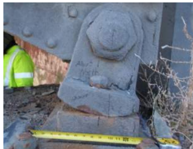
(2220 – Alignment) Condition State 2
