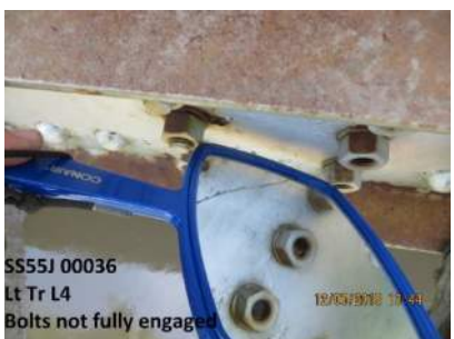
(1020 – Connections) Condition State 2
