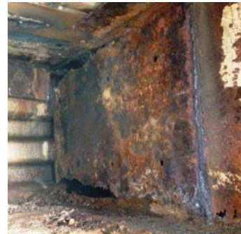
(1000 – Corrosion) Condition State 4
