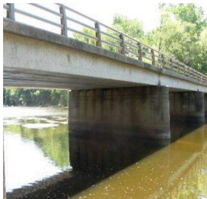
210 Reinforced Concrete Pier Wall
