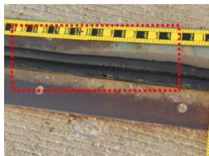
(2330 – Seal Damage) Condition State 2
