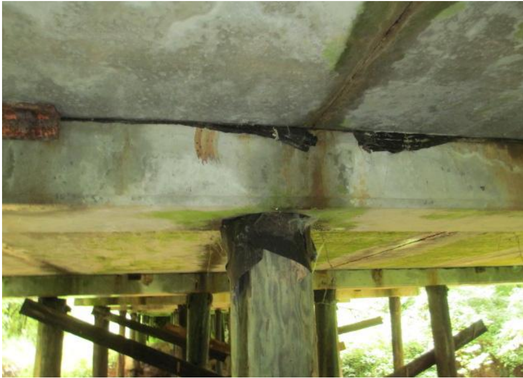
Photo 3 View of thin friction barrier found between wooden piers and concrete caps and thick friction barrier found between the caps and the decking.
