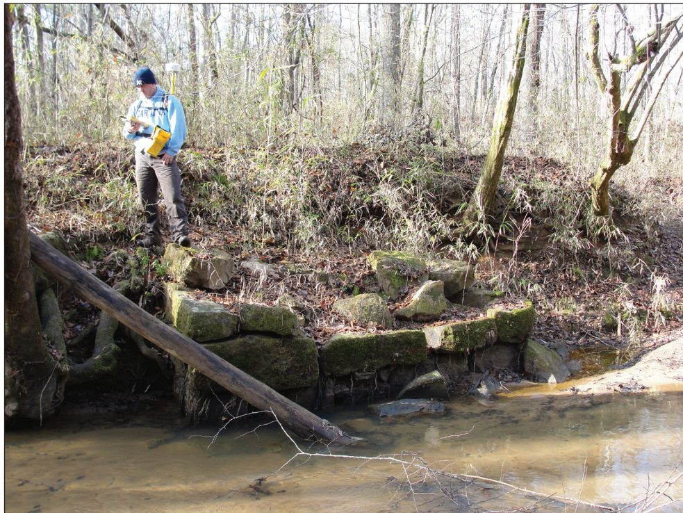
Figure 6. Views of Site 1: northern bridgehead foundation looking north (top); southern bridgehead foundation looking south (bottom).
