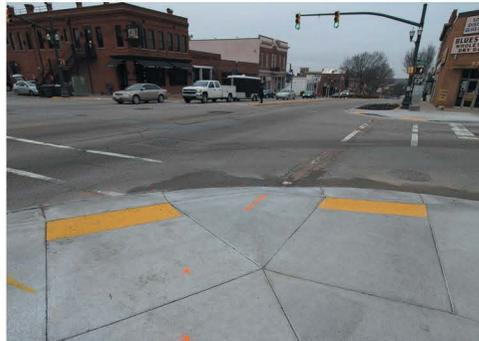
**Detectable Warning Surfaces (DWS)** — a surface of Truncated Domes. A standardized surface feature built in or applied to walking surfaces to warn visually impaired people of hazards on a circulation path. DWS can be identified under foot and by sound on cane contact. Color contrast enables visual detection from surrounding surface.
