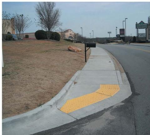
Current specifications require parallel or in-line. If retrofitting existing curb ramp with new DWS, follow SCDOT Standard Drawings.
