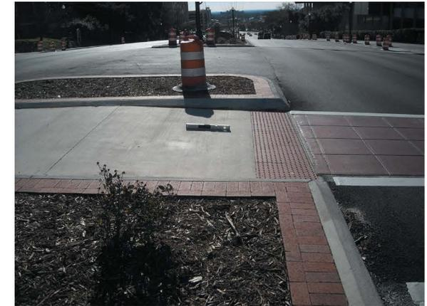
**Pedestrian Refuge Island** — Pedestrian element that provides resting space. Minimum length = 6’-0”; DWS required each side regardless if design is cut-through or uses curb ramps.
