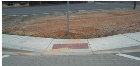
**Truncated Dome** — Individual raised element. 1991 Dome Size and Spacing Requirements:
