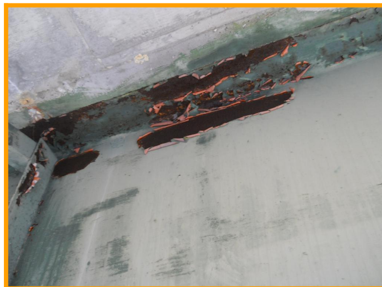
4. Lead-based paint on a beam spanning the Great Pee Dee River.
