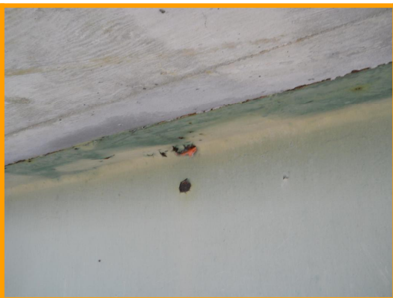
3. Lead-based paint on a beam spanning the Great Pee Dee River.
