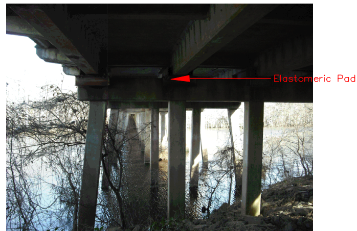
Photograph of Bridge Components (Underneath)
