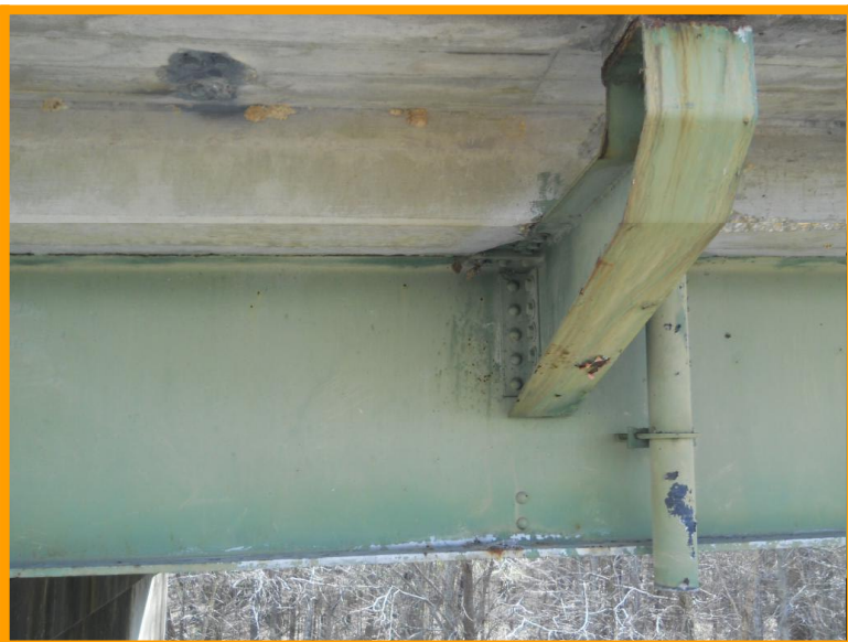
1. Lead-based paint on support associated with a beam spanning the Great Pee Dee River.
