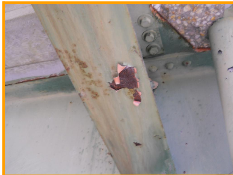
2. Lead-based paint on support associated with a beam spanning the Great Pee Dee River.
