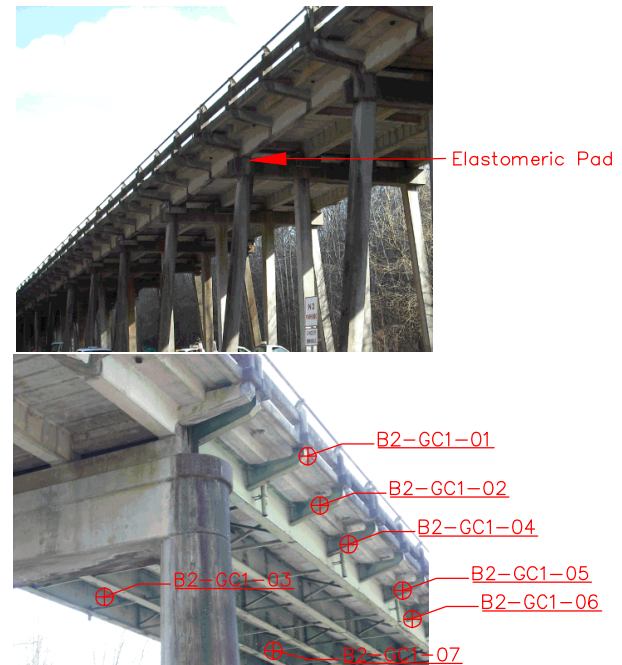
Photograph of Bridge Components (Underneath)
