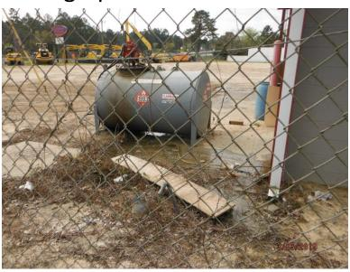
View of Parcel 12 (Company Wrench) within the Project Area. This is the former location of Blanchard Machinery. Note the diesel AST appears rusted around and beneath the fill port. Also note the potential diesel fuel beneath the tank.
