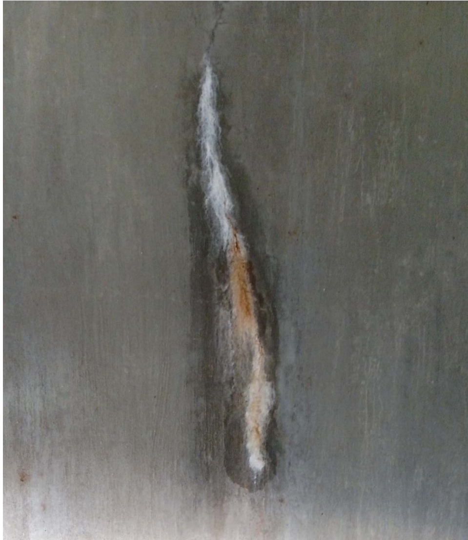
Figure 9 – Water Penetration at End Wall (Southbound)
