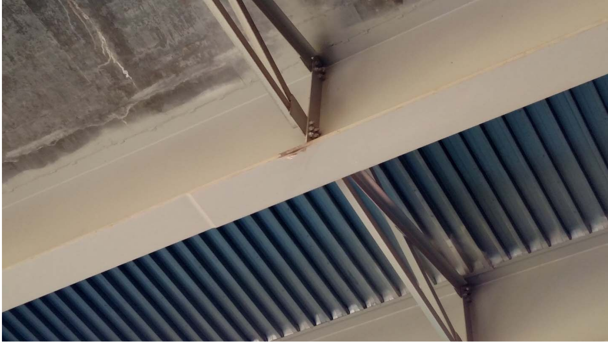
Figure 21 – Paint Peeling at Cross Frame
