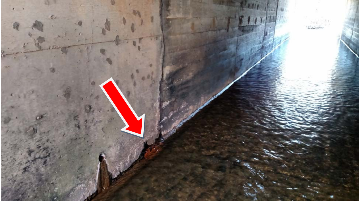
Figure 6 – Deterioration at Wall Base
