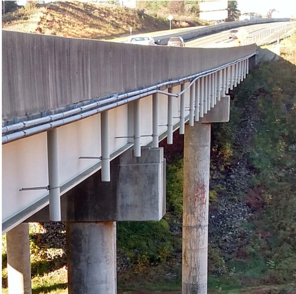
Figure 23 – Utility Line detached from Bridge
