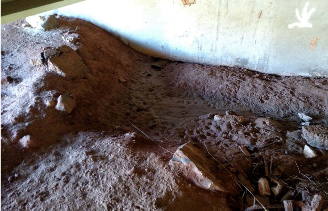
Figure 32 – Water Infiltration under End Bent 4
