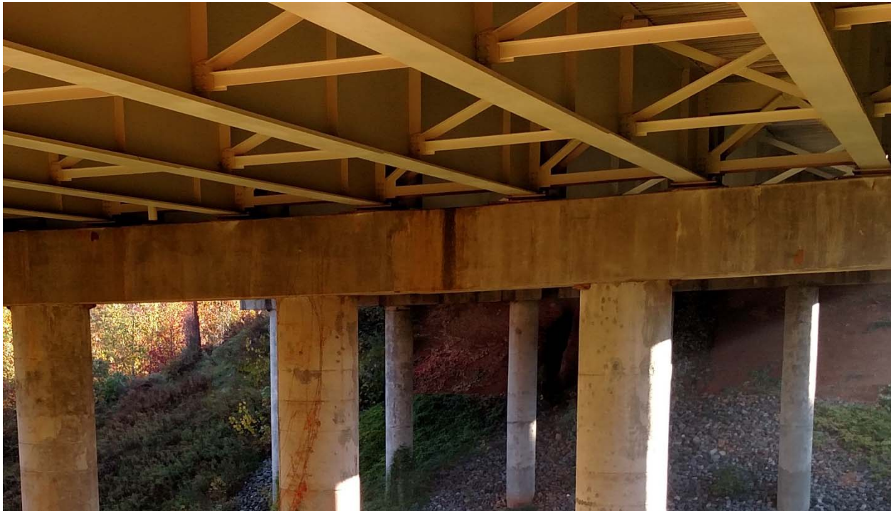
Figure 24 – Staining at Pier Cap (Southbound)
