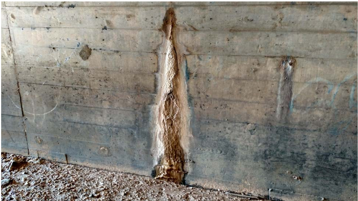
Figure 5 – Crack/leak in culvert wall
