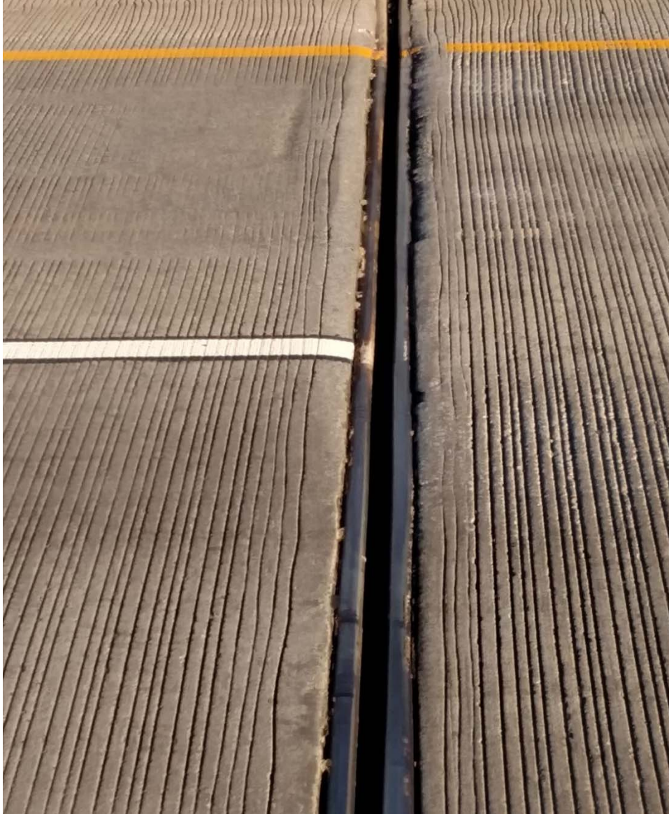
Figure 17 – Strip Seal Expansion Joint (Northbound)
