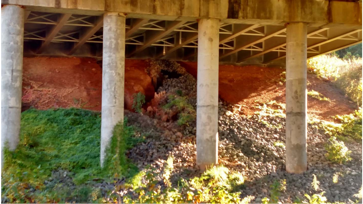
Figure 30 – Embankment Erosion at End Bent 4
