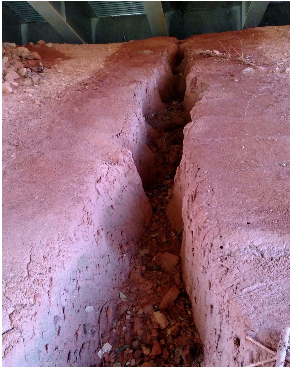
Figure 27 – Embankment Erosion at I-85 Northbound Closure Pour (End Bent 1)
