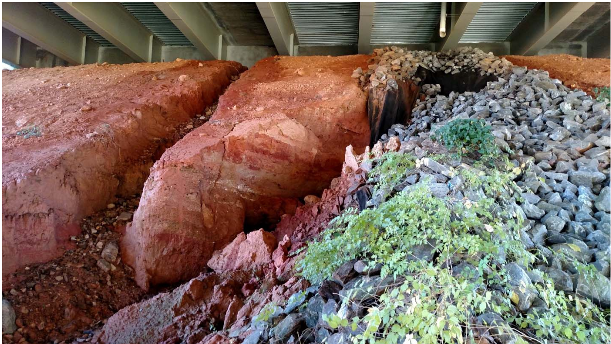
Figure 31 – Embankment Erosion at End Bent 4
