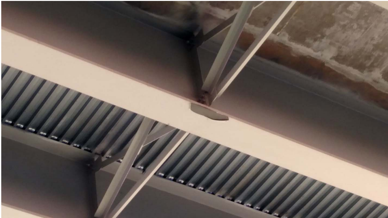
Figure 22 – Paint Peeling at Cross Frame
