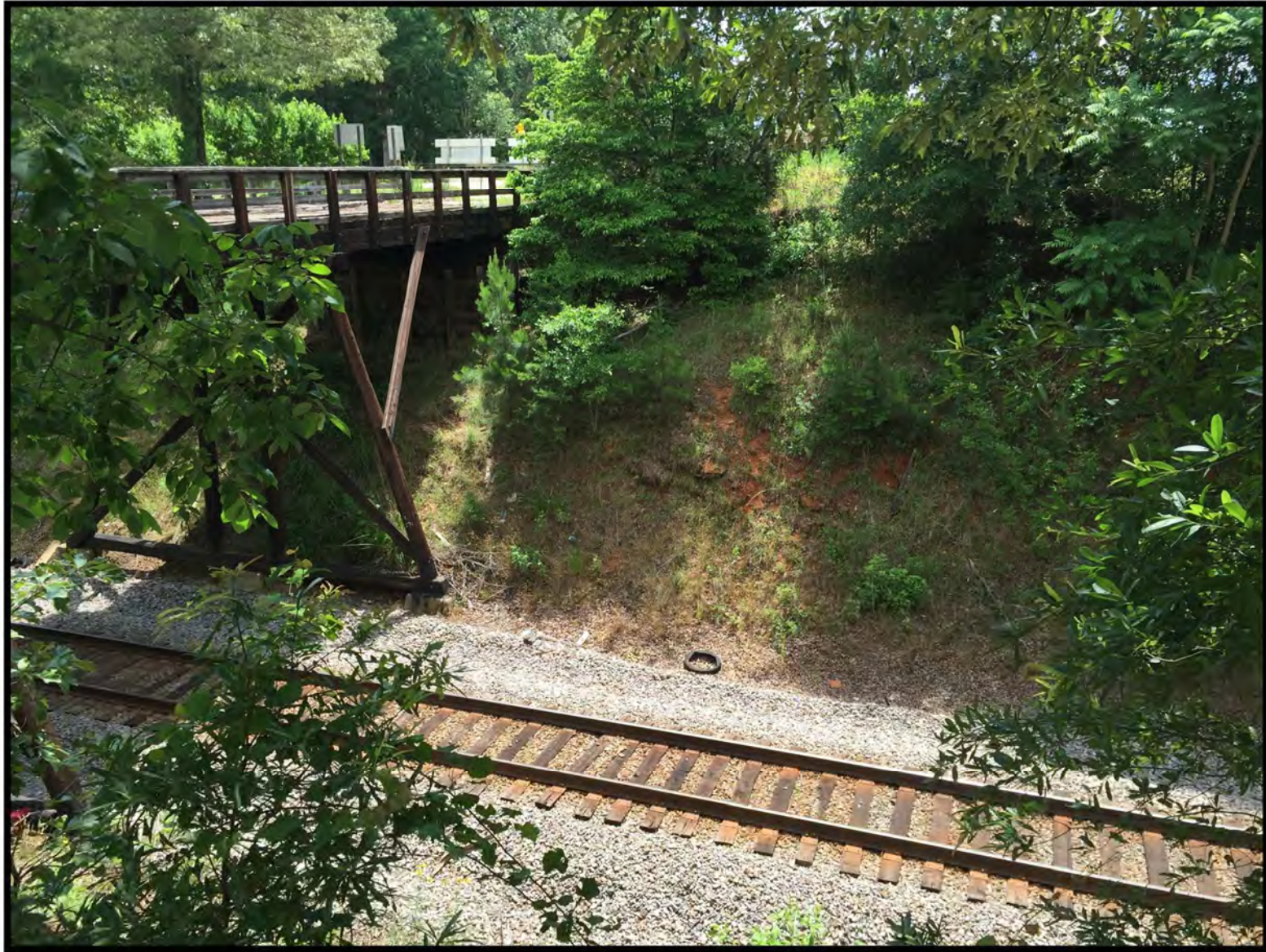
Photograph 9: Looking east at Conway Black Road Bridge.
