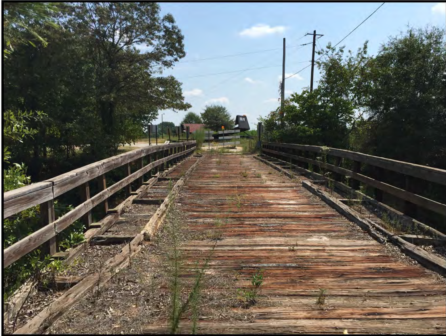
Photograph 11: Looking east at Conway Black Road Bridge.
