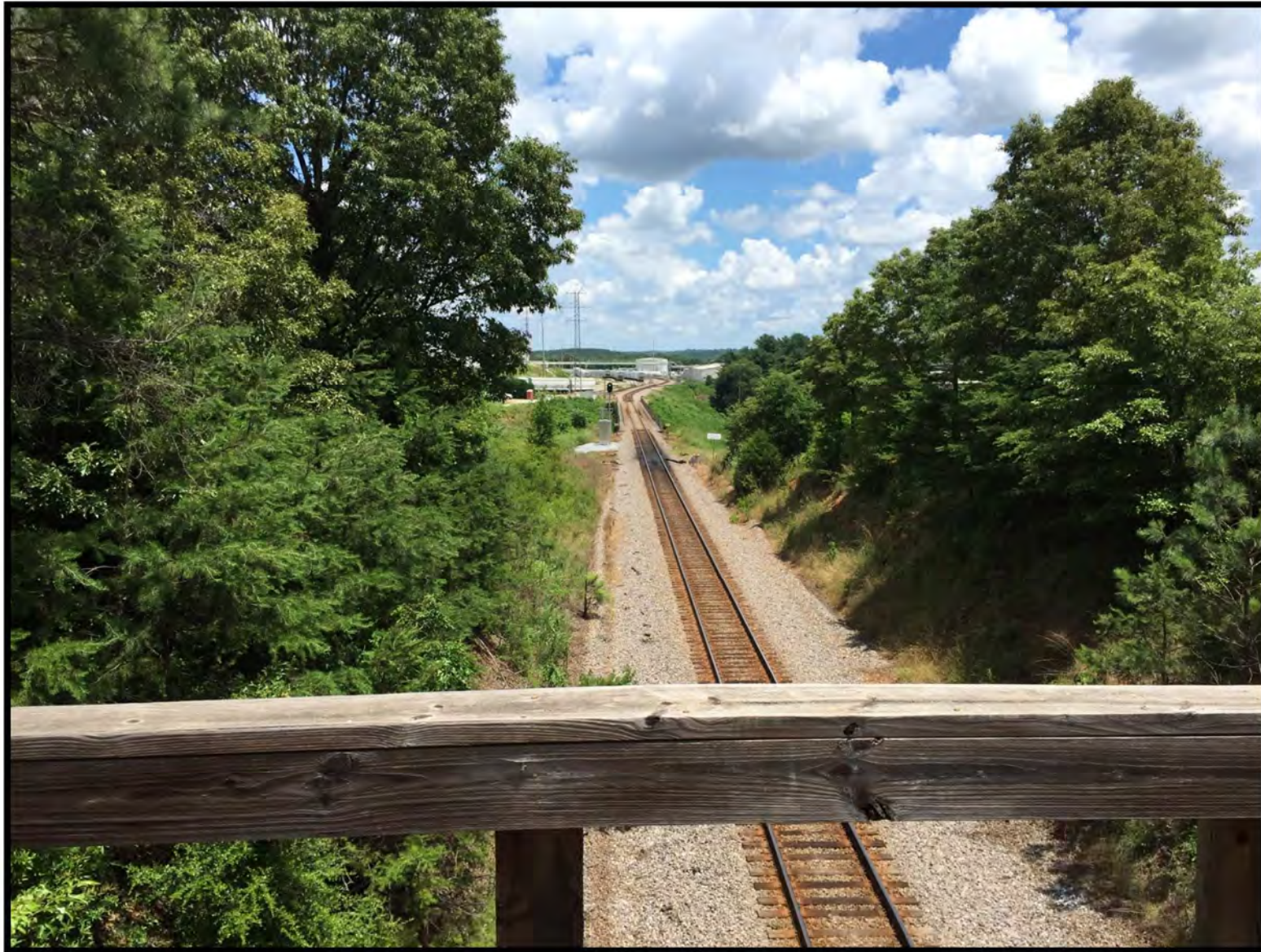
Photograph 5: Looking north from existing Conway Black Road Bridge at study area.
