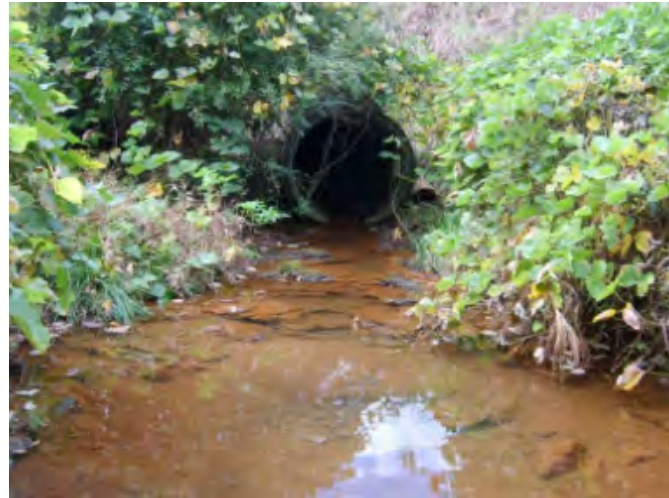
View of 60" RCP on UT to Pole Bridge Branch at I-85
