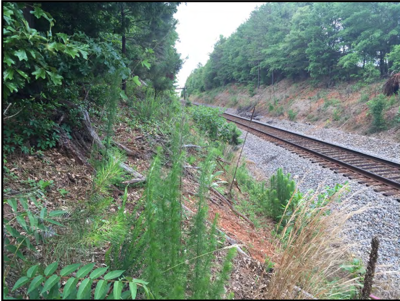
Photograph 4: Looking north along existing railroad slopes.
