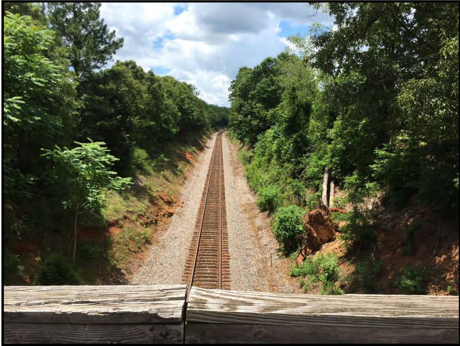
Photograph 6: Looking south from existing Conway Black Road Bridge at study area.
