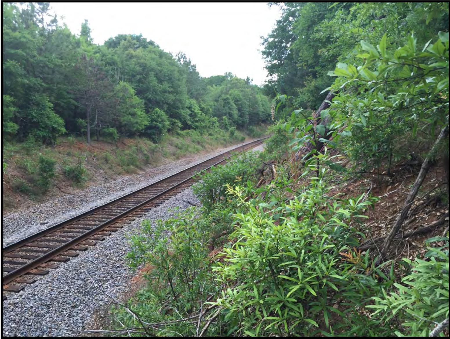
Photograph 3: Looking south along existing railroad slopes.
