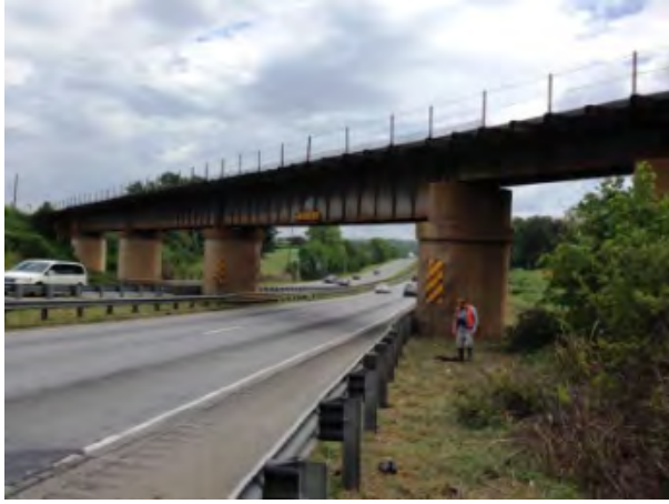
View of CSX Railroad Bridge over I-85
