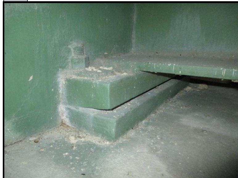
4 The green paint on the bolt plate tested positive for lead-based paint (0.8 – 1.2 mg/cm 2 ).
