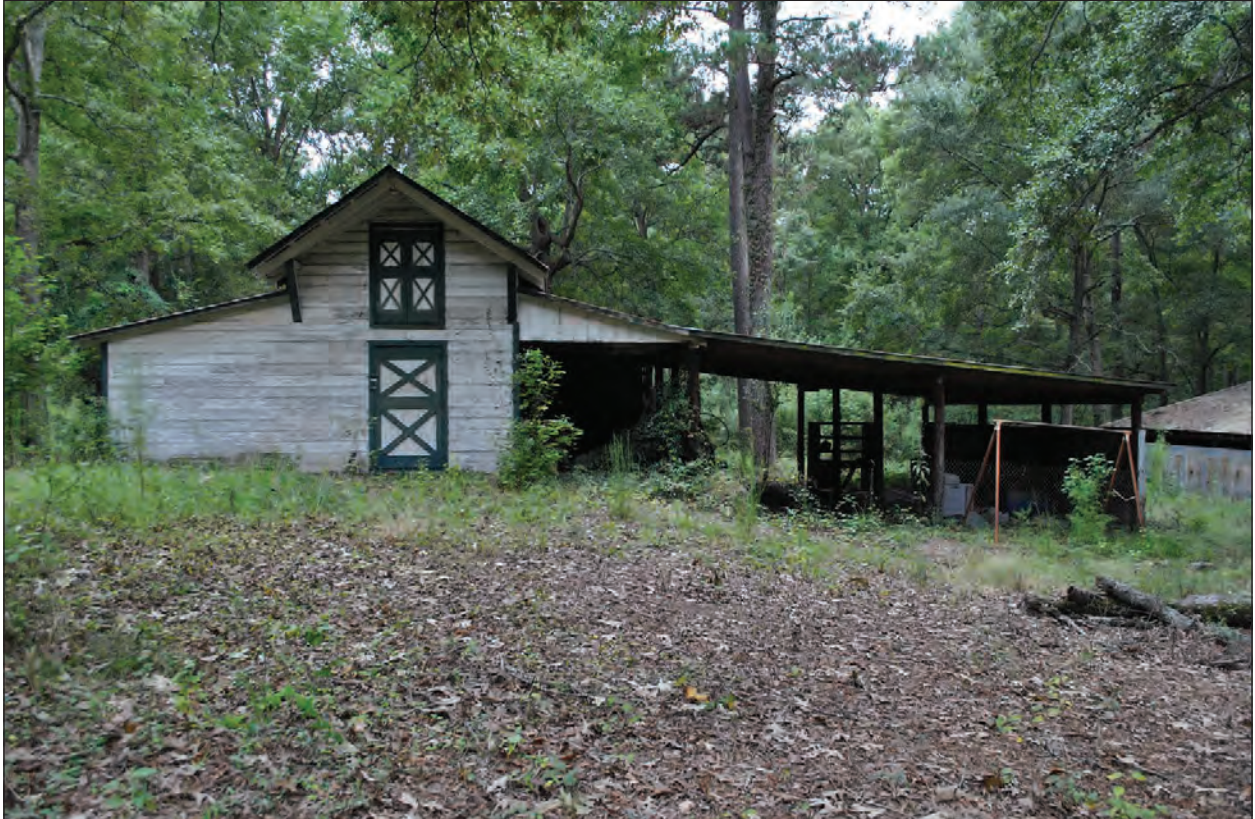
Figure 5. View of Resource 6382.01, looking southwest.
