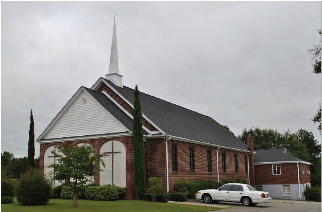
Figure 12. View of Resource 6386, looking east.
