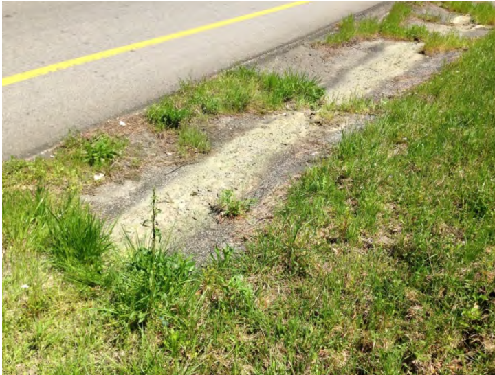
OP-0683 (not located, assumed as buried)
