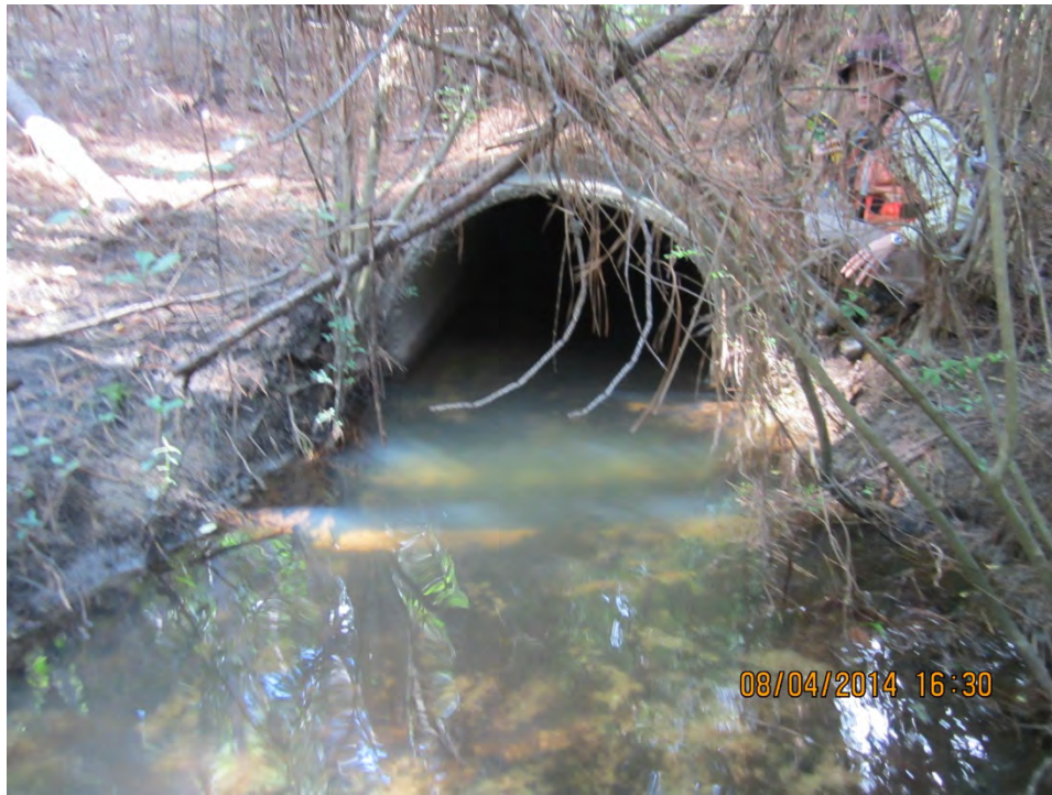
Photograph #1 – s2 (looking northeast)
