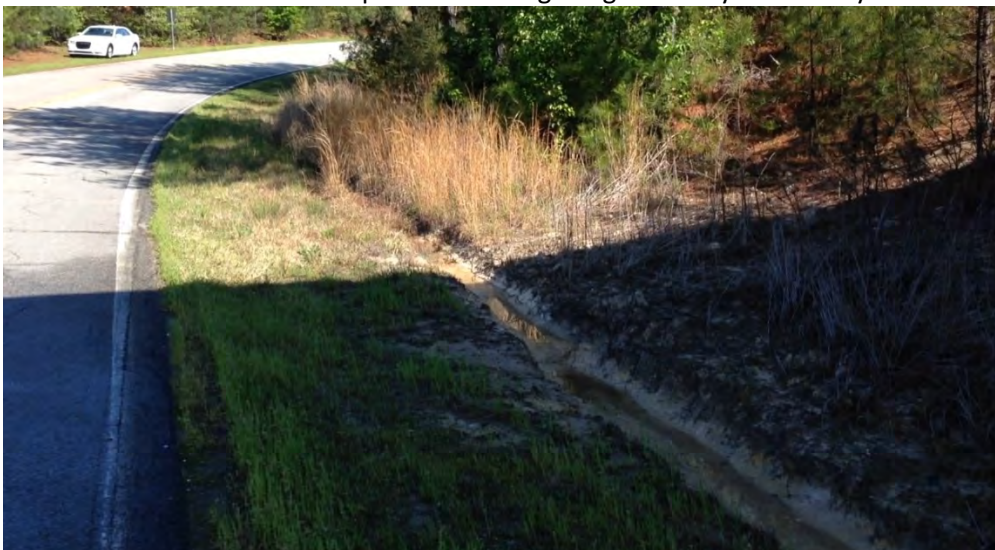
OP-1698 (not located, assumed as buried)
