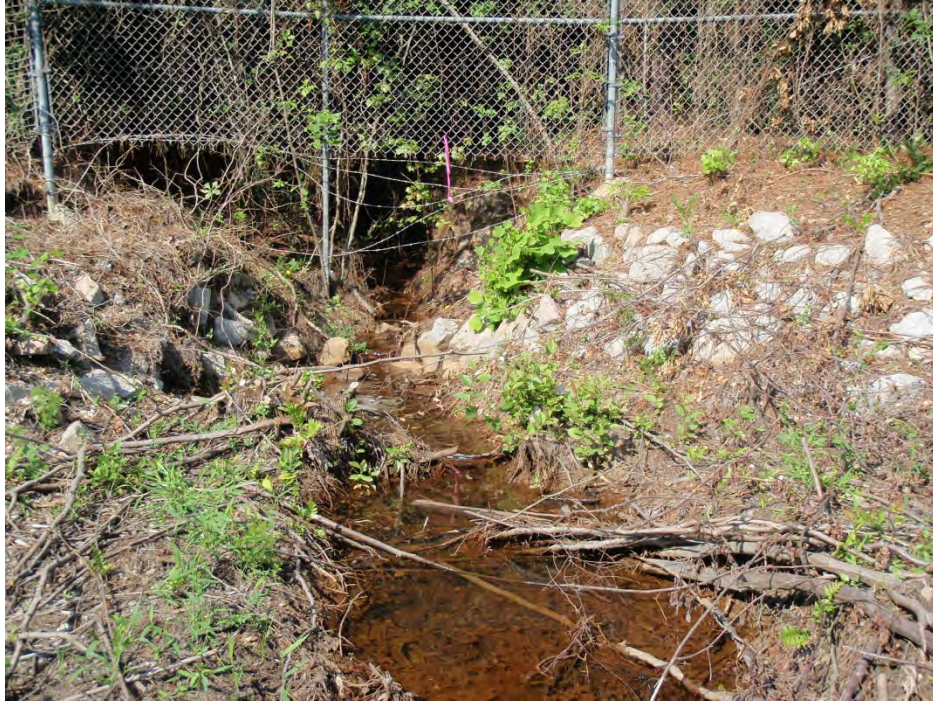
Photograph #14 – s20 (looking northeast)
