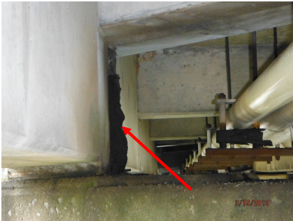
Asbestos-Containing Expansion Joint Material
