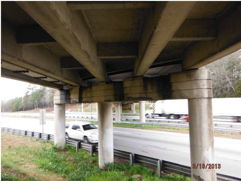
Underside of bridge with concrete beams and diaphragms
