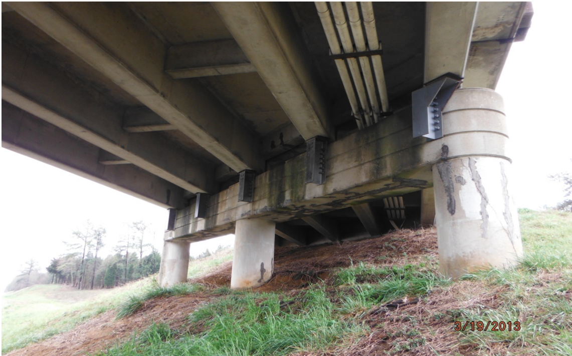
Interior bent cap with silver-painted I-beam sections
