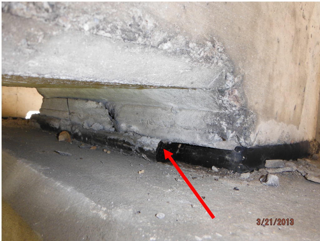
Asbestos-Containing Interior Bent Cap Pads
