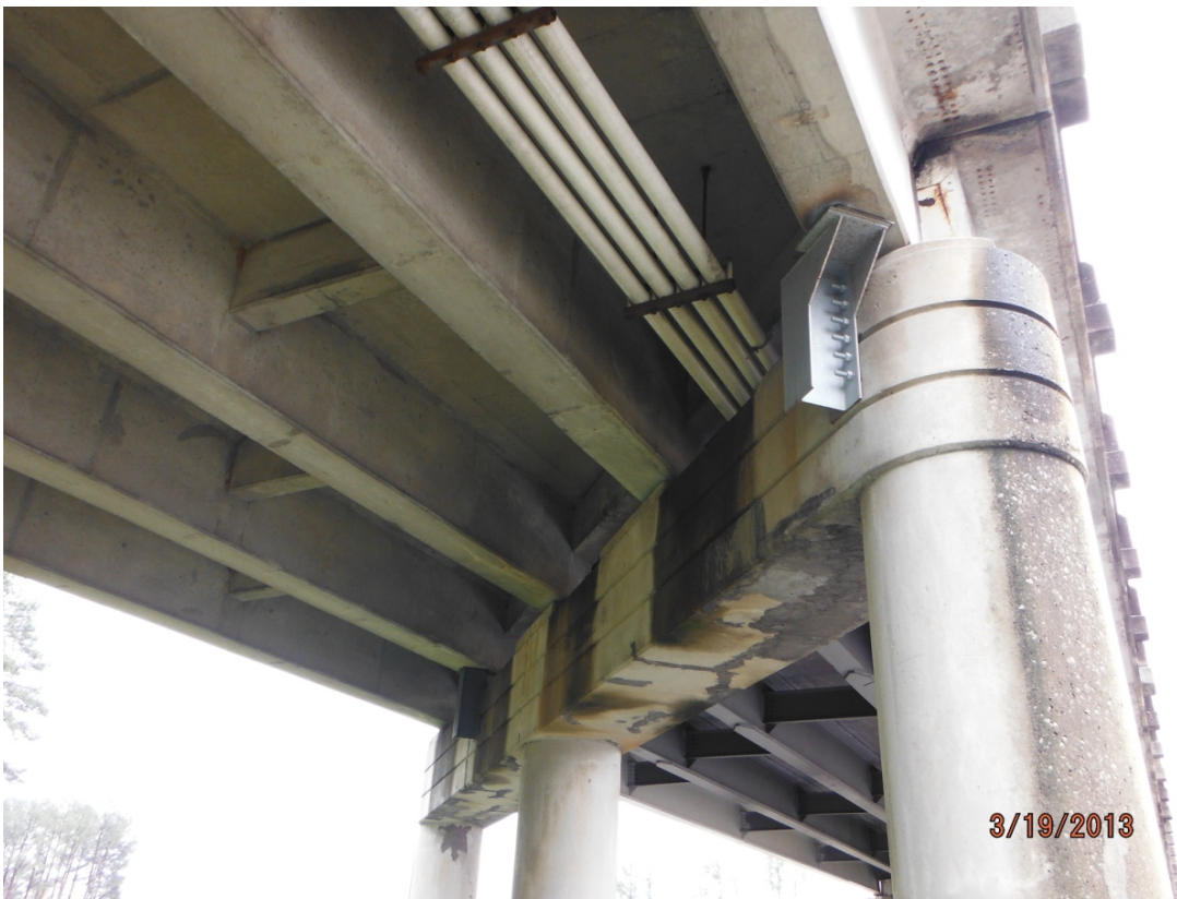
Interior bent cap with gray-painted I-beam sections
