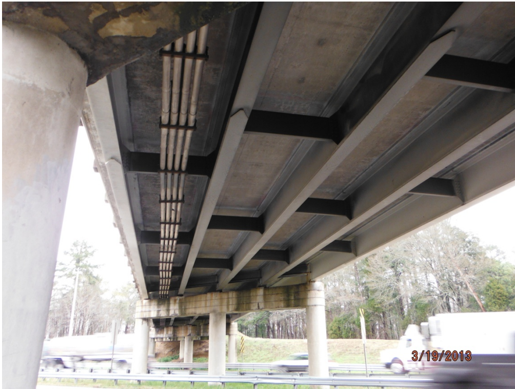
Underside of bridge span with steel beams and diaphragms
