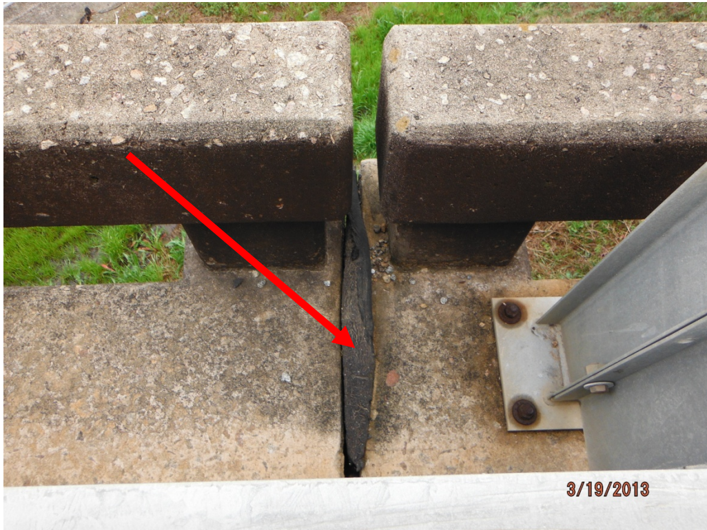
Asbestos-Containing Expansion Joint Material
