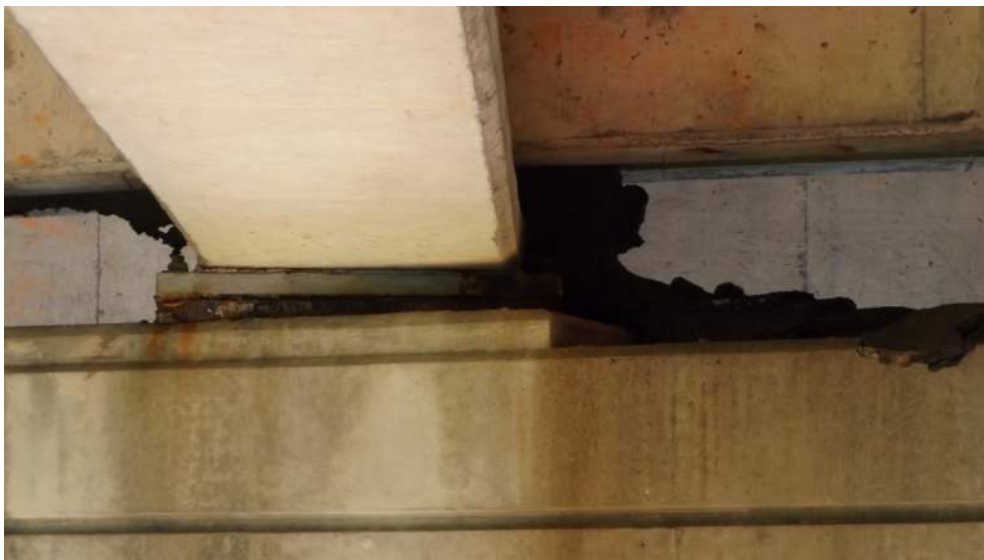
Figure 7 - Expansion Joint material falling through joint opening
