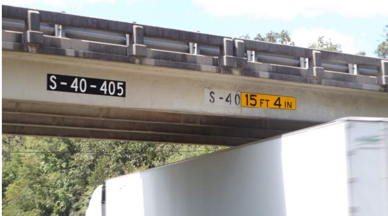
Figure 11 - Vertical Clearance
