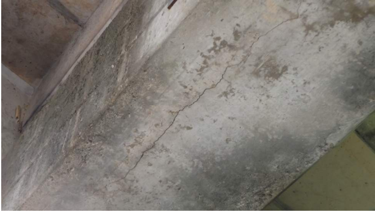
Figure 10 - Crack in Bottom of Pier Cap
