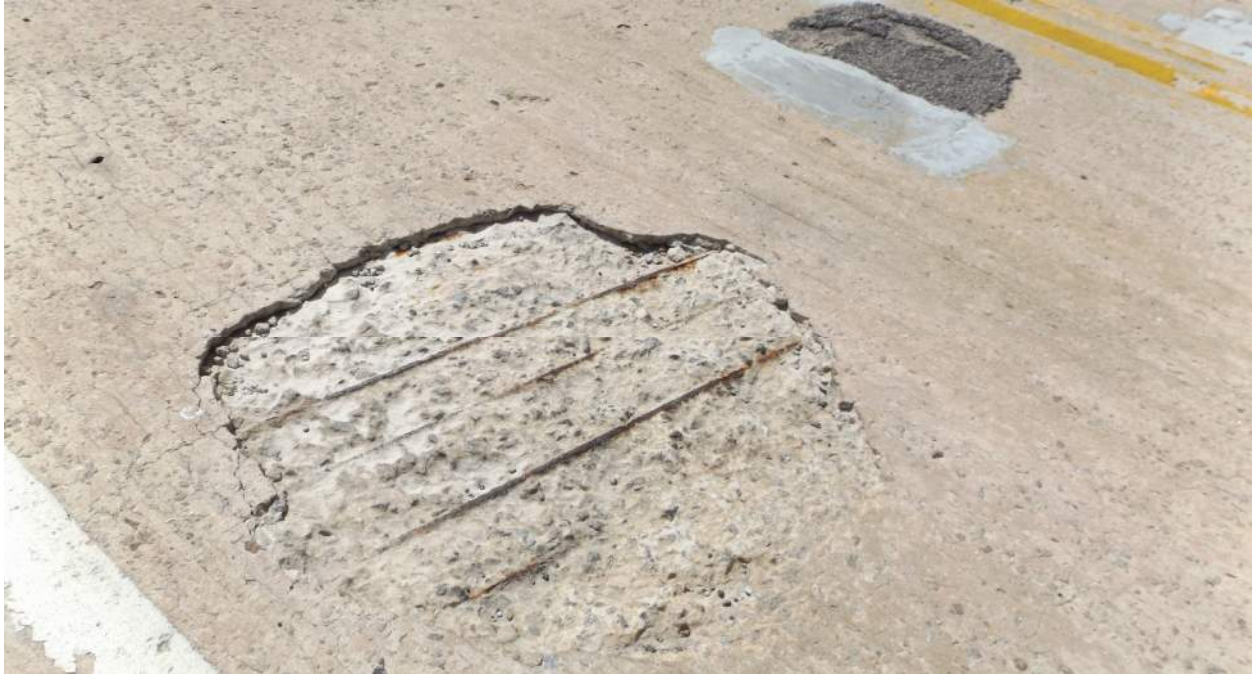
Figure 4 – Exposed Rebar in Concrete Deck
