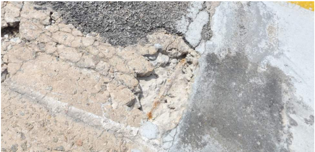
Figure 5 - Exposed Rebar in Concrete Deck
