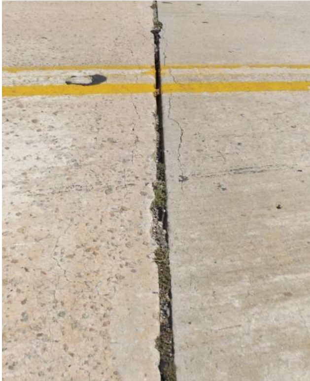
Figure 7 - Expansion Joint
