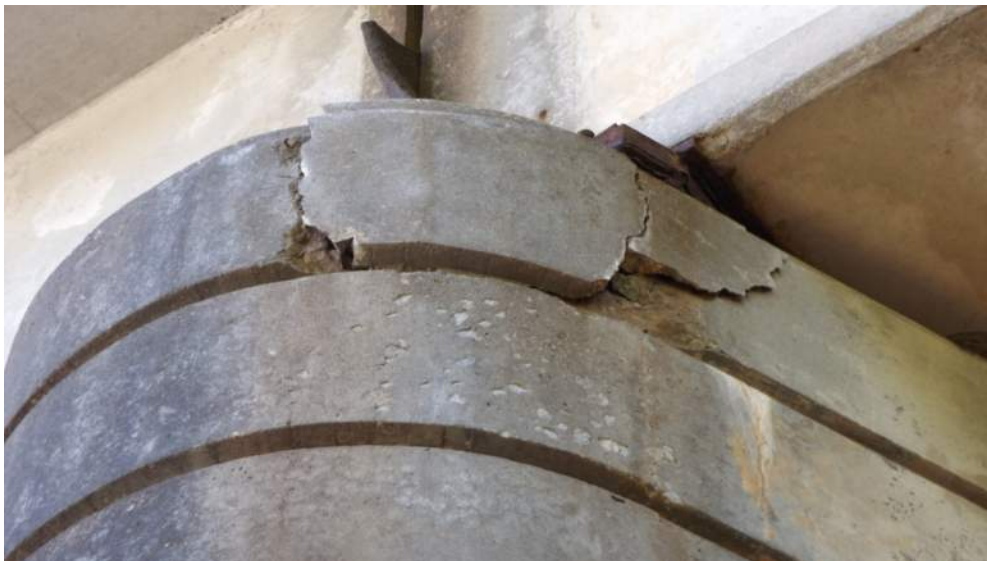
Figure 9 - Spall on Top of Pier Cap
