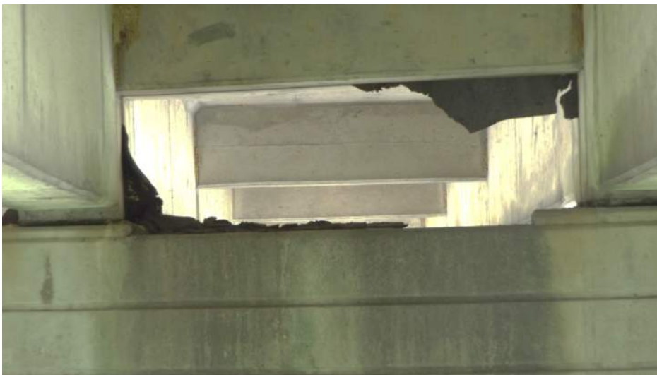
Figure 8 - Expansion Joint material falling through joint opening
