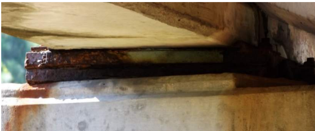
Figure 5 - Bearing Corrosion
