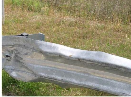
**Minor** damage is usually more aesthetic than structural. In most cases the damage may not be bad enough to warrant repair. There may be numerous types of dings all along its length and still be very safe and perform properly. As long as the rail can perform its intended purpose, repairs should not be made until convenient to the work schedule and all severe and moderate repairs have been completed.
