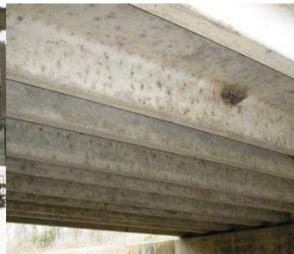
109 Prestressed Concrete Open Girder (Precast Double T)
