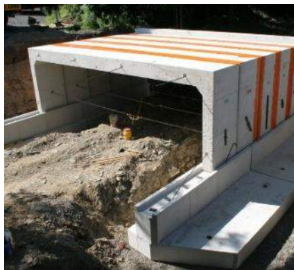
3-Sided Concrete Box Culvert
