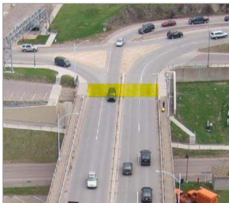
321 Reinforced Concrete Approach Slab
