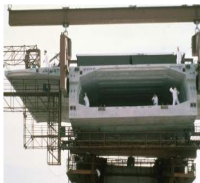
104 Prestressed Closed Web/Box Girder (Segmental)
