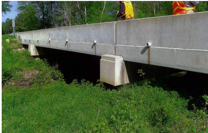
Photo from March 2017 inspection
