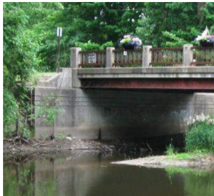
215 Reinforced Concrete Abutment
