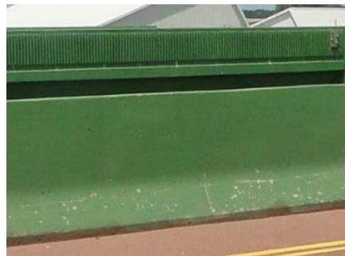
521 Concrete Protective Coating
