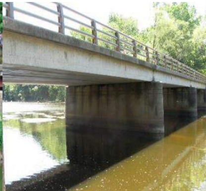
210 Reinforced Concrete Pier Wall
