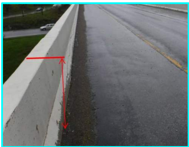
Figure 5.3.1.9.1.2-2 Reveal Measurement at Barrier
