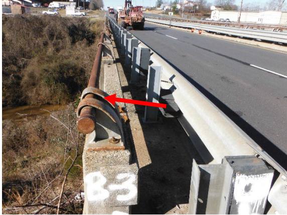
Photo 1. LBP on silver painted original metal guardrails.
