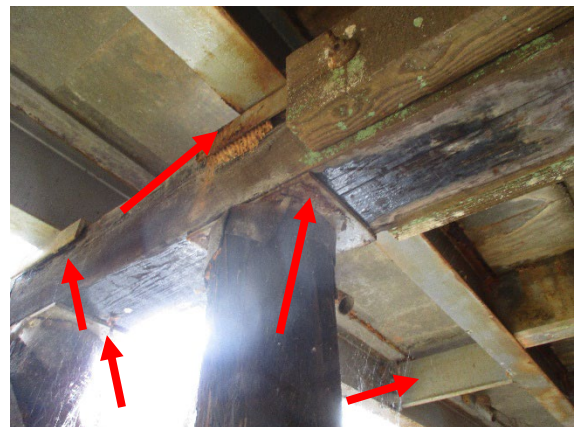
Photo 6 LBP on Gray Girder Bearing Plates, Gray Timber Pile Plates and Diaphragms.
