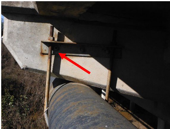
Photo 3. LBP on utility pipe support bracket.
