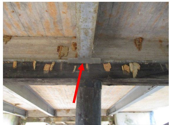
Photo 6 LBP on Gray Girder Bearing Plates.
