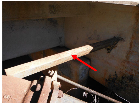
Photo 4. LBP on utility pipe support bracket.
