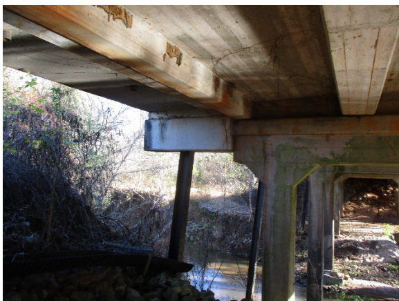
Photo 5. New Bridge Addition Underside View.
