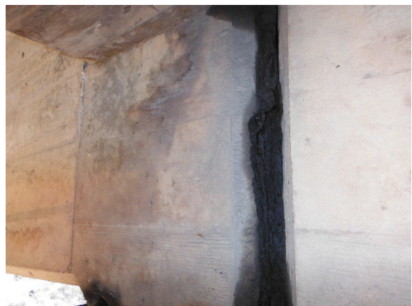
Photo 6. Black Expansion Joint Material
