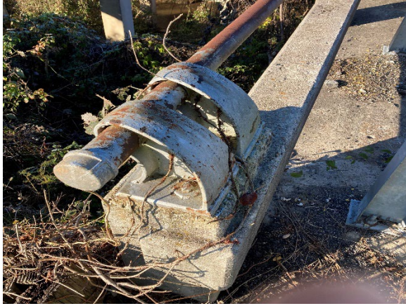
Photo 1. LBP containing silver painted original metal guardrail.
