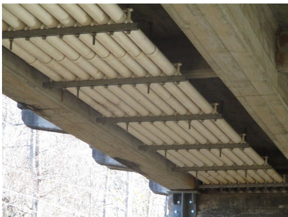
Photo 5. Nine (9) Communication Conduits attached to the North Underside of Bridge.
