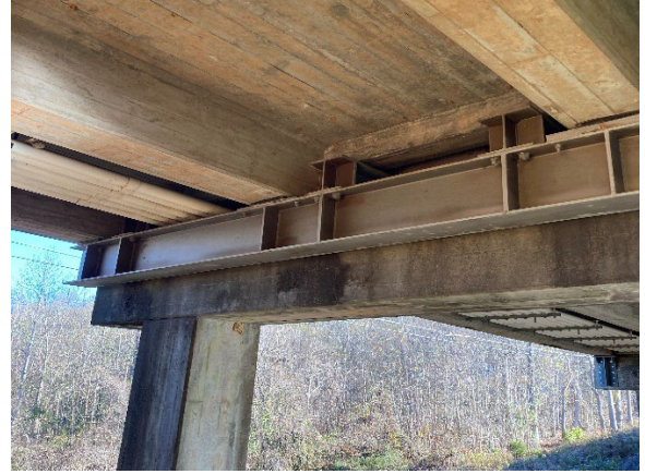
Photo 2. View of Bent Cap Repair
