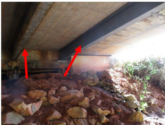
Photo 5. LBP on Gray Horizontal Steel Girders.
