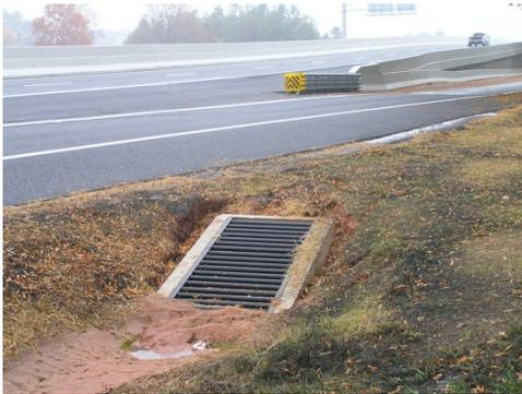
Use **Pipe End Structure** (719-615-00) when specified in the plans or special provisions. Use pipe end structure in locations where pipe exposed end faces the direction of traffic. Pipe end structures may be used in other locations if approved by the RCE.
