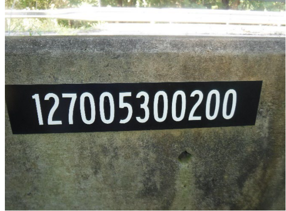
Photo 2. SCDOT Bridge Number Placard Attached to Concrete Curb.
