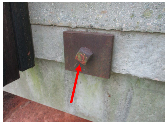
Photo 6 LBP on Rust Colored Tie-Rod Washers on Sides of Bridge Deck.
