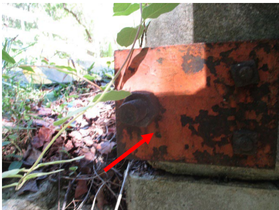
Photo 5. LBP on Orange/Rust Tie-Rod Washer on Sides of Bridge Deck.
