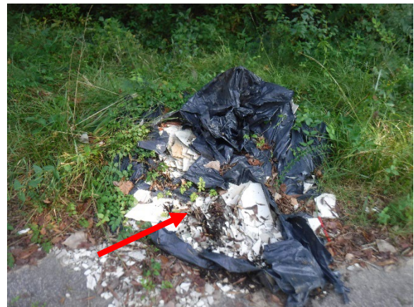
Photo 6. ACM Transite Siding Debris on SCDOT Right Away.
