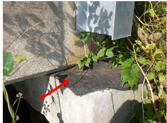
Photo 4. ACM Black bond Break Pad Material
