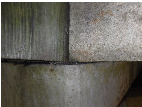
Photo 5. Bearing Pad Material.
