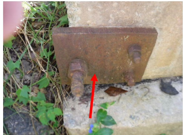
Photo 4. LBP on Rust Colored Tie-Rod Washer.
