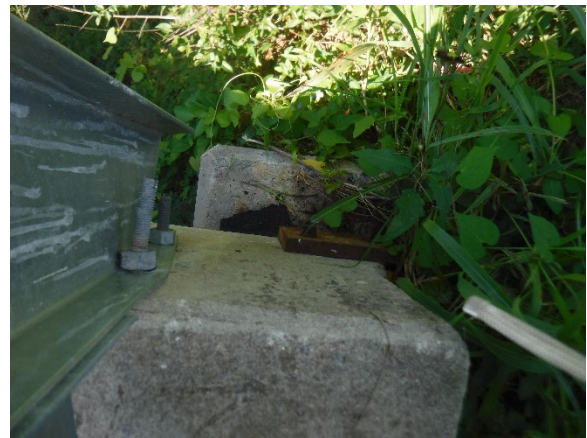
Photo 4. Bond Break Pad Material.
