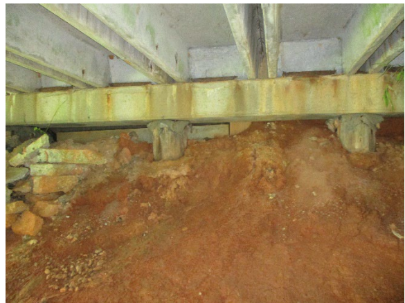
Photo 4. Timber Pile Cap Felt.
