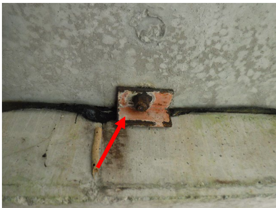
Photo 5. LBP on Orange/Rust L-Bracket.
