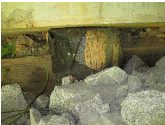
Photo 5. Timber Pile Cap Felt.
