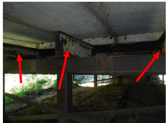
Photo 6 LBP on Gray/Rust Large Horizontal I-Beams.
