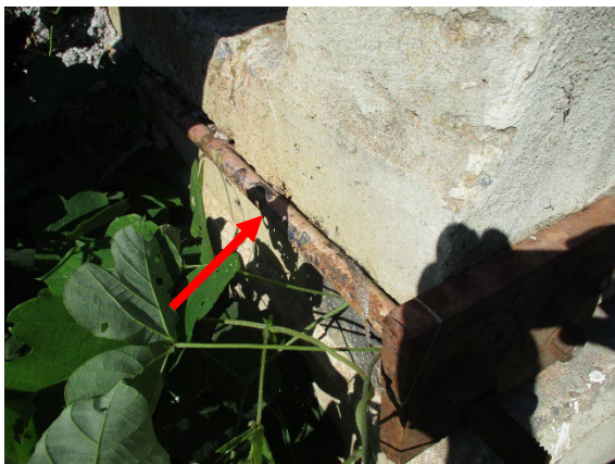
Photo 5. LBP on Exposed Tie-Rod.
