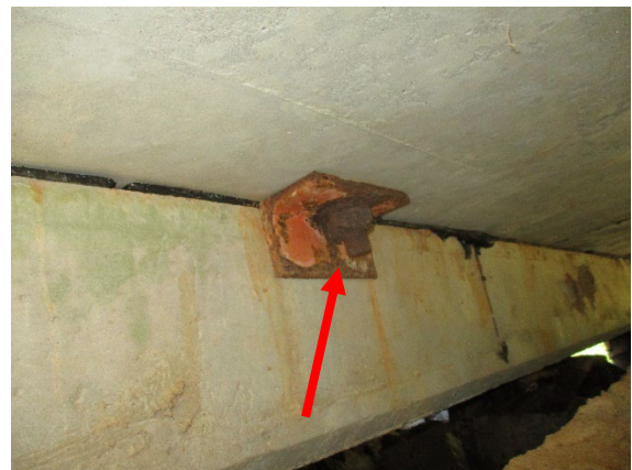
Photo 6 LBP on Orange/Rust L-Bracket on Underside of Bridge Deck.
