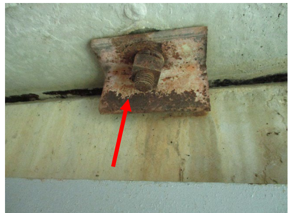
Photo 6 LBP on Orange/Rust L-Bracket.
