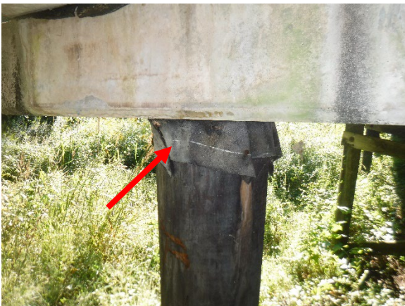
Photo 5. ACM timber Pile Cap Felt.
