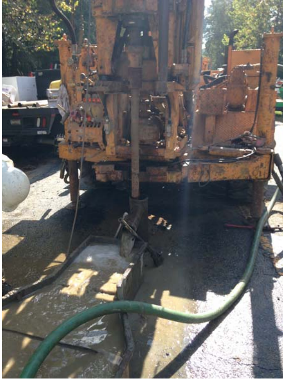
Photo 1. Drill Rig at B-1
