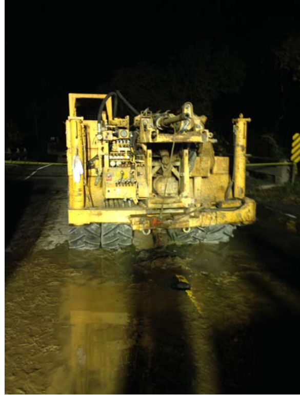
Photo 2. Drill Rig at B-2
