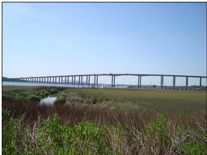
I-526 Bridge over the Wando River
