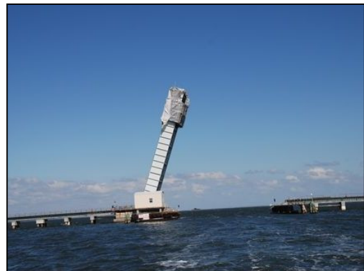
View of a typical bascule bridge
