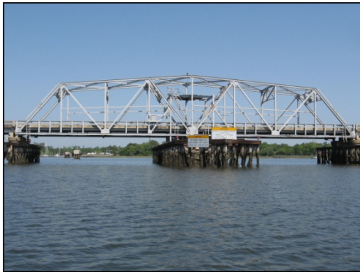
View of the existing swing bridge
