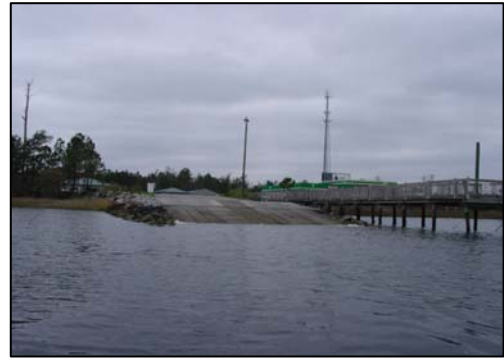
Boat Landing and Gas Station
