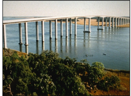
View of a typical fixed span bridge (I-526 over the Wando River downstream)
