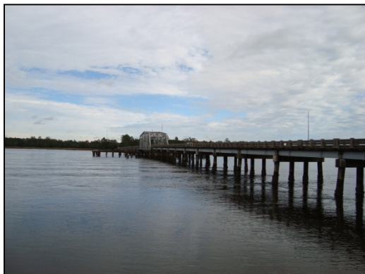
View of the bridge
