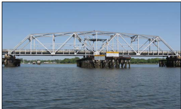
Existing SC-41 Bridge
