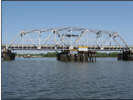
View of the existing swing bridge
