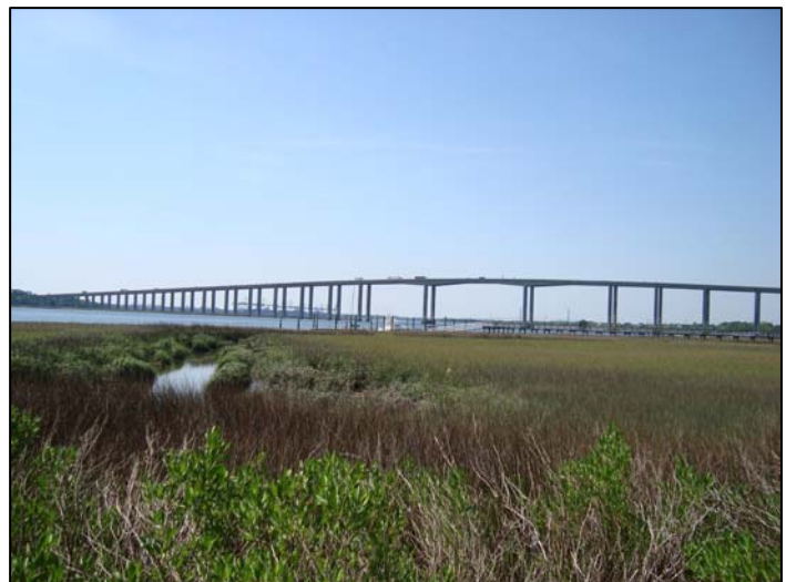
I-526 Bridge over the Wando River
