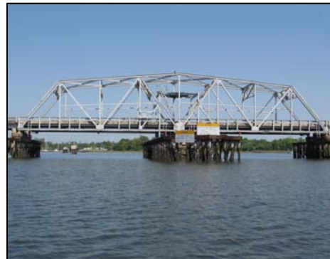
Existing SC-41 Bridge
