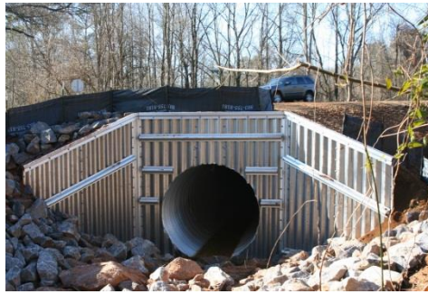
Use Pipe Wingwall
