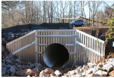
Use Pipe Wingwall
