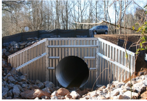
Use Pipe Wingwall
