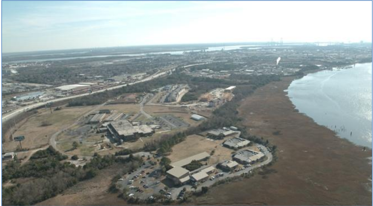
FIGURE 2-2 AERIAL VIEW OF THE STUDY AREA (LOOKING SOUTHEAST)
