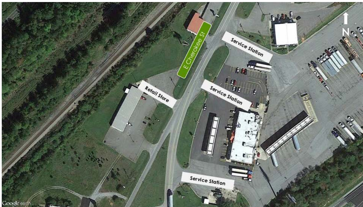
Figure 26 – Service Station/Retail Store Driveways at E. Cherokee Street
