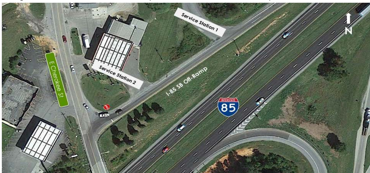
Figure 29 – Service Station Driveways at I-85 Southbound Off-Ramp to E. Cherokee Street
