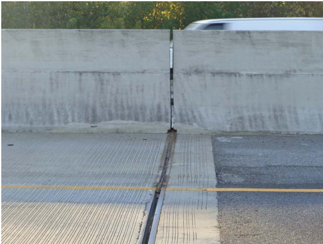
Figure 4: Joint View from Deck (End Bent 4)
