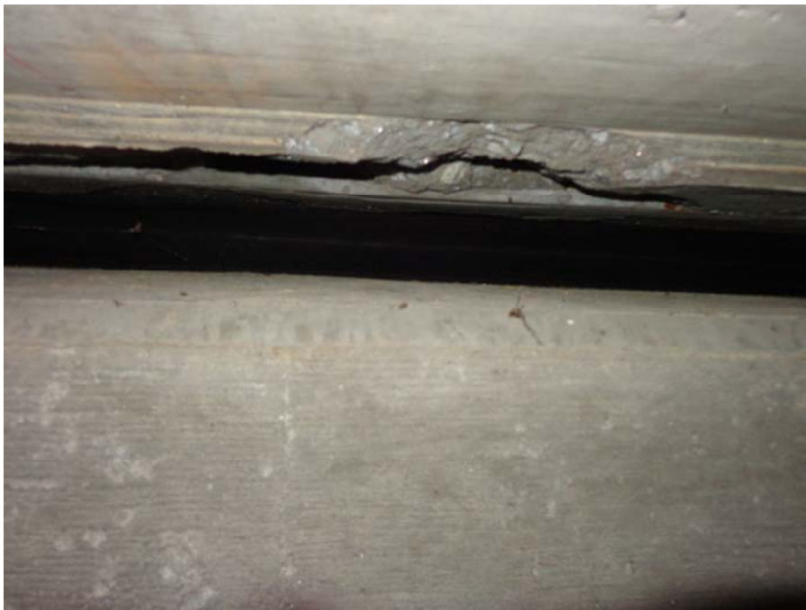
Figure 4: Typical Underside of Joint (End Bent 6)
