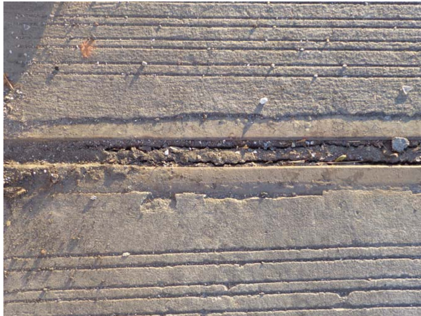
Figure 2: Debris in Joint (End Bent 1)
