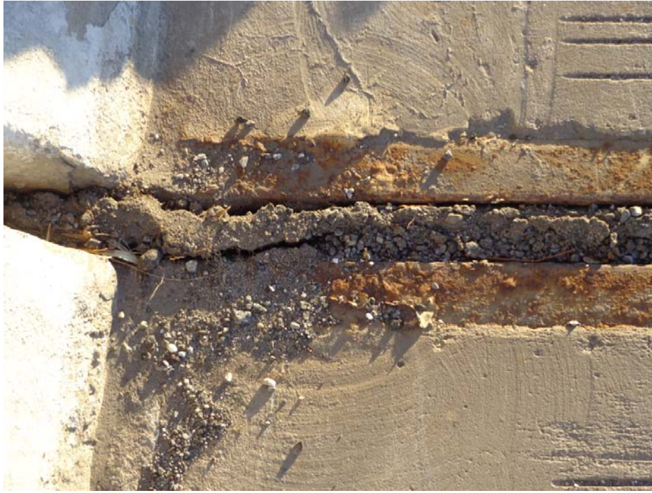
Figure 2: Debris in Joint along Barrier (End Bent 1)
