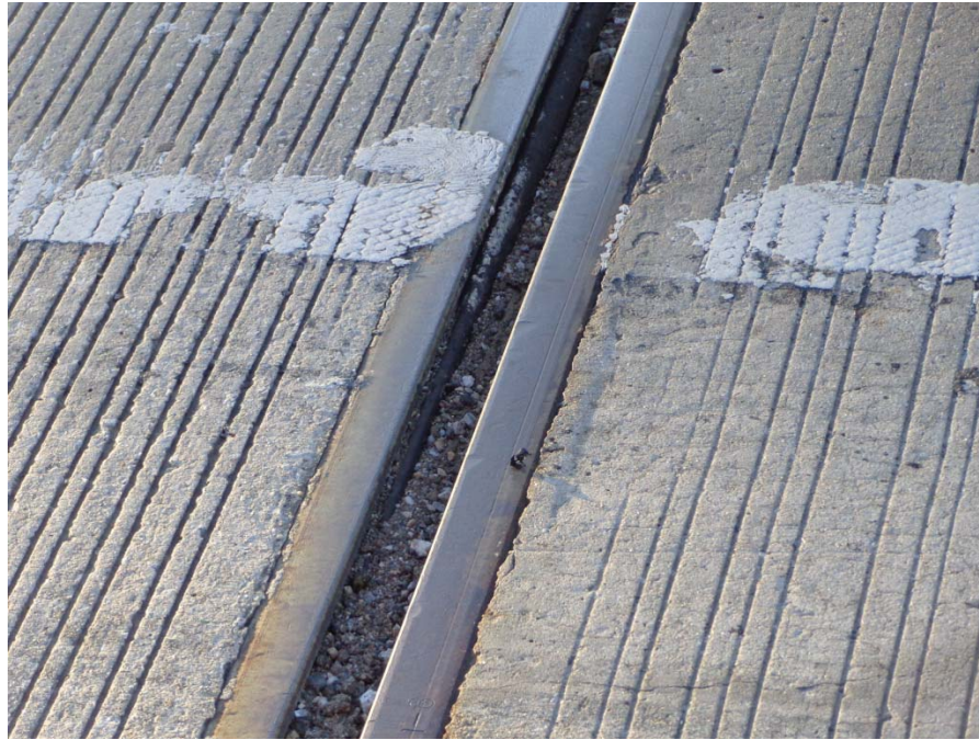
Figure 3: Joint View from Deck (End Bent 1)
