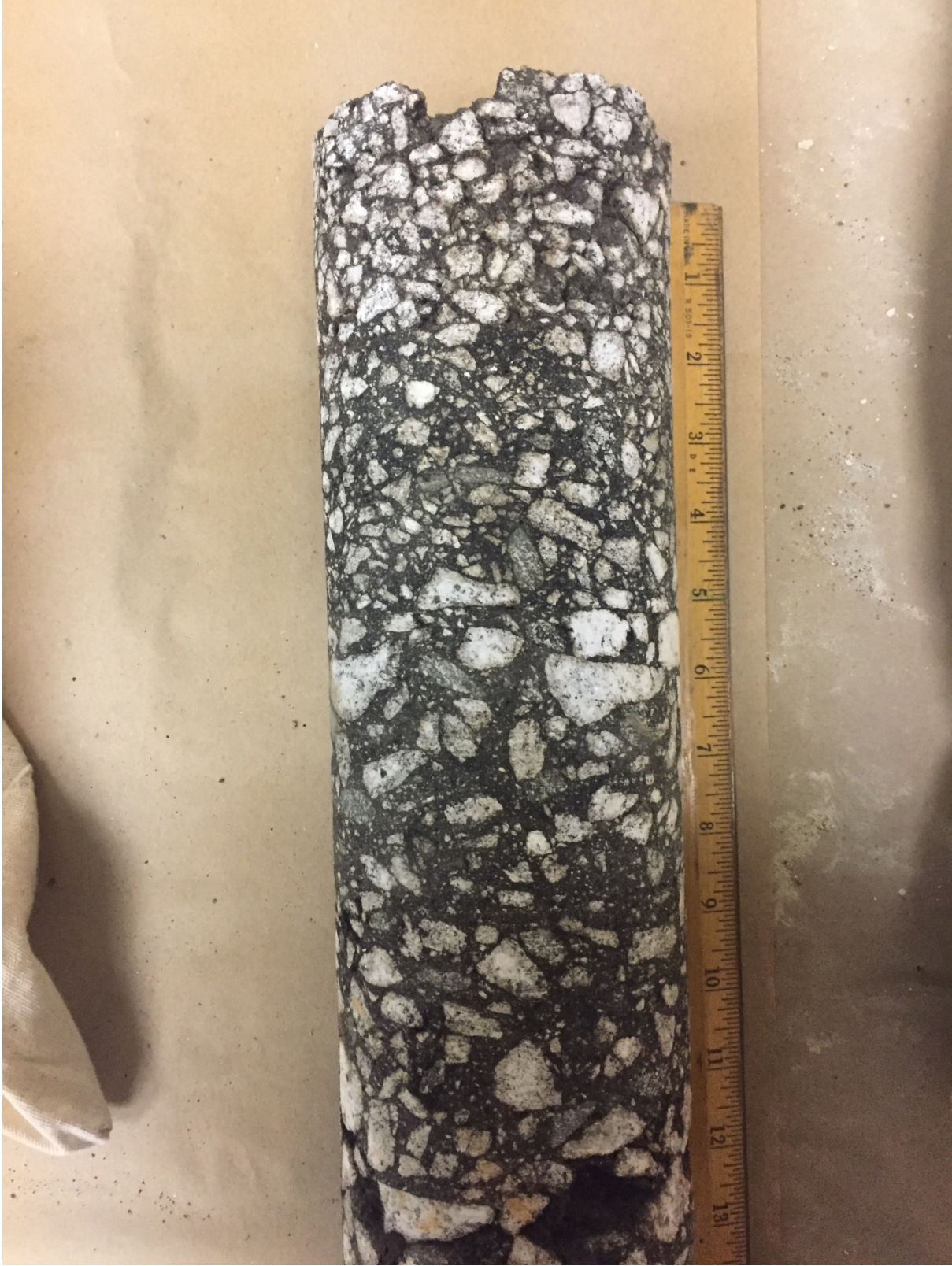
SC-5 N Mountain Street (South of I-85 – Outside Lane)
