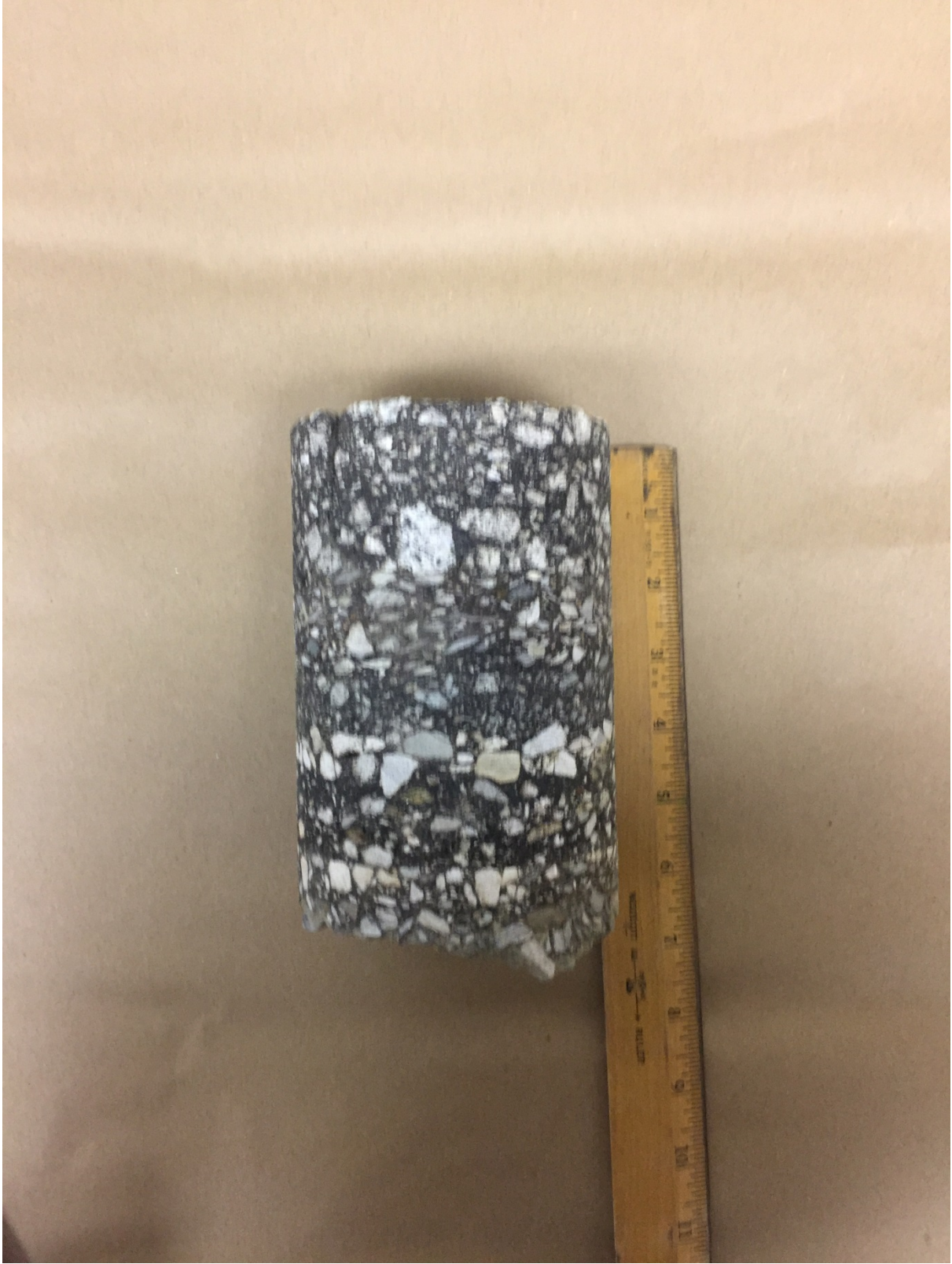
US 29 ( South of I-85 prior to Lakeview Drive)
