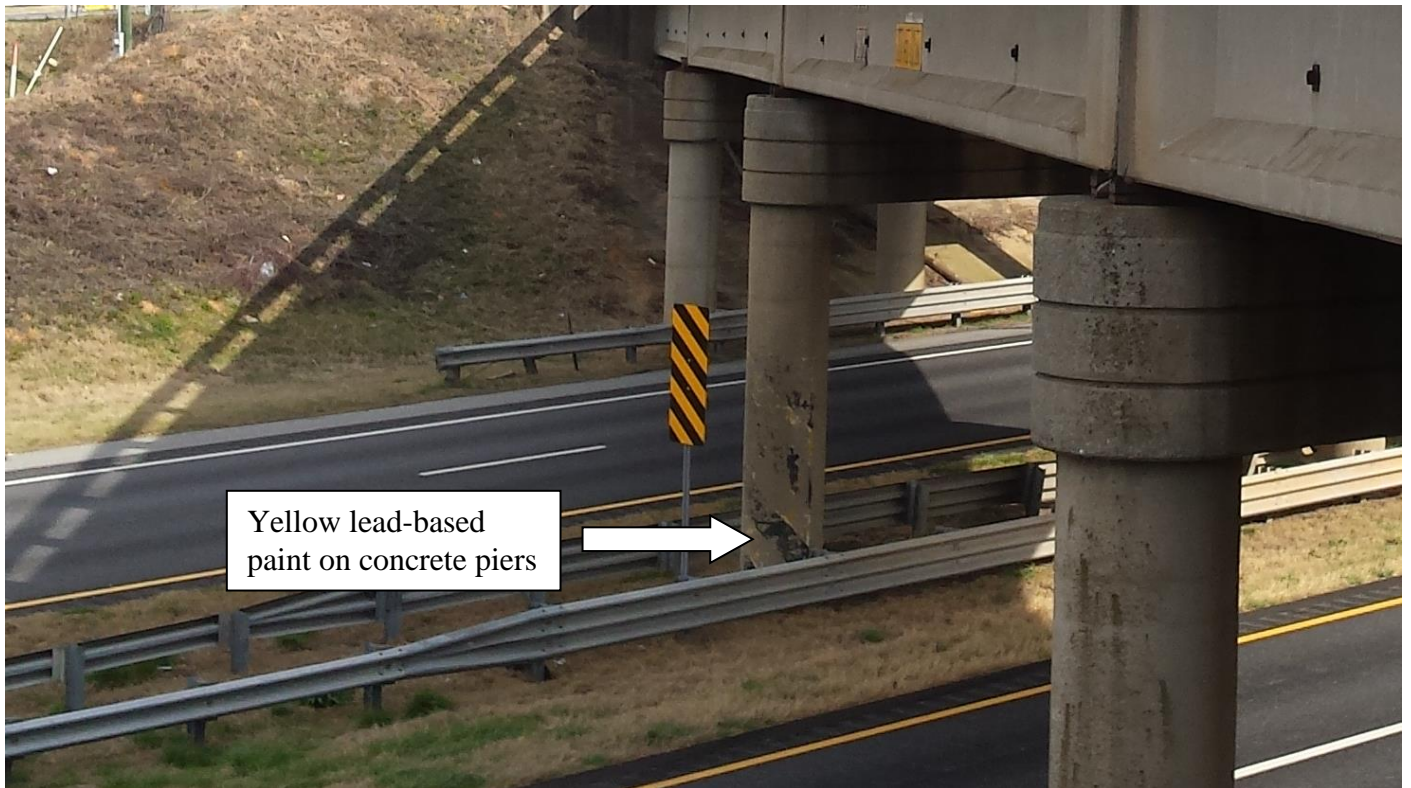
Photograph 6 – View of the side of the bridge showing the yellow paint on the concrete piers that tested positive for lead-based paint.
