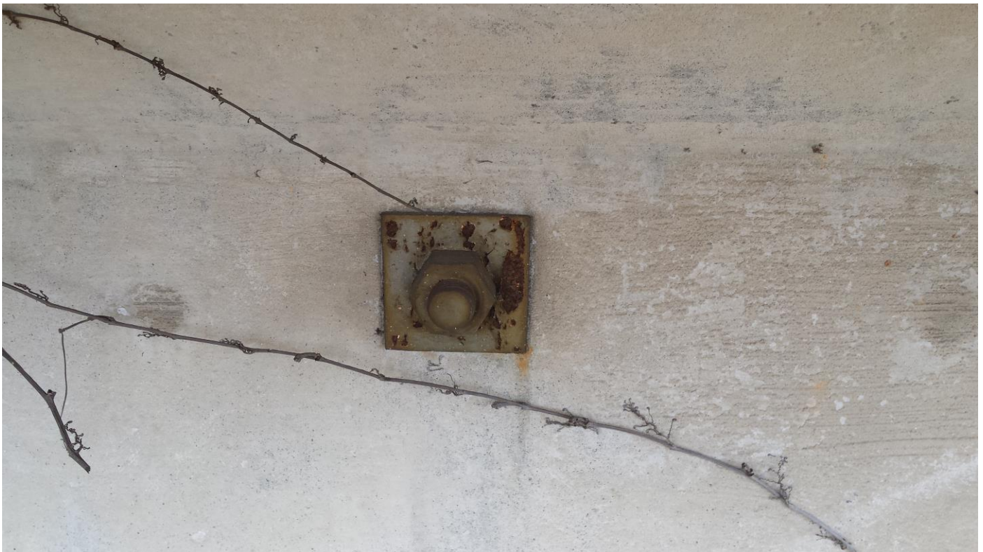
Photograph 4 – View of the metal bridge plates and bolts that tested positive for lead-based paint.
