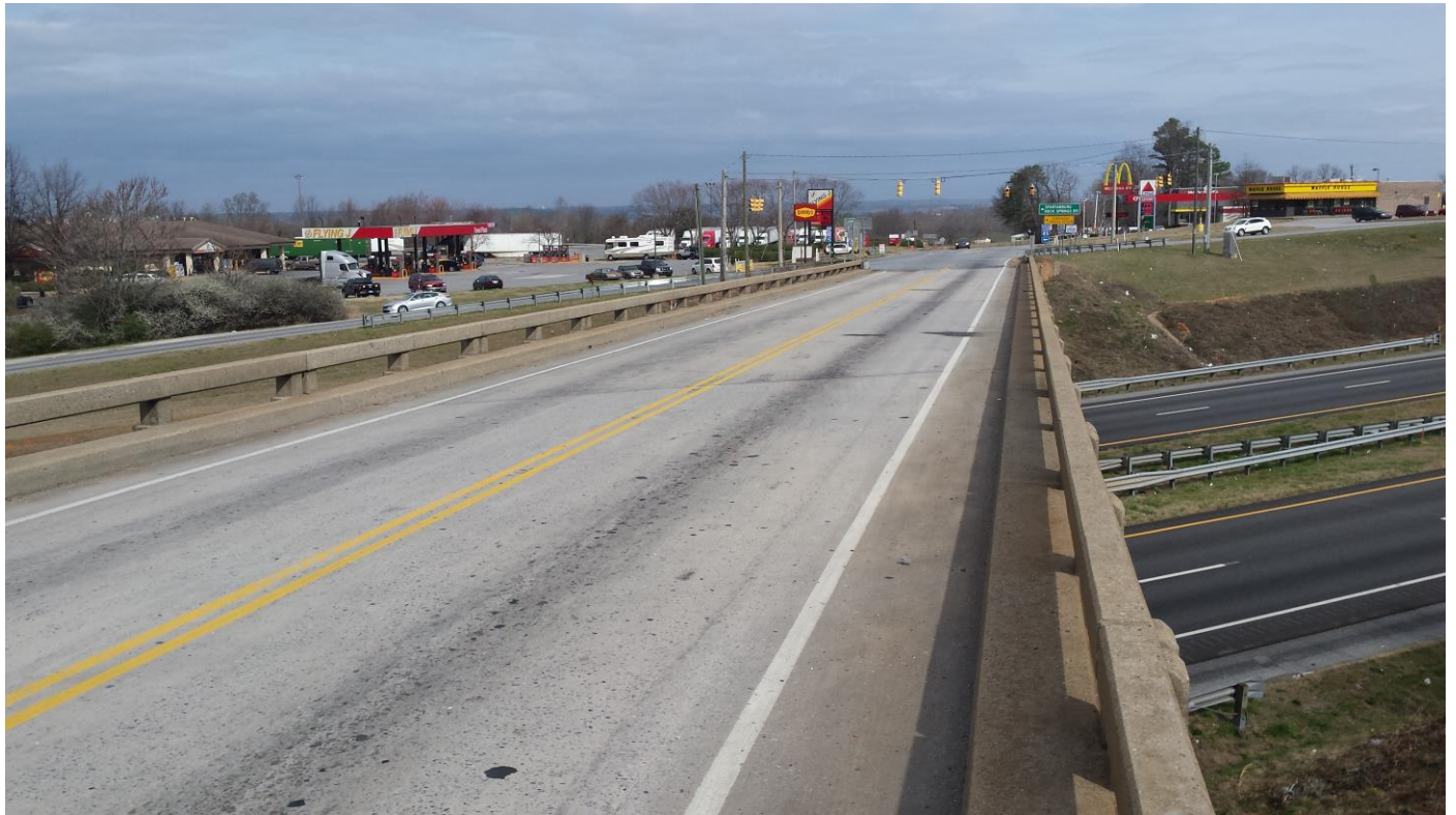
Photograph 2 – View of the top of the bridge at the SC 5/198 (North Mountain Street) Bridge over I-85 at Exit 102 in Cherokee County, South Carolina.
