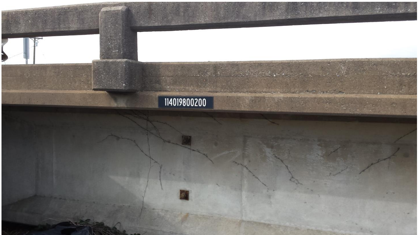
Photograph 1 – View of the bridge structure number at the SC 5/198 (North Mountain Street) Bridge over I-85 at Exit 102 in Cherokee County, South Carolina.
