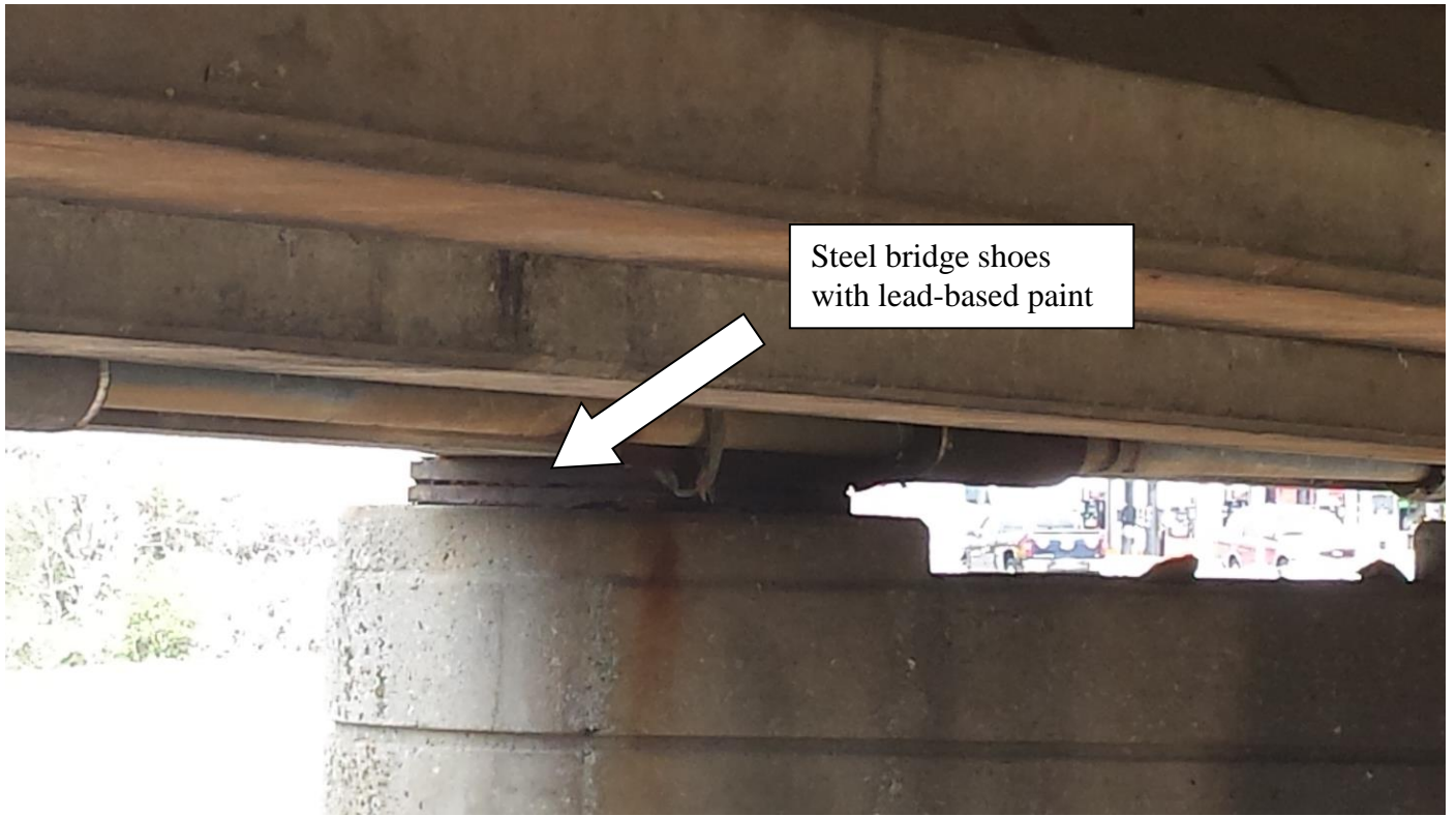
Photograph 5 – View underneath the bridge showing the steel bridge shoes between the concrete pier caps and the concrete deck that tested positive for lead-based paint.
