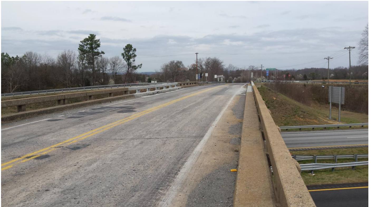
Photograph 2 – View of the top of the bridge structure at the S-11-99 (Tribal Road) Bridge over I-85 in Cherokee County, South Carolina.
