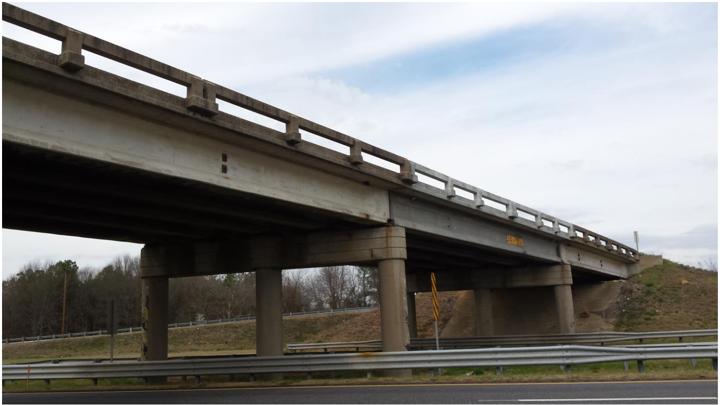
Photograph 3 –View of the side of the S-11-99 (Tribal Road) Bridge over I-85 in Cherokee County, South Carolina.
