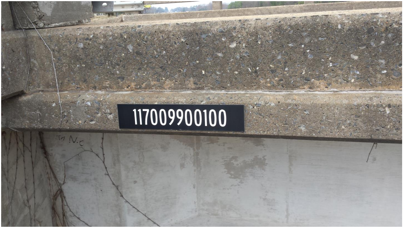
Photograph 1 – View of the bridge structure number at the S-11-99 (Tribal Road) Bridge over I-85 in Cherokee County, South Carolina.
