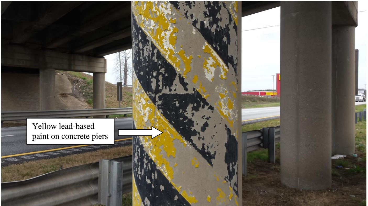
Photograph 6 – View of the yellow paint on the concrete piers that tested positive for lead-based paint.
