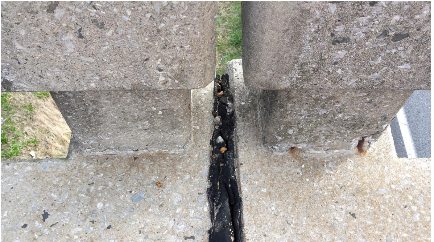
Photograph 4 – View of the black expansion joint material between concrete deck sections that was tested for asbestos.
