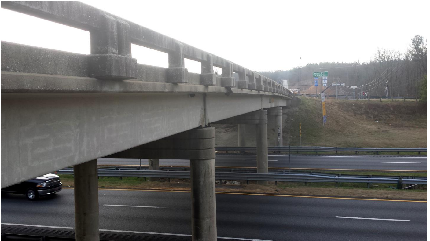
Photograph 3 – View of the side of the S-11-83 (Blacksburg Highway) bridge over I-85 in Cherokee County, SC.
