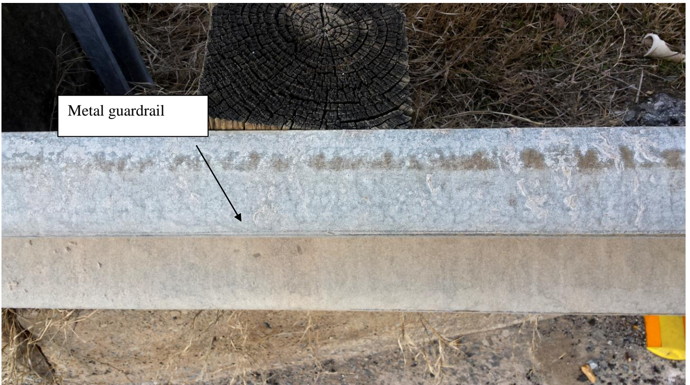
Photograph 6 – View of the metal guardrail that was tested for lead-based paint.
