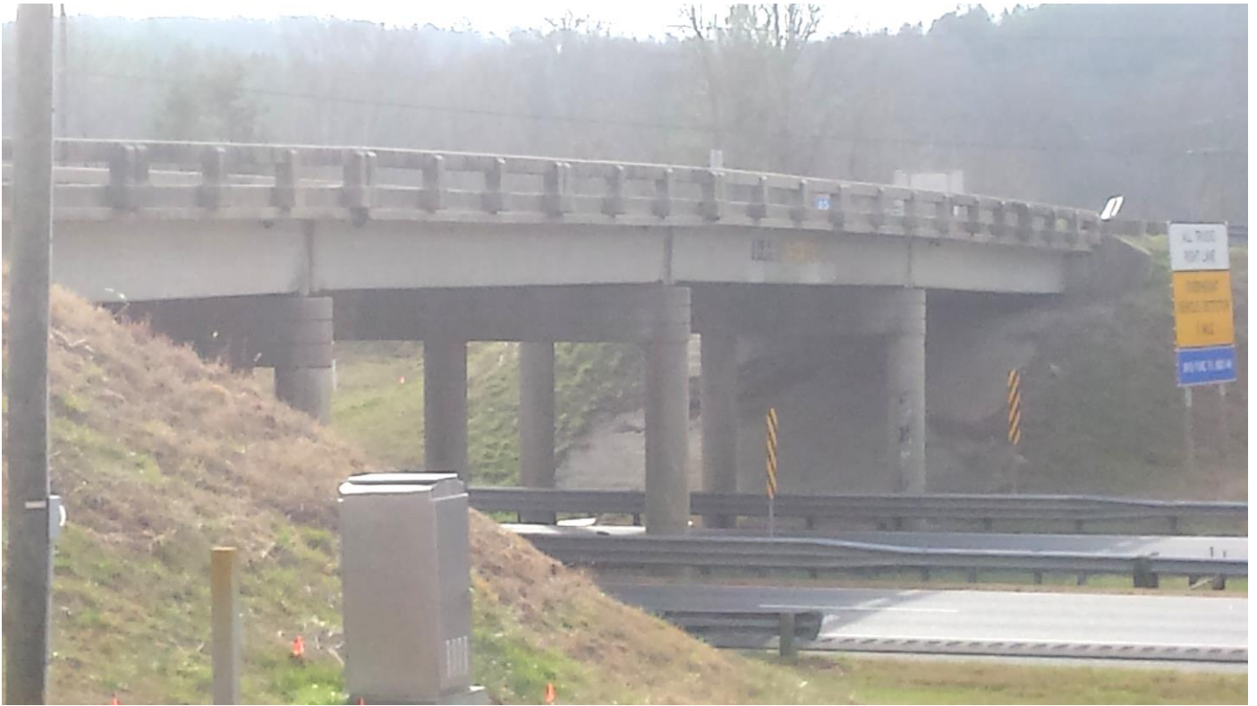
Photograph 1 – View of bridge structure at S-11-83 (Blacksburg Highway) over I-85 in Cherokee County, SC.
