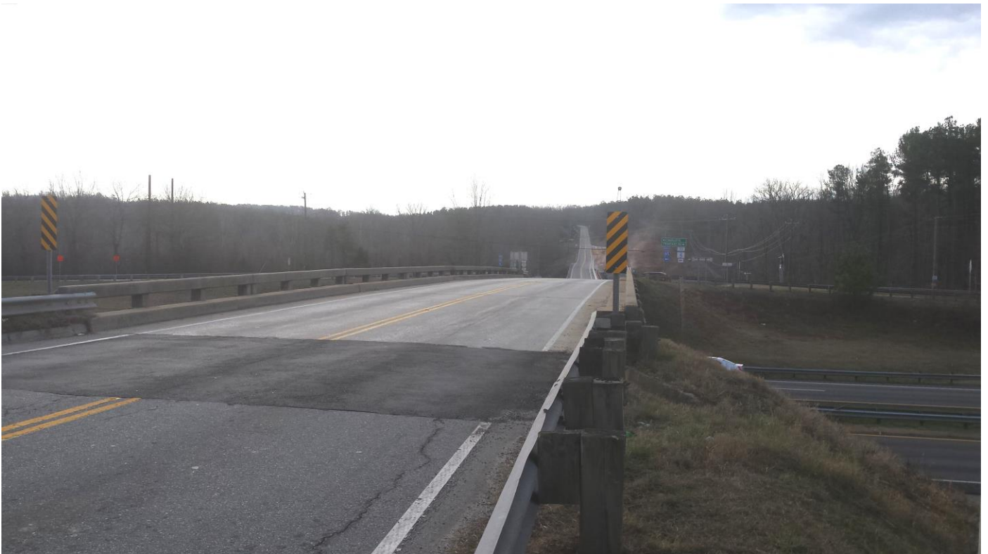
Photograph 2 –View of the top side of the S-11-83 (Blacksburg Highway) bridge over I-85 in Cherokee County, SC.
