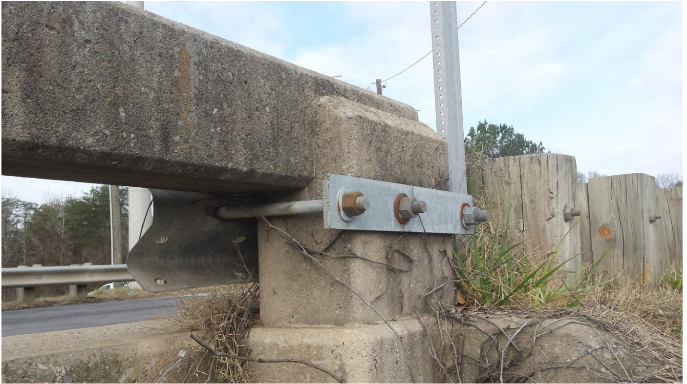
Photograph 5 – View of the metal and wood guardrails on the side of the S-11-83 Bridge at Exit 100 that were tested for lead-based paint.
