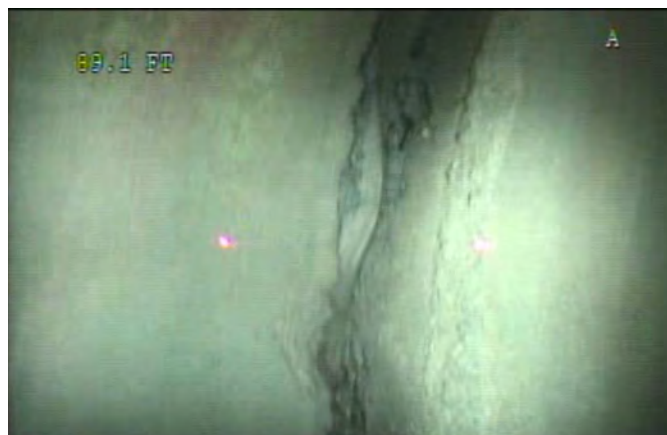
Joint - Separated at 89 ft
