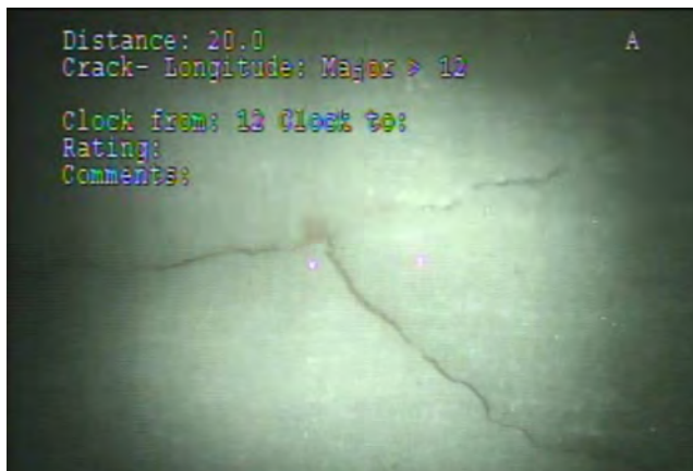
Longitudinal crack at 20 ft
