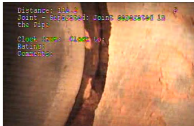
Joint - Separated at 112 ft
