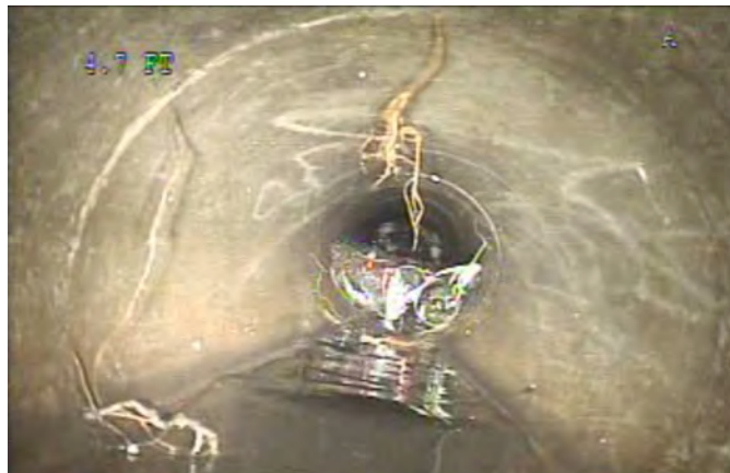
Root in joint at 6 ft; Debris ahead
