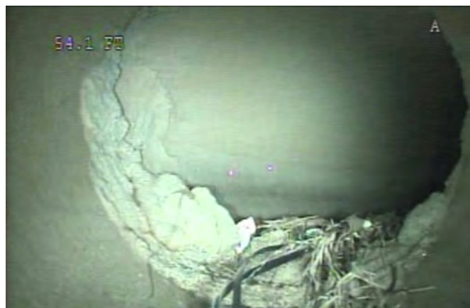
Joint - Separated and Joint - Angular at 58 ft
