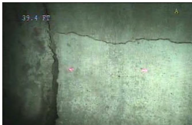
Joint - Separated and Multidirectional crack at 40 ft
