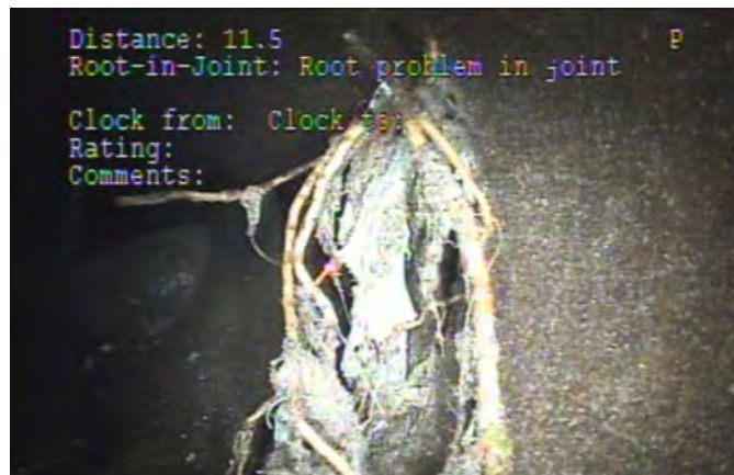
Root in joint at 12 ft
