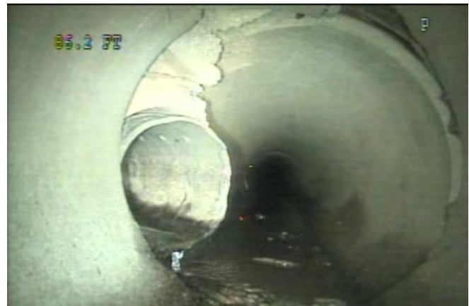
Collapsed at 88 with lateral pipe
