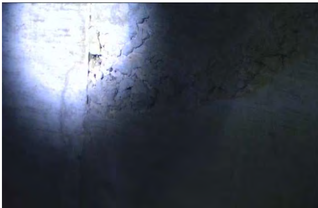
Typical chipping/scaling
