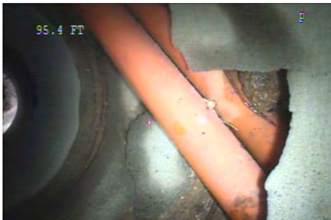
Thru pipe at 95 ft
