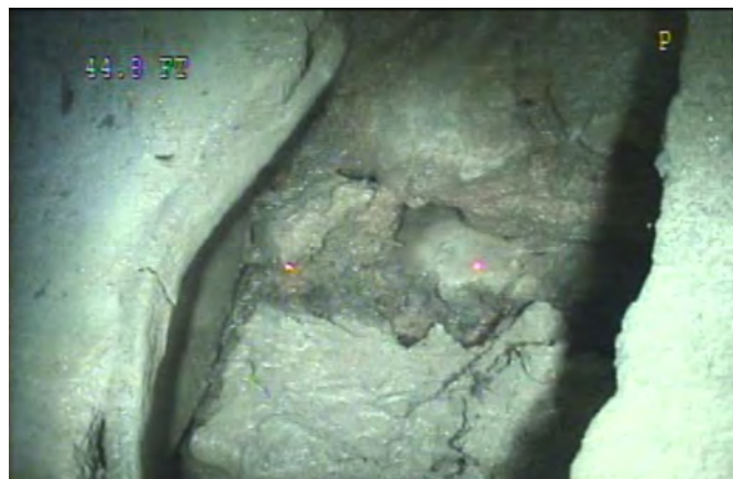
Broken at 45 ft
