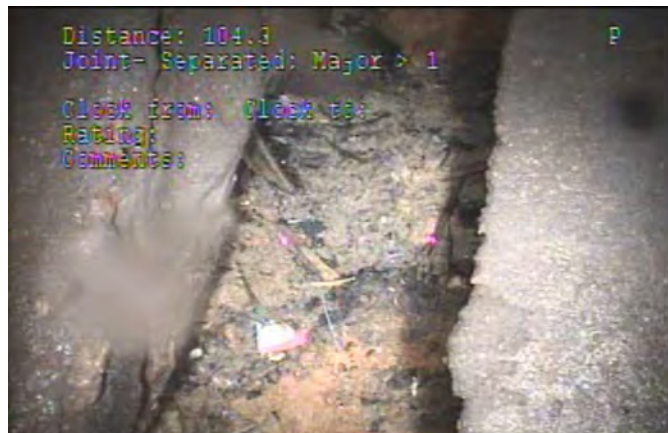
Joint - Separated at 104 ft
