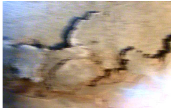
Typical cracking/chipping along side
