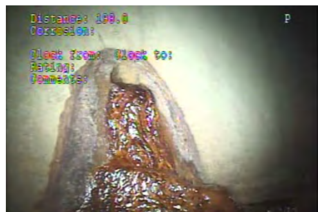
Corrosion at 198 ft
