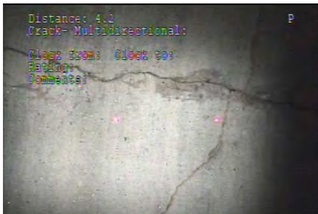
Multidirectional crack at 4 ft
