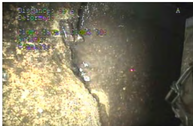
Deformed at end adjacent to junction box
