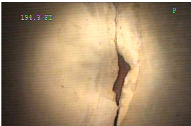
Joint - Separated at 11 ft
