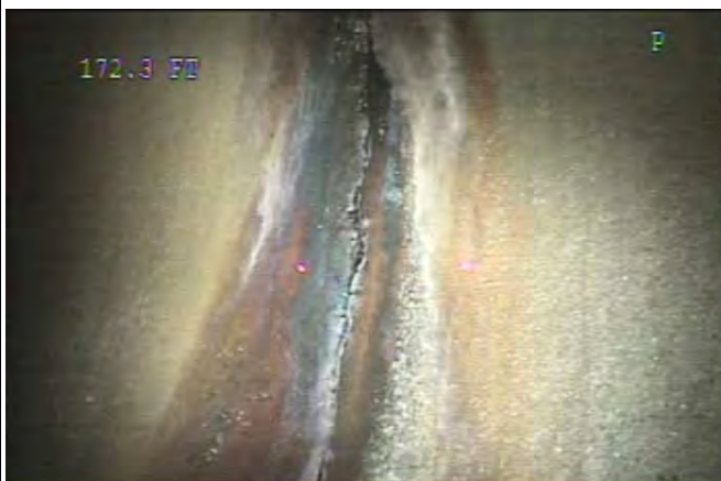
Joint - Alignment at 172 ft
