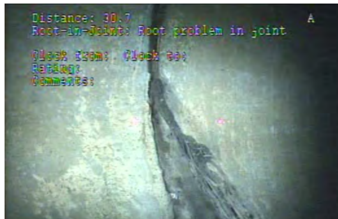
Root in joint at 31 ft
