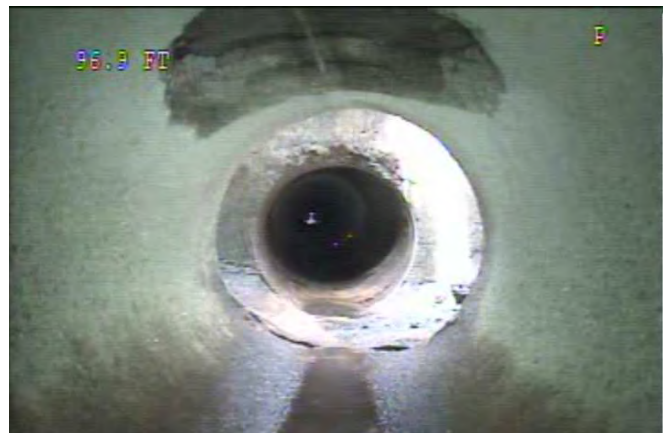
Broken (above) at 100 ft
