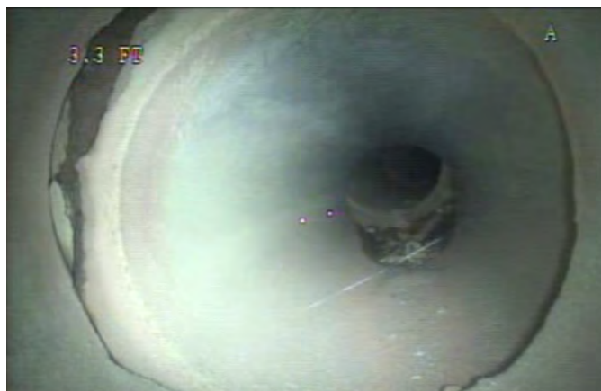
Pipe not connected at 6 ft; All joints major offset as far as camera will zoom
