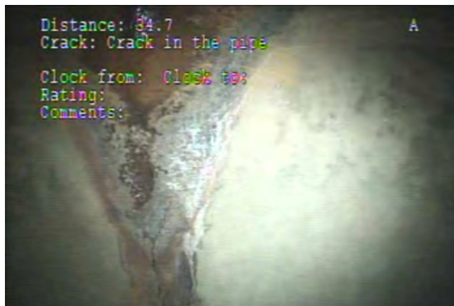
Crack at 35 Ft
