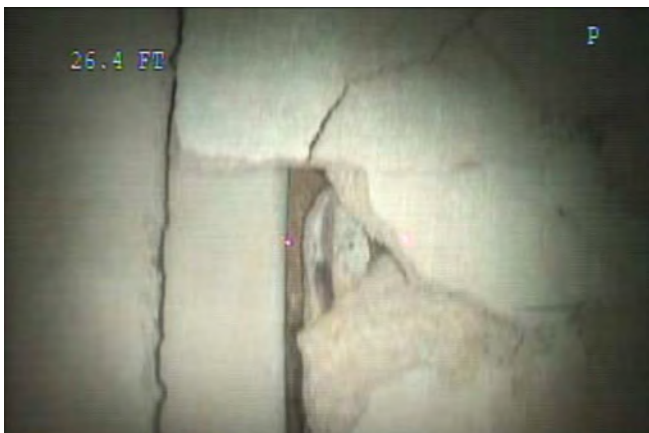
Joint - Separated and Multidirectional crack at 26 ft
