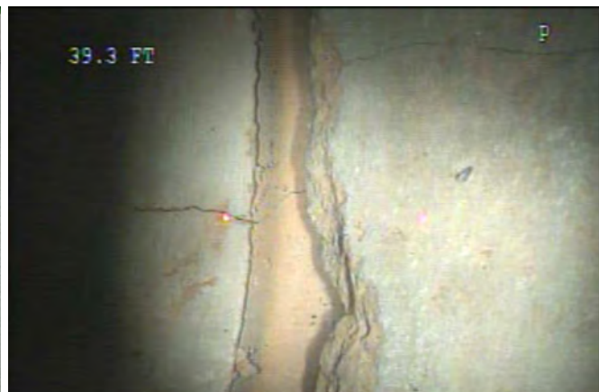
Joint - Separated and crack at 39 ft
