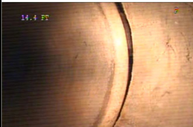
Joint - Separated and cracked at 14 ft
