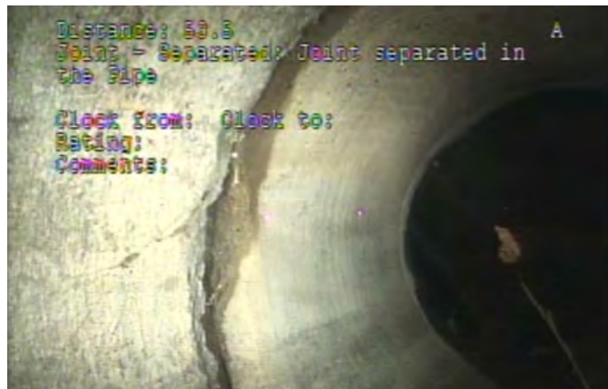
Joint - Separated at 53 ft
