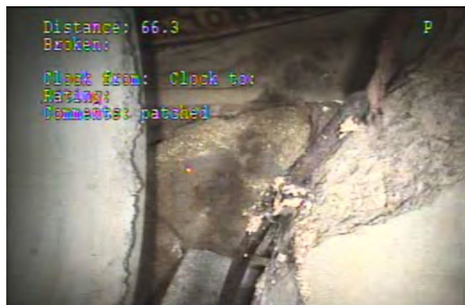
Broken at 66 ft
