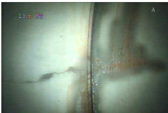
Crack at 14 ft (runs for 63 ft length)
