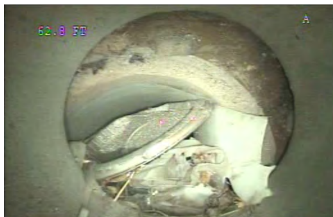
Broken at 65 ft
