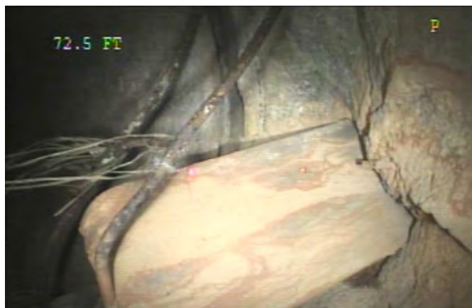
Guardrail post driven through pipe at 73 ft
