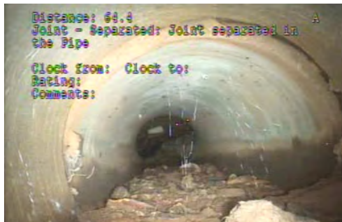
Joint - Separated at 64 ft
