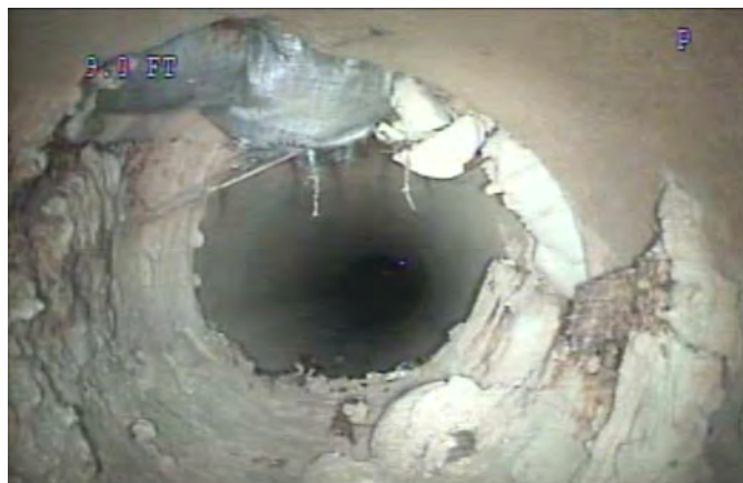
Broken at 9 ft
