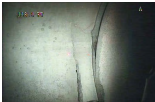
Joint Offset and chipped at 118 ft
