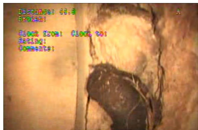
Broken at 37 ft (left) and 45 ft (right)
