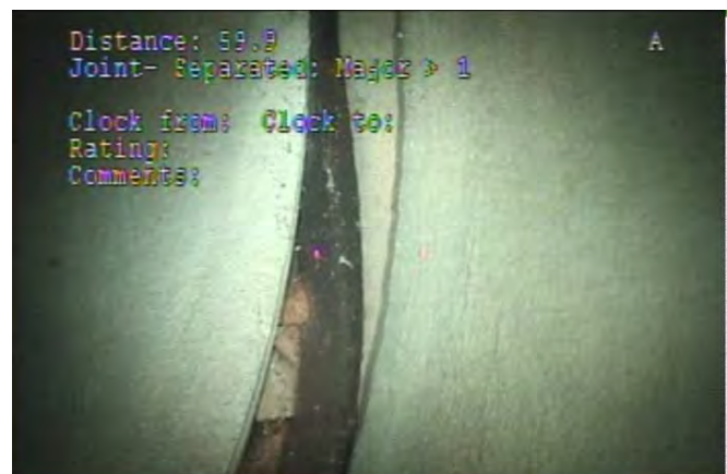
Joint - Separated at 53 ft (left) and 60 ft (right)
