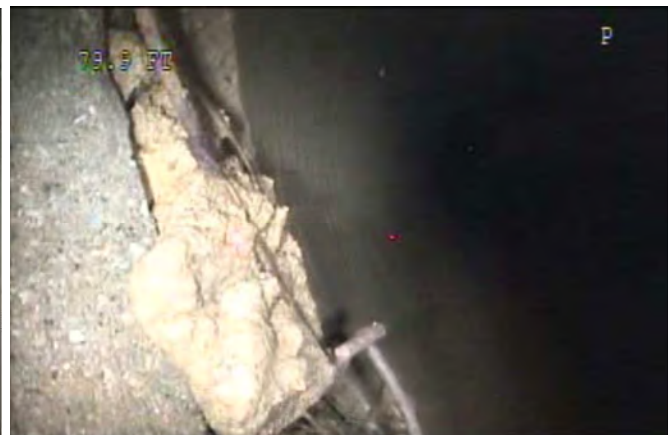
Joint - Separated at 80 ft
