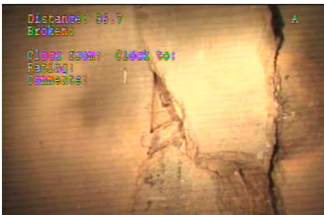
Broken at 37 ft (left) and 45 ft (right)
