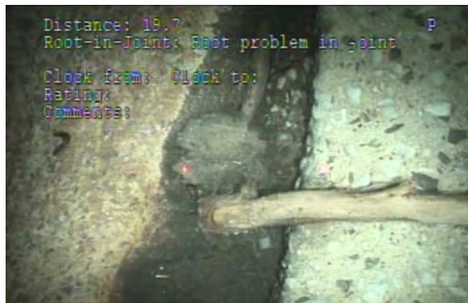
Root in joint at 19 ft
