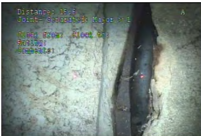
Joint - Separated at 16 ft
