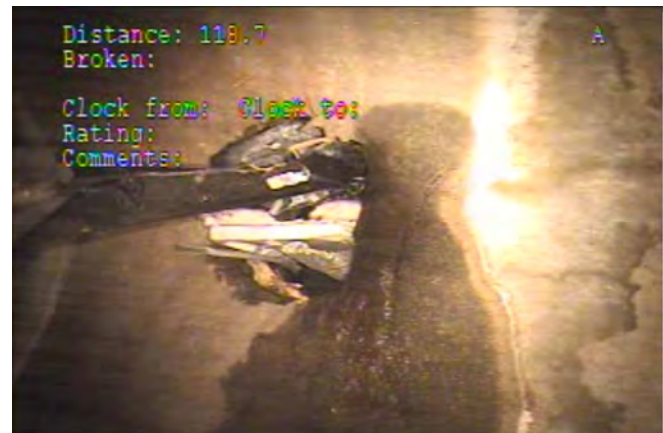
Broken at 119 ft
