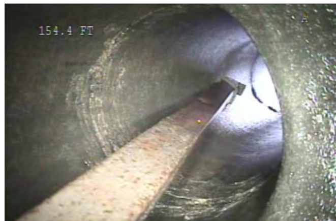
Debris at 154 ft (Left: looking ahead; Right: looking up)
