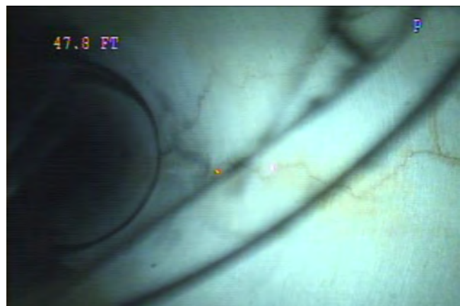
Multidirectional crack at 48 ft
