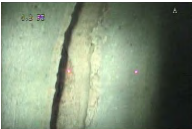
Joint - Separated at 4 ft
