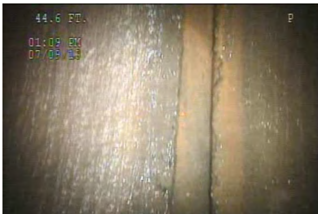
Joint - Separated at 45 ft
