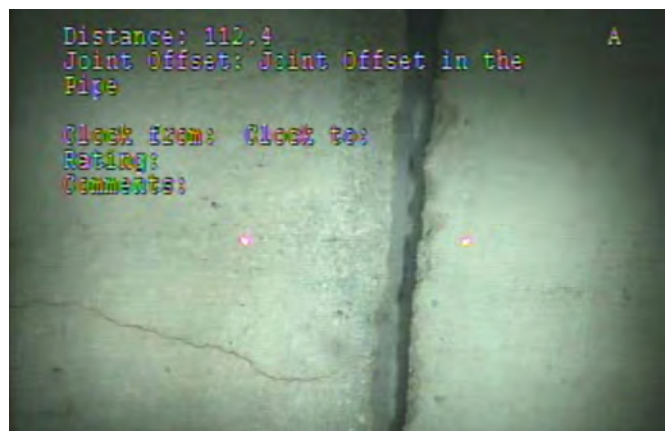
Joint Offset and longitudinal crack at 112 ft; other offset and cracks similar
