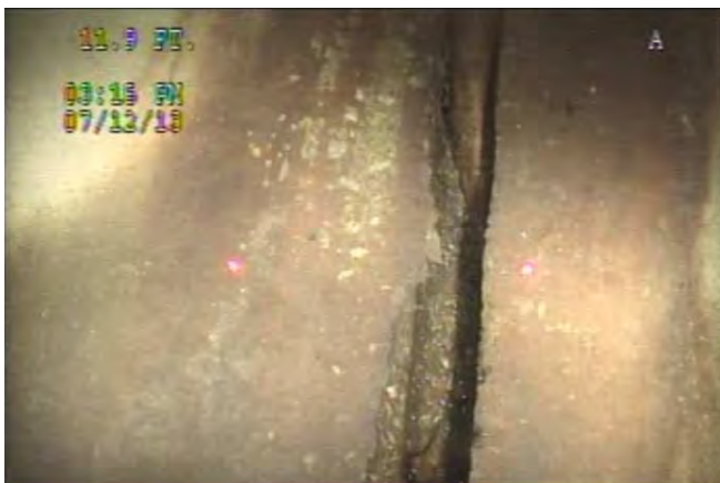
Joint - Separated at 12 ft
