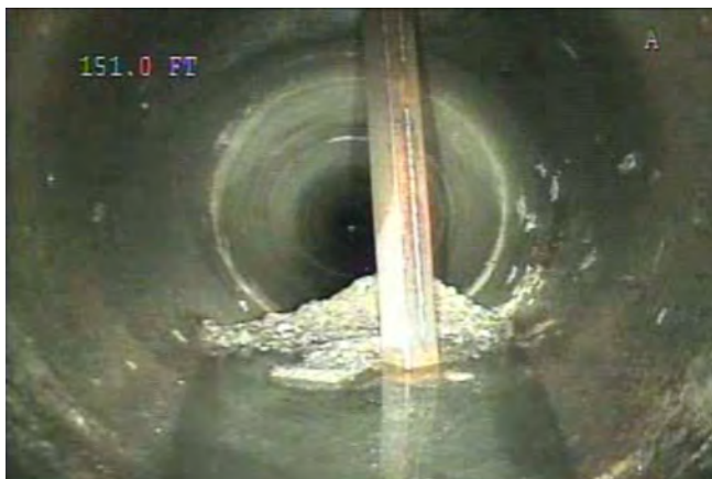
Debris at 154 ft (Left: looking ahead; Right: looking up)
