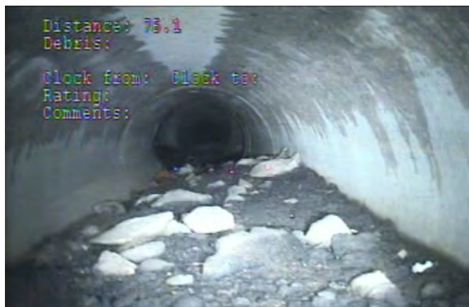
Debris at 75 ft
