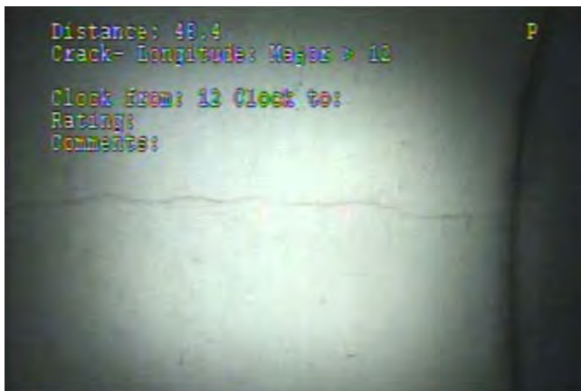
50-ft long. crack at 48 ft; other cracks similar
