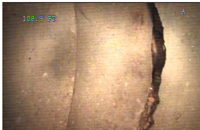
Joint - Separated at 109 ft
