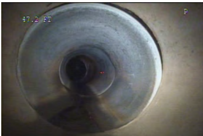
Joint - Separated at 53 ft (left) and 60 ft (right)
