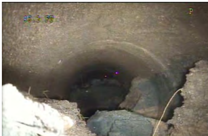
Debris at 46 ft
