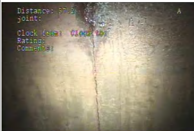
Joint issues/deformed at 37 ft
