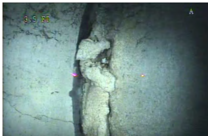
Joint - Separated at 4 ft
