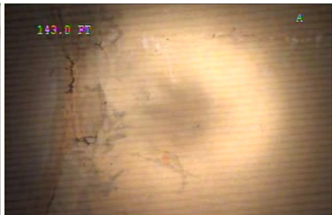
Joint - Separated and cracked at 42 ft (left) and 143 ft (right)
