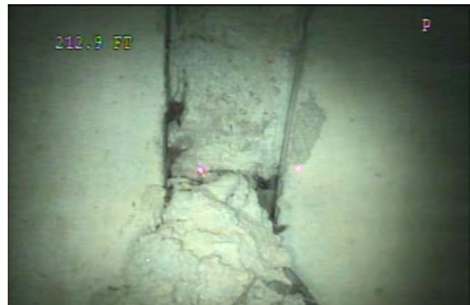
Joint - Separated at 213 ft
