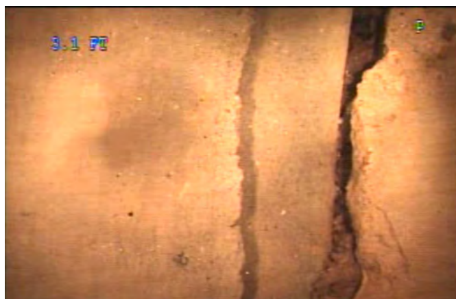
Joint - Separated at 3 ft
