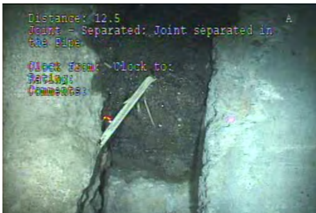
Joint - Separated at 13 ft
