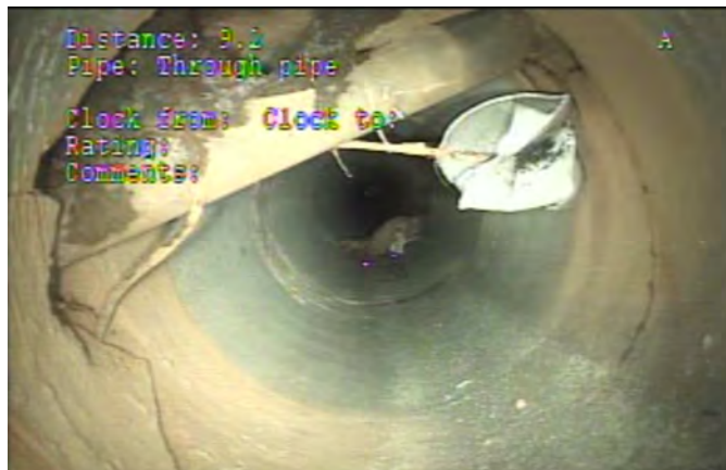
Utility conduit through pipe at 9 ft
