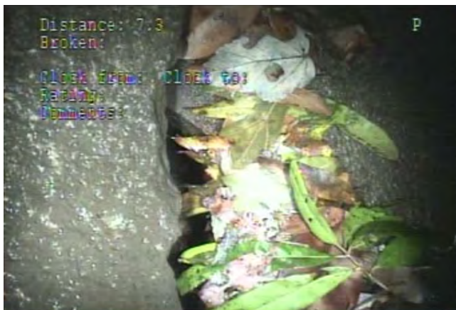
Broken at 7 ft
