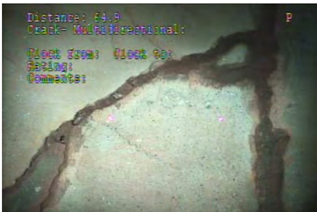
Multidirectional crack at 65 ft
