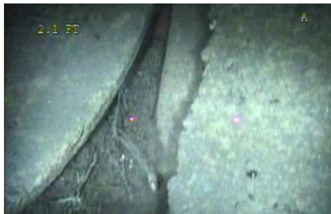
Joint - Separated at 2 ft
