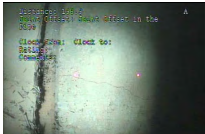
Joint Offset and crack at 138 ft
