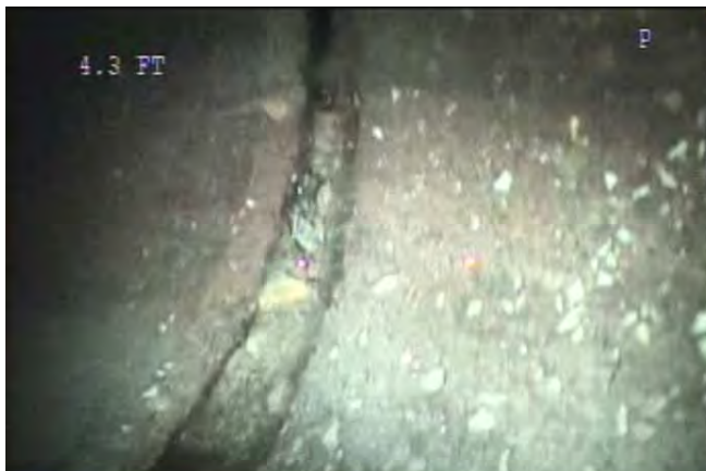
Joint - Separated at 4 ft (left) and 17 ft (right); other joint separations similar
