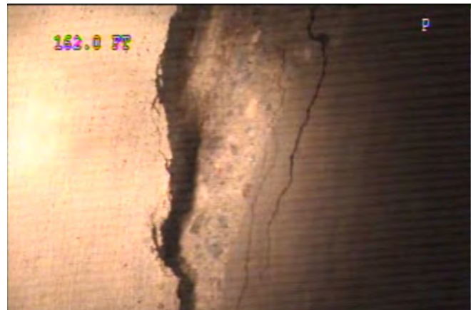
Joint - Separated and cracked at 162 ft
