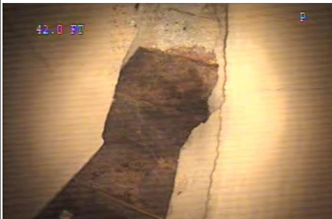
Joint - Separated and cracked at 42 ft (left) and 143 ft (right)
