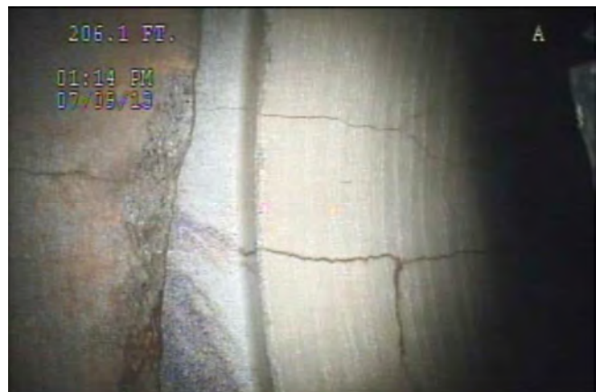
Crack at 206 ft
