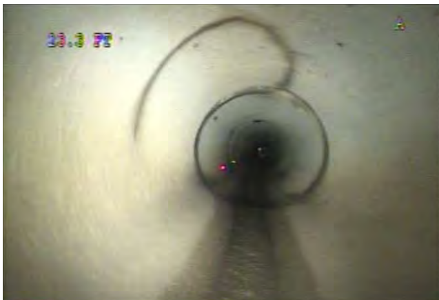
Cracks at 27 ft (left) and 127 ft (right)
