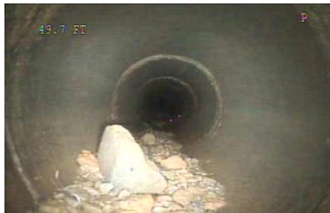
Debris at 50 ft
