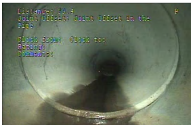
Joint Offset at 59 ft; other Joint Offset issues similar
