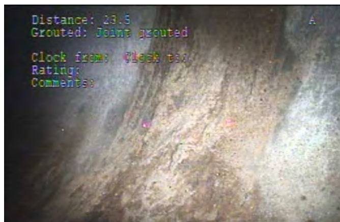
Grouted at 24 ft
