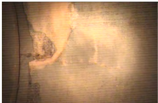
Joint Offset and crack at 404 ft
