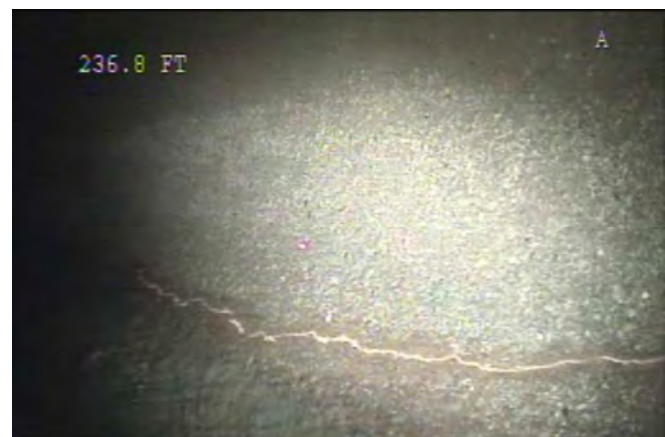
Longitudinal crack at 237 ft
