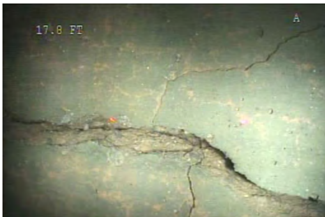
Broken at 18 ft
