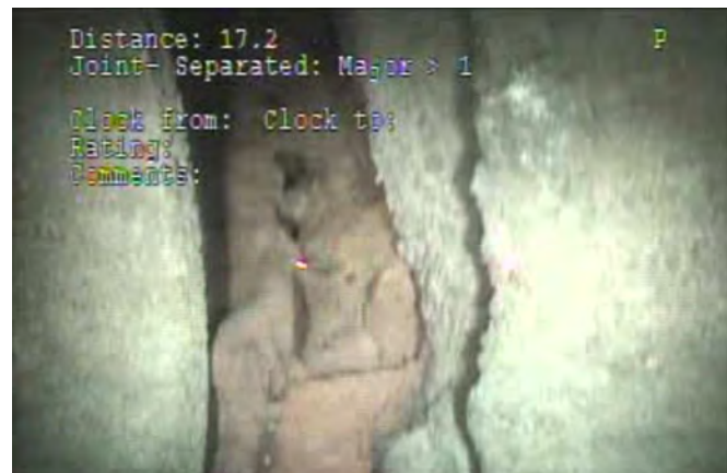
Joint - Separated at 4 ft (left) and 17 ft (right); other joint separations similar
