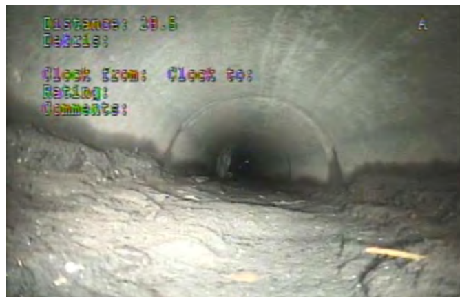
Debris at 29 ft
