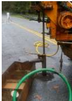
Photo 1. Drill rig at STB-1 (S-21-57)
