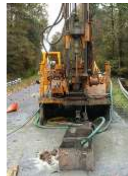
Photo 2. Drill rig at STB-2 (S-21-57)
