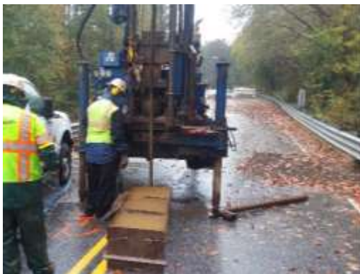
Photo 1. Drill rig at STB-1 (S-20-101)
