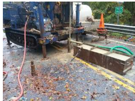
Photo 2. Drill rig at STB-2 (S-20-101)
