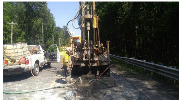
4. Photograph of rig on B-4
