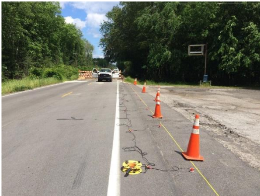
15. Photograph of MASW Array Dry Branch Bridge
