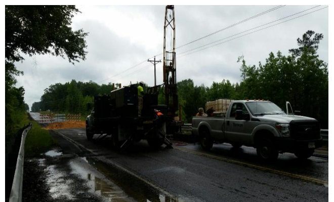
12. Photograph of rig on CPT-6
