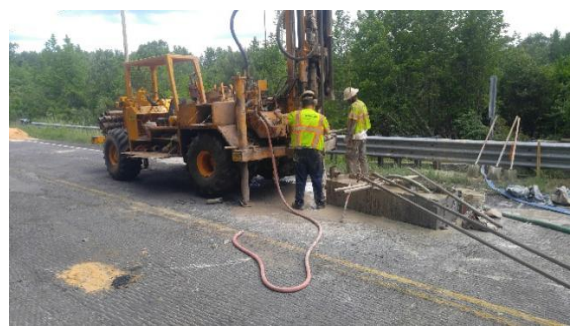
6. Photograph of rig on B-6
