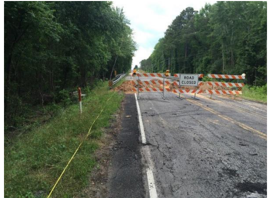
14. Photograph of MASW Array Cedar Branch Bridge
