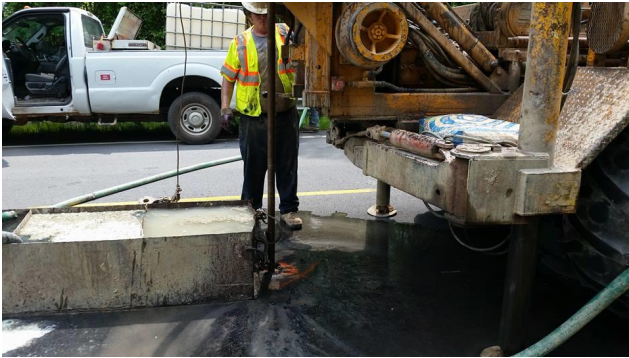
1. Photograph of rig on B-1
