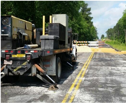
9. Photograph of rig on CPT-3
