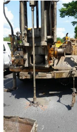
2. Photograph of rig on B-2
