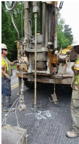
3. Photograph of rig on B-3
