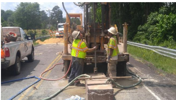
5. Photograph of rig on B-5
