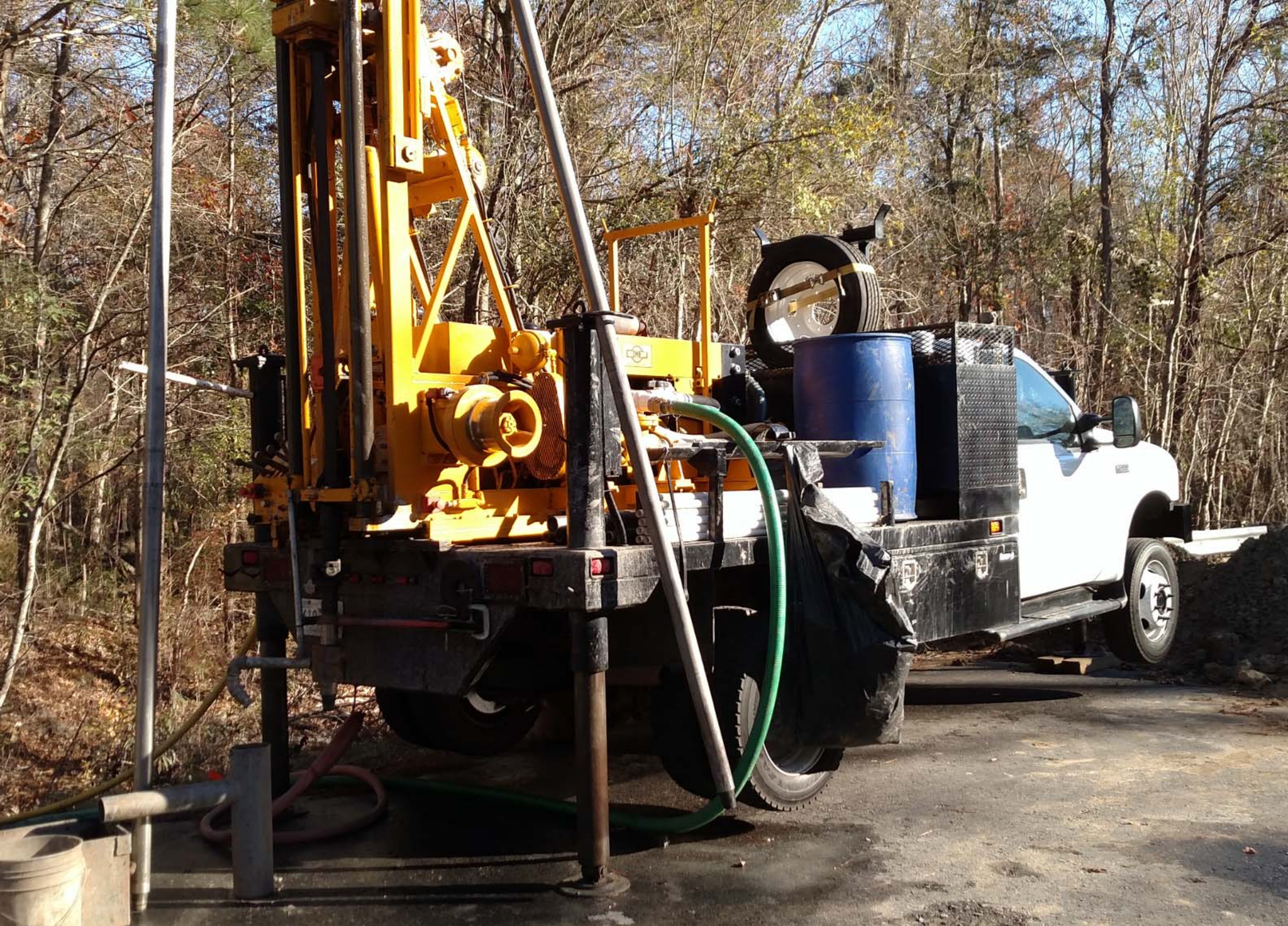
Figure No. 3: Photograph of Soil Test Boring STB-301 Being Drilled
