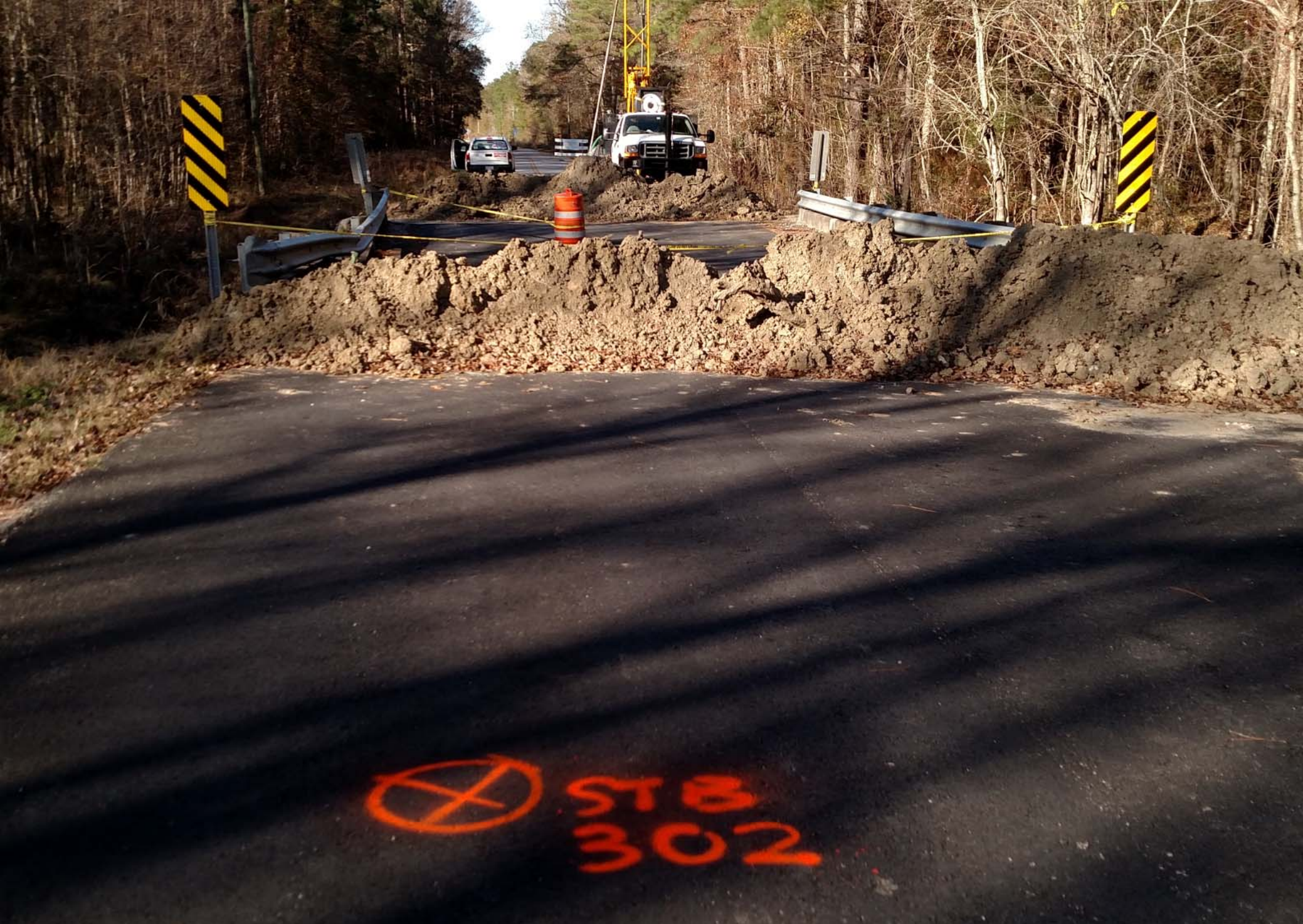
Figure No. 4: Photograph of Soil Test Boring STB-302
