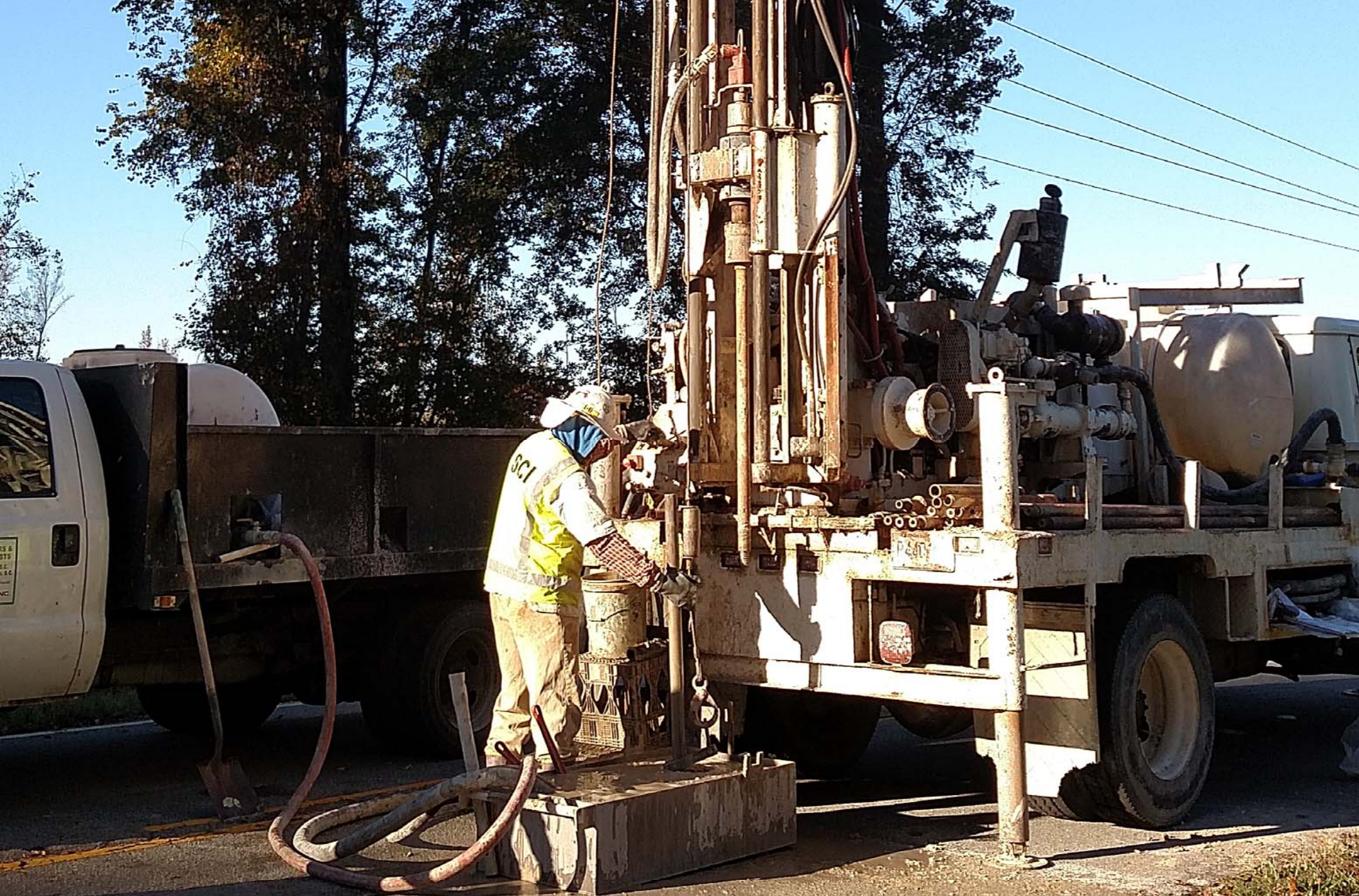
Figure No. 3C - Photograph of Boring B-03 Being Drilled
