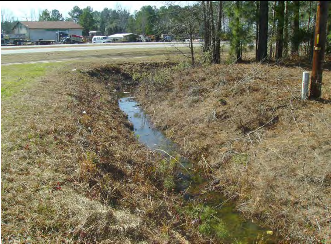
South view of Ditch D
