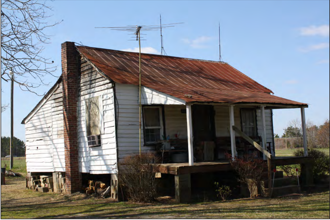
Figure 11. View of Resource 240, facing northwest.
