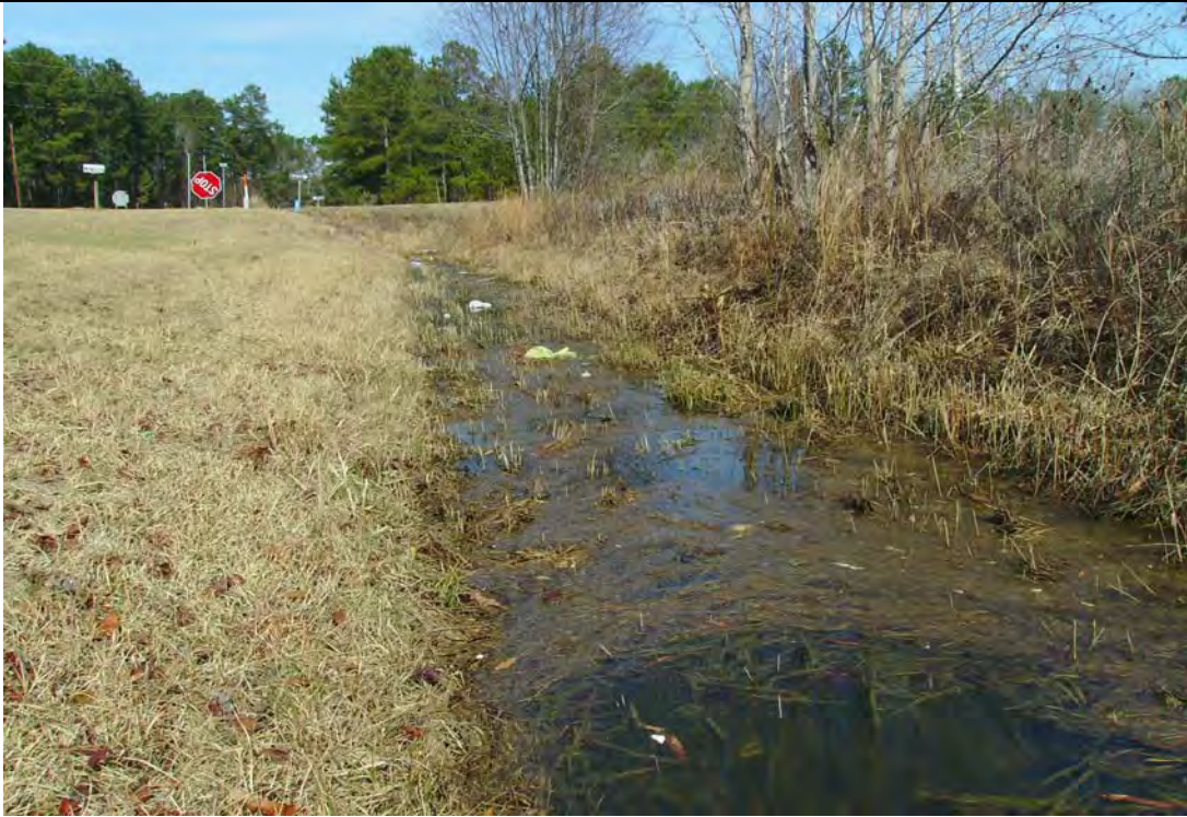
North view of Ditch E
