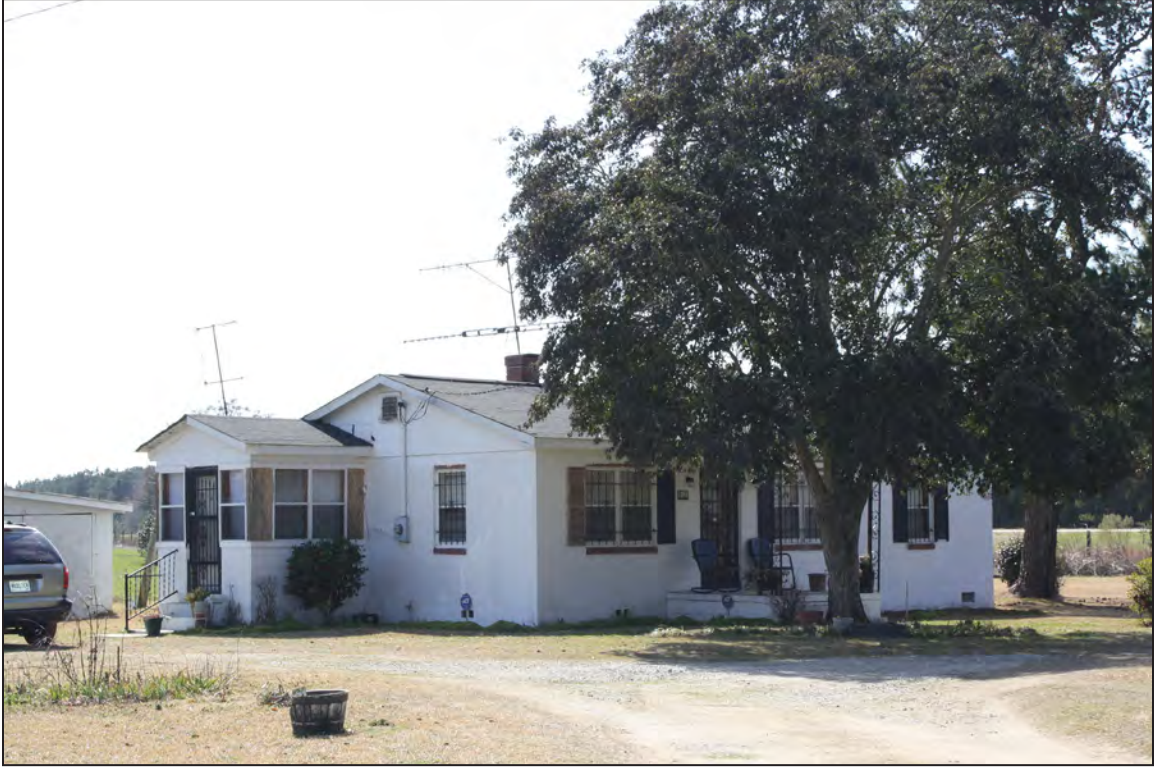
Figure 9. View of Resource 248, facing southwest.
