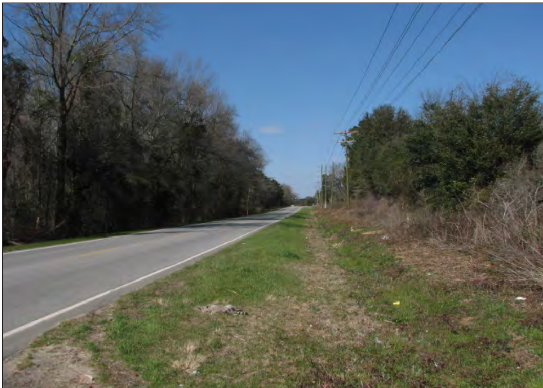
Figure 3. Typical views of the project area: view of US 301, looking east toward the I-95 overpass (top); view of project corridor along SC-6, looking north (bottom).
