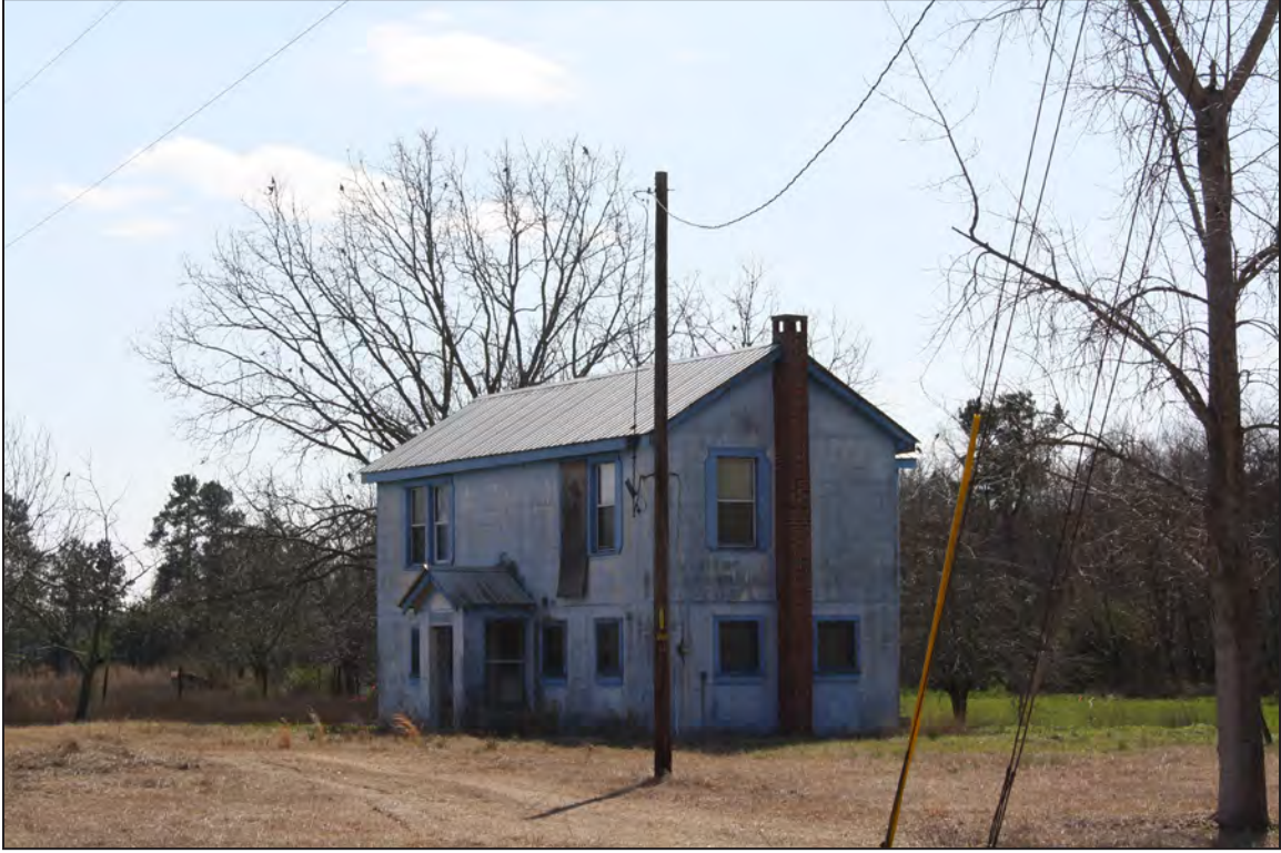
Figure 10. View of Resource 249, facing southwest.
