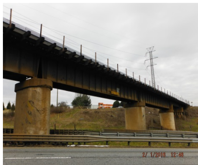
Photo 1 – CSX Railroad Bridge over I-85
