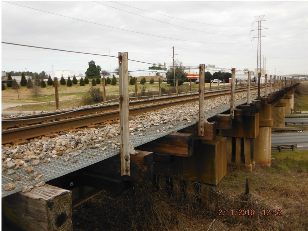
CSX Railroad Bridge over Interstate 85
