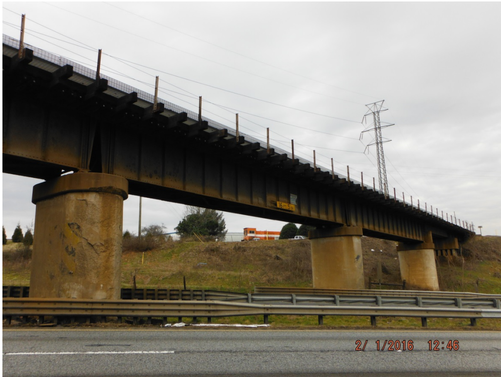
CSX Railroad Bridge over Interstate 85
