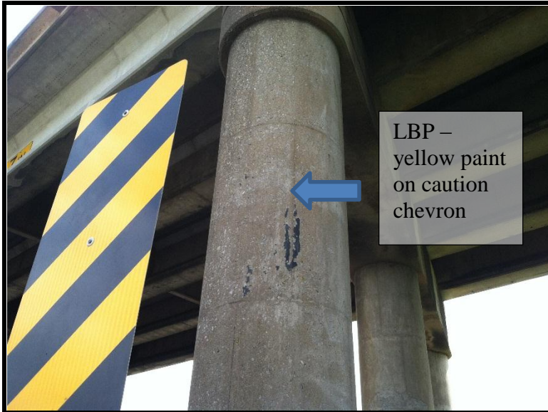
5 Lead sample from caution chevron on piers
