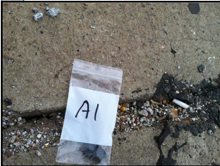
3 Tar expansion material on top deck Sample A -
