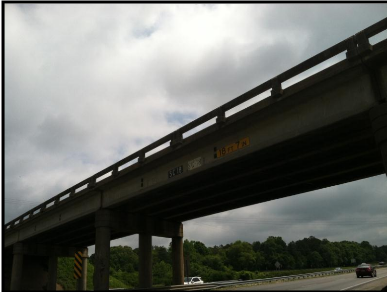
1 Bridge SC-18 on Shelby Road over I-85 General view from I-85
