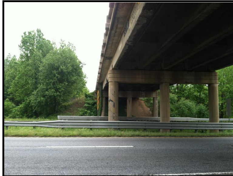
2 General view from I-85
