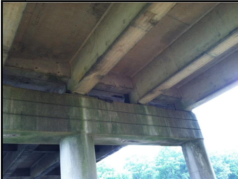
7 Concrete support and concrete decking
