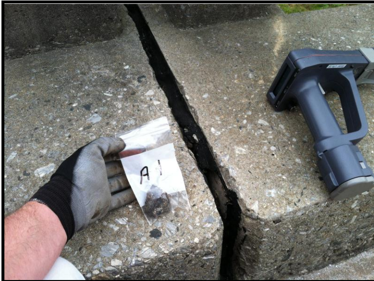
5 Tar expansion material located on top deck expansion joints Sample A -
