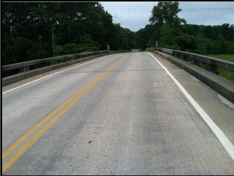
3 General view top deck
