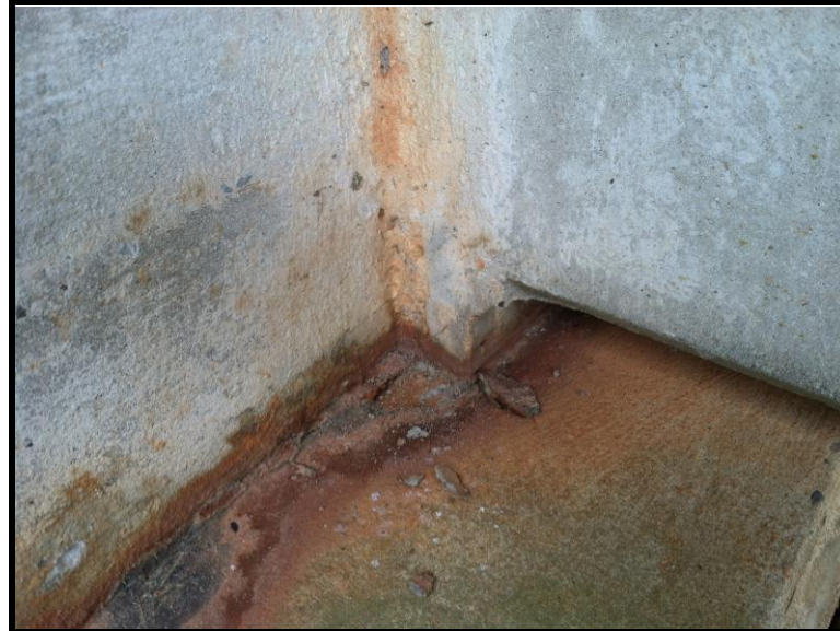
4 No bearing pads noted at back wall abutment
