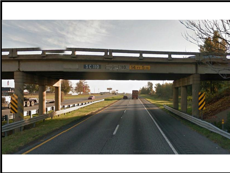
1 Bridge SC 110 on Battleground Road over I-85
