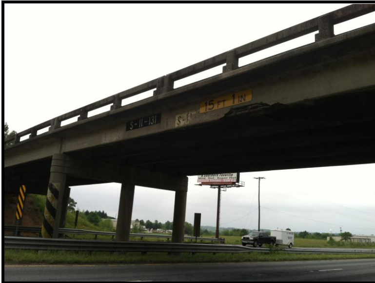
1 Bridge S-11-131 on Sunny Slope Drive over I-85 General view from I-85
