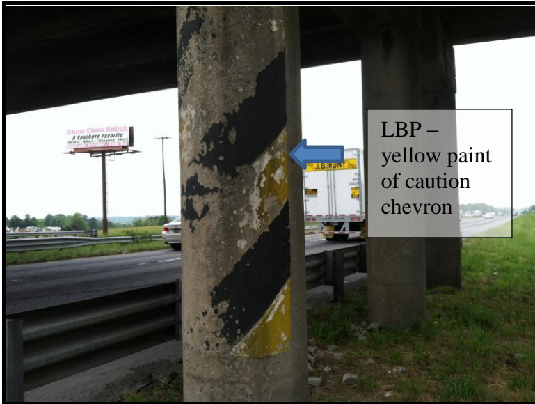
5 Lead sample from caution chevron on piers.
