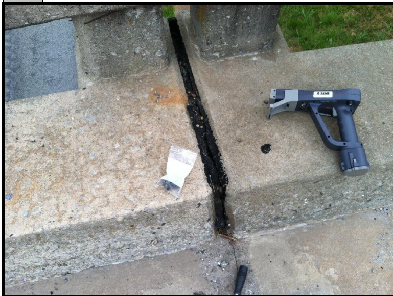
3 Tar expansion material located on top deck expansion joints Sample A -
