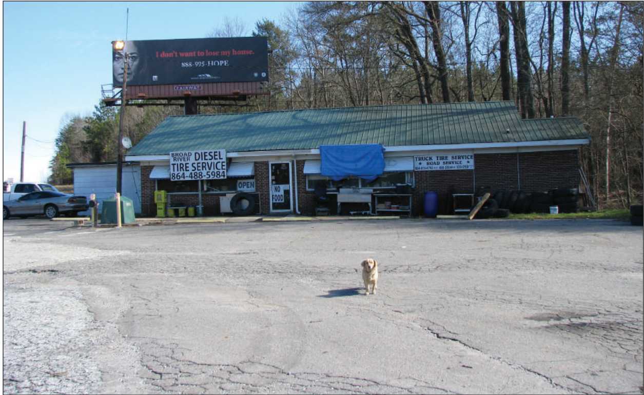
A. Restaurant (U/21/0247), View to East
