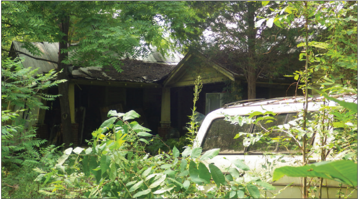
B. Detail of Porch, View to South
