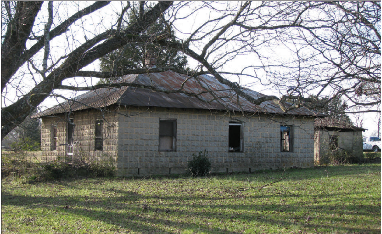
A. East Oblique, View to Northwest
