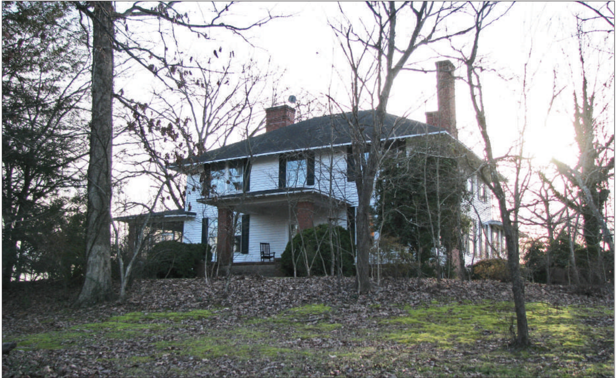
A. East Oblique, View to Northwest
