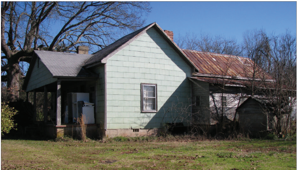
B. West Side, View to Southeast
