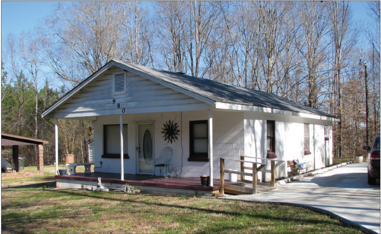
A. South Oblique, View to Northeast
