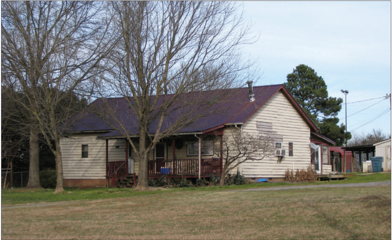
A. Façade and South Side, View to Northeast
