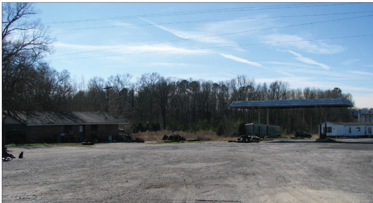
B. Gas Station and Canopy, View to Southwest
