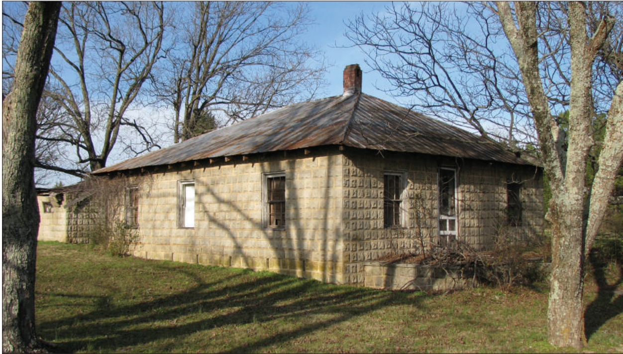
B. West Oblique, View to Northeast
