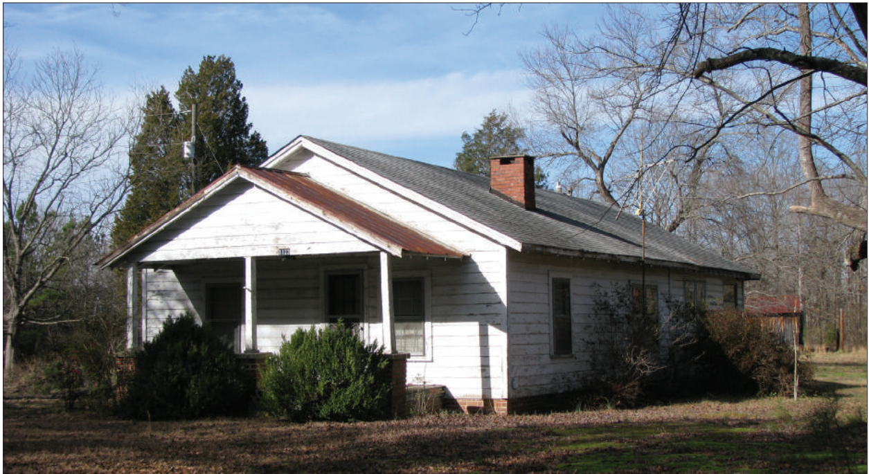
B. East Oblique, View to Northwest
