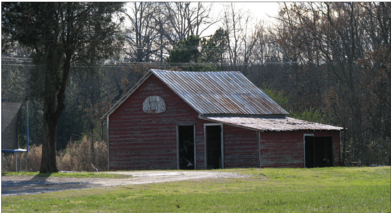
B. U/21/0254.03, View to Southwest
