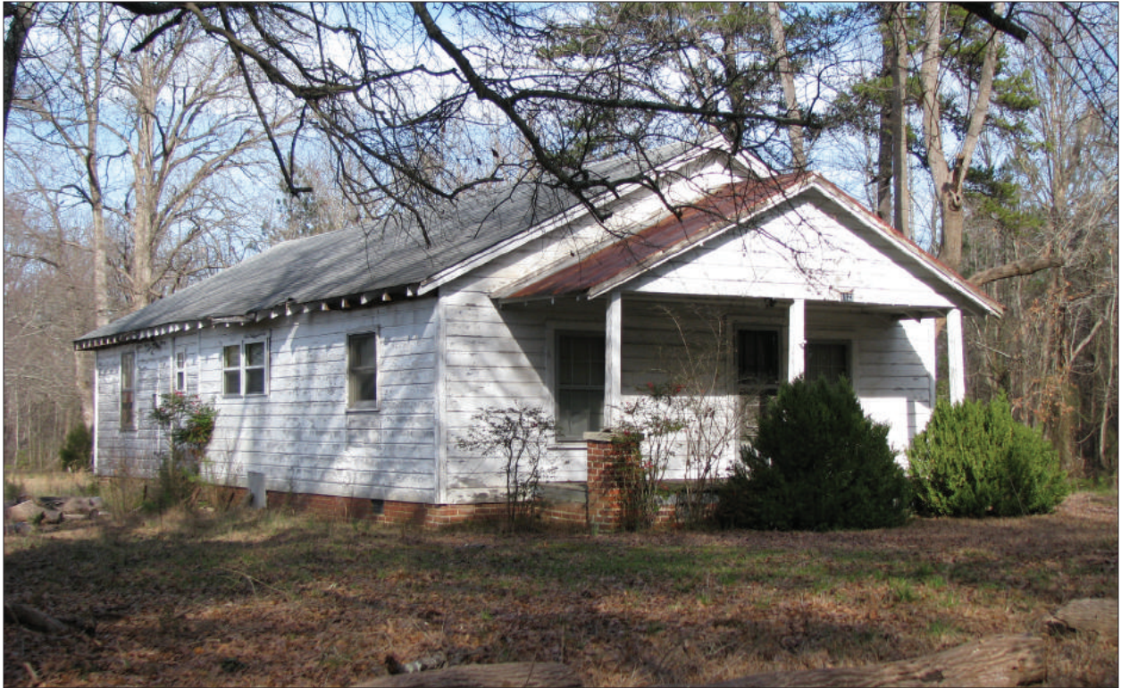
A. West Oblique, View to Northeast
