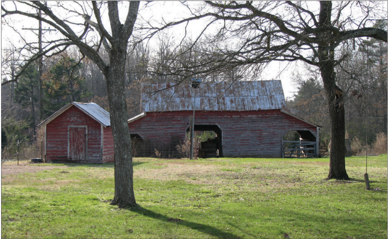
A. U/21/0254.01 and U/21/0254.02, View to West
