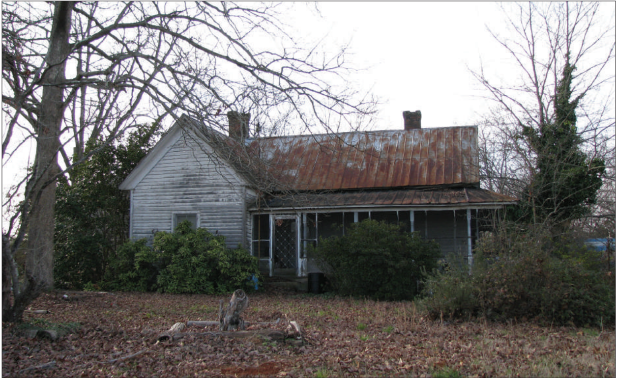
A. Façade, View to West
