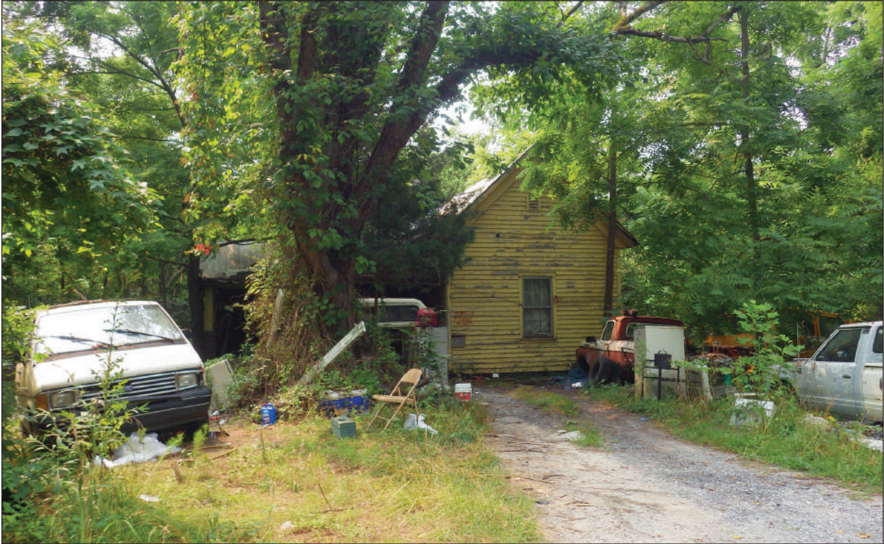
A. Façade, View to Southeast
