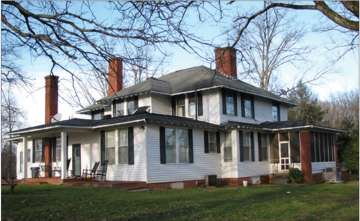
A. South Oblique, View to Northeast
