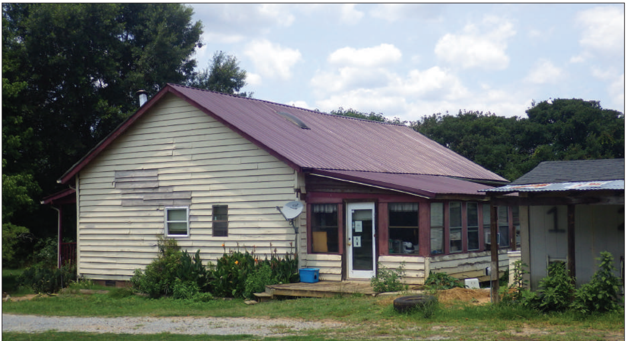
B. Rear (East) and South Side, View to North/Northwest
