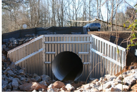
Use Pipe Wingwall
