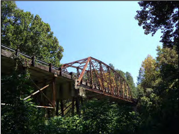
Existing S-68/S-227 Bridge
