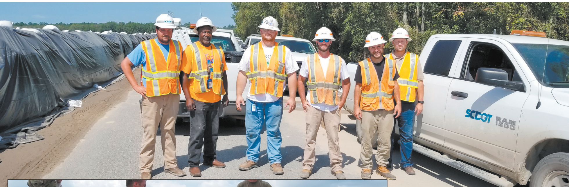
SEPT. 22: SCDOT crew members on the U.S. 501 Bypass flood barrier wall project included, from left: Danny Lane, Drew Drayton, Derrick Tindale, Corey Johnson, Philip Bethea and Travis Patrick.
