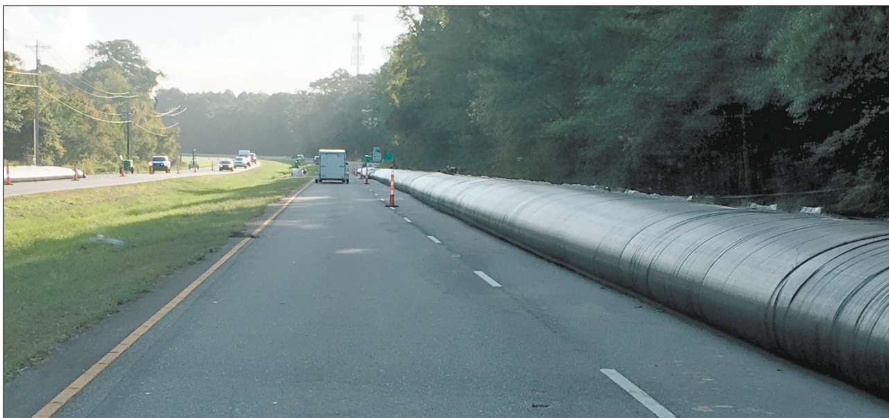
In Georgetown, SCDOT used AquaDams to keep U.S. 17 and U.S. 521 open. The AquaDams are large water-filled tubes that serve as dams to keep rising waters off the roadway.
