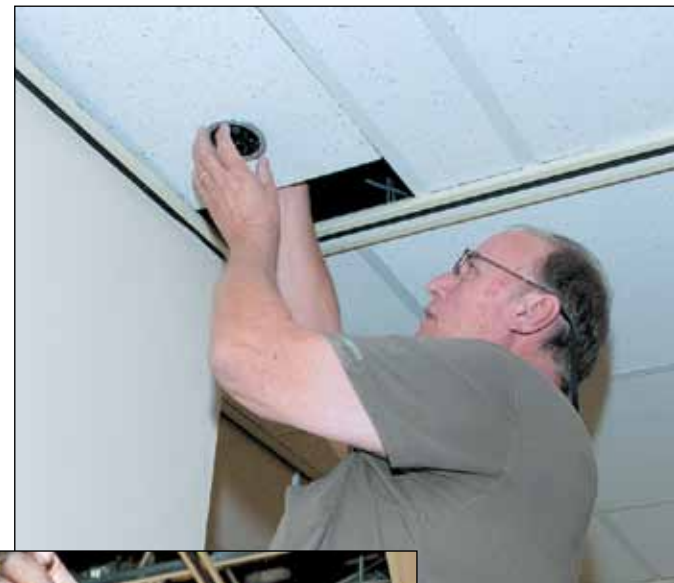
ABOVE: David Hamm runs wiring for cameras and audio visual equipment.
